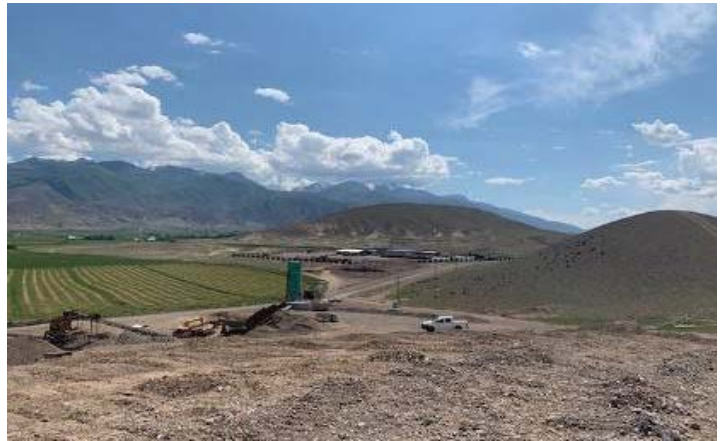
Lot 2 crusher section in front and Contractor's camp in background.
