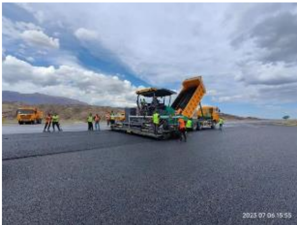
Photo 11. Lot 1. SMA-20 paving at 31+000-31+120 LHS (car park). July
