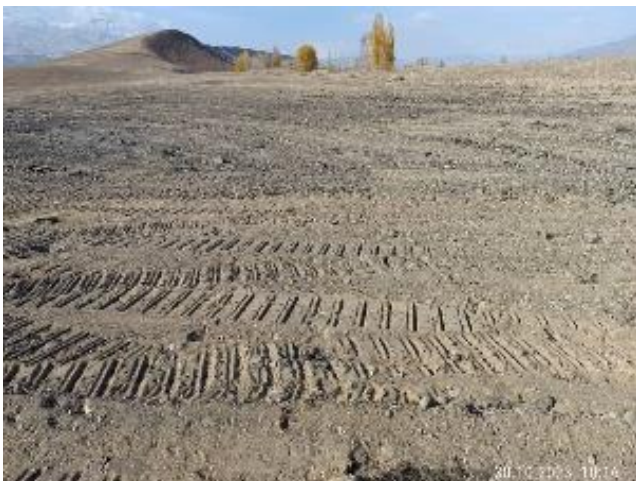
Photo 93. Old asphalt dump at km. 70+180 LHS after reclamation. October
