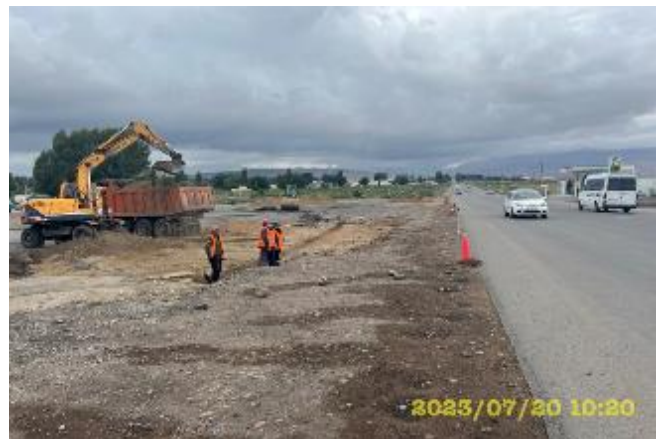
Photo 8. Lot 1. Exit's construction at km.2+680 LHS. July.
