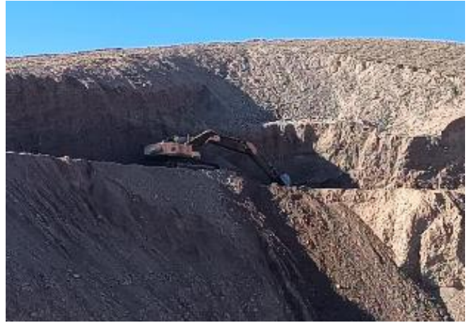
Photo 90. Quarry km. 75+400. Bringing the sides to a stable position
