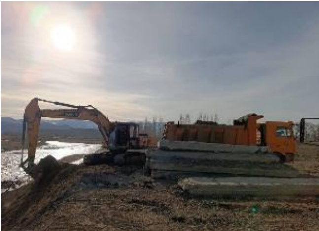
Photo 97. Temporary bridge of the bypass road dismantling at km 62+500
