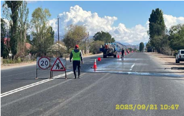
Photo 21. Chekildek village. Road marking. September
