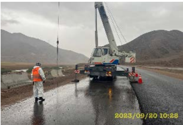
Photo 17: Parapets installation at km.42+000-43+000 September
