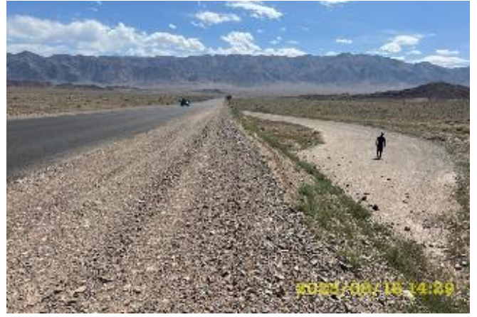
Photo 80. Bypass road km.21+430 RHS
