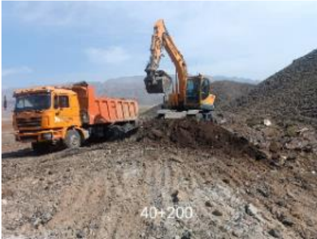
Photo 73. Levelling of the old asphalt spoil dump km. 40+200. September
