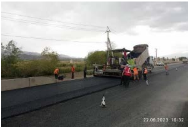
Photo 37. SMA pavement on km 67+945-68+915 RHS. August.
