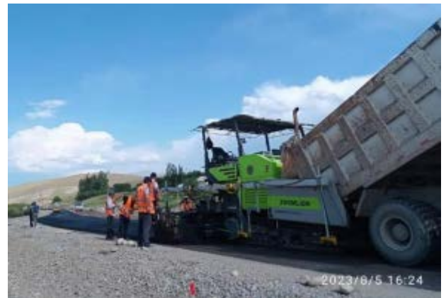
Photo 38. Sub-base pavement at km 85+900-86+500 RHS. August.
