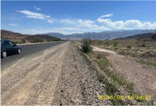
Photo 79. Bypass road km.18+300 RHS
