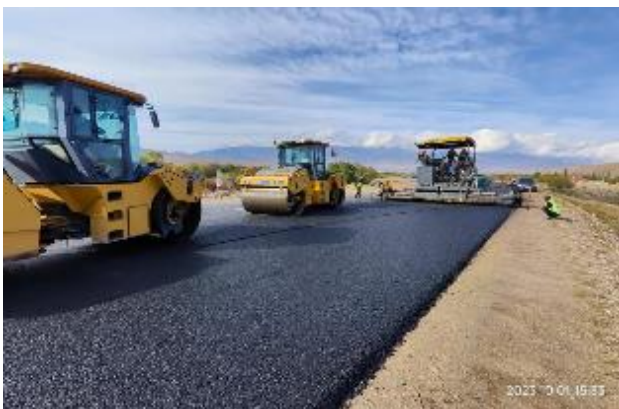
Photo 25. SMA paving on km 9+700-10+600 LHS. October.
