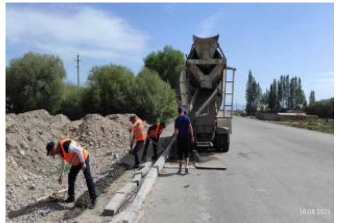
Photo 36. Sidewalk parapets installation at km 86+500-87+000 RHS. August.
