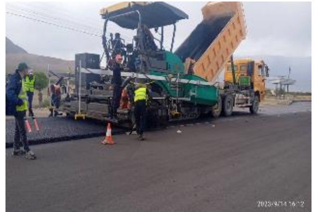
Photo 16. SMA pavement, Tash-Saray village. September.
