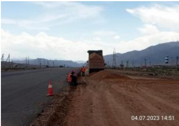
Photo 7. Lot 1: Sub-base backfilling of at the south coast exit 0+020-0+180 RHS. July
