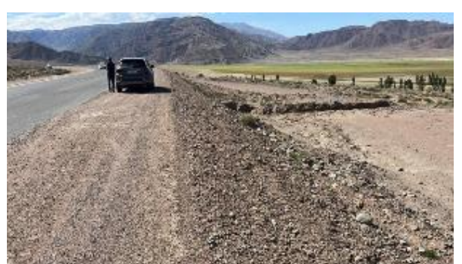
Photo 82. Bypass road km.37+700 RHS
