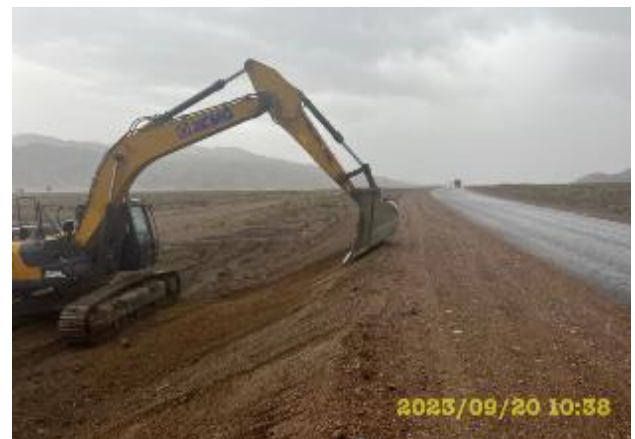
Photo 18. Slope cut at km.38+700. September.
