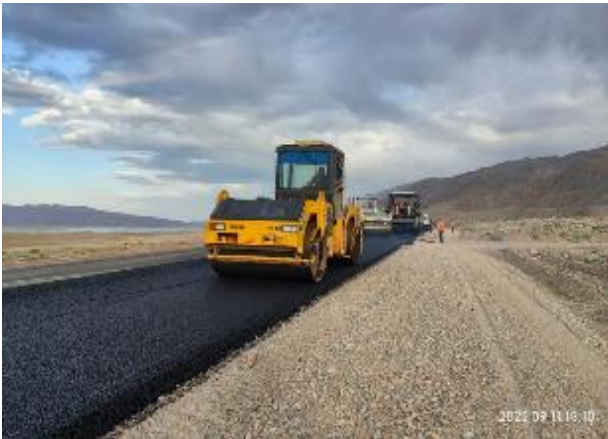
Photo 15. SMA pavement on km 39+424-40+545 LHS. September.
