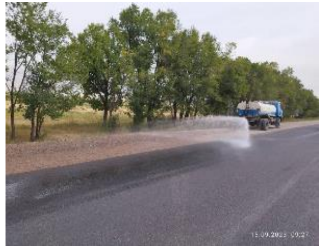
Photo 74. Watering of the road km 66+200. September
