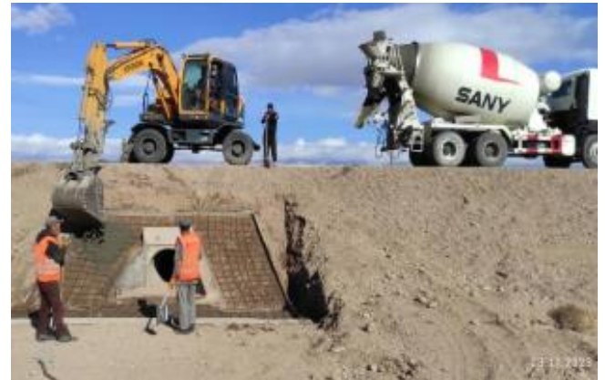
Photo 44. culvert inlet slopes reinforcement at km 71+800 LHS. November.
