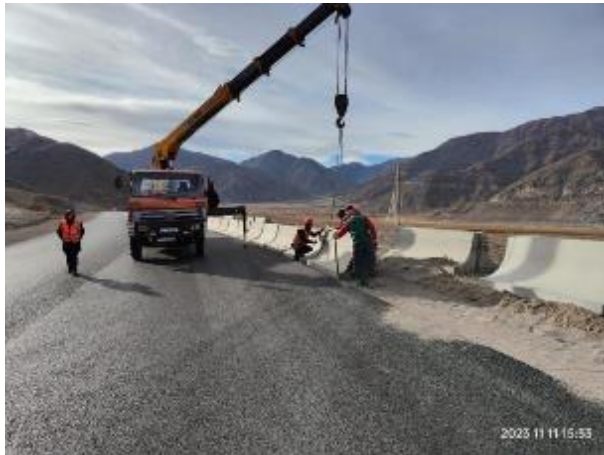
Photo 29. Parapets installation at km 40+700-40+870 RHS. November
