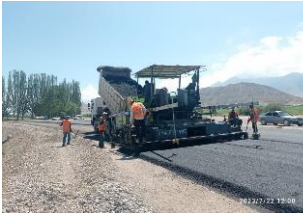
Photo 35. Sub-base pavement (roundabout). July.
