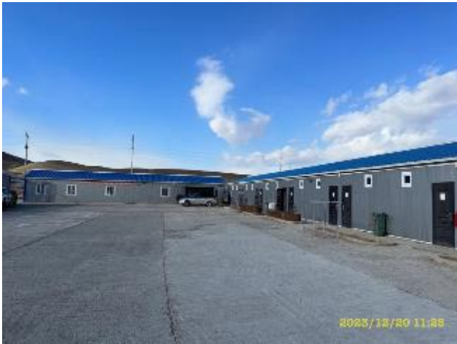
Photo 55. Contractor's accommodation camp
