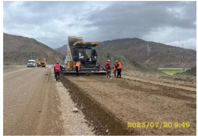
Photo 10. Lot 1. Earth works on km. 42+000-43+000. July
