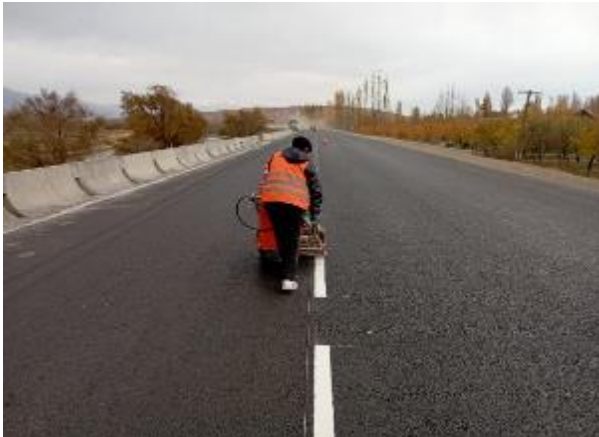
Photo 23. Tash-Saray village. Road marking. October
