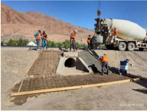
Photo 13: Culvert concrete reinforcement of inlet and outlet at 13+763 km. August
