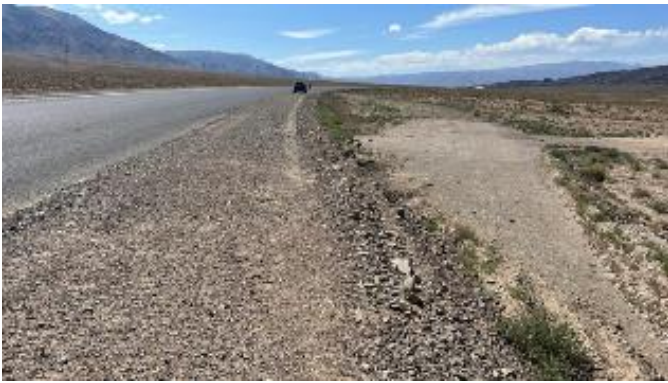
Photo 81. Bypass road km.24+430 RHS
