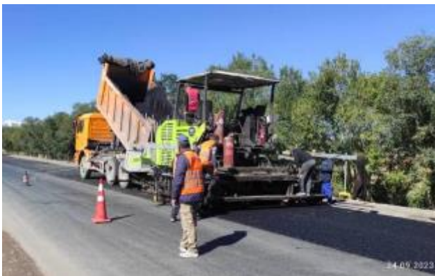
Photo 39. SMA pavement at km 85+500-87+000 RHS. September
