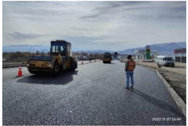
Photo 28. SMA pavement at km 0+600+0+840 RHS. November
