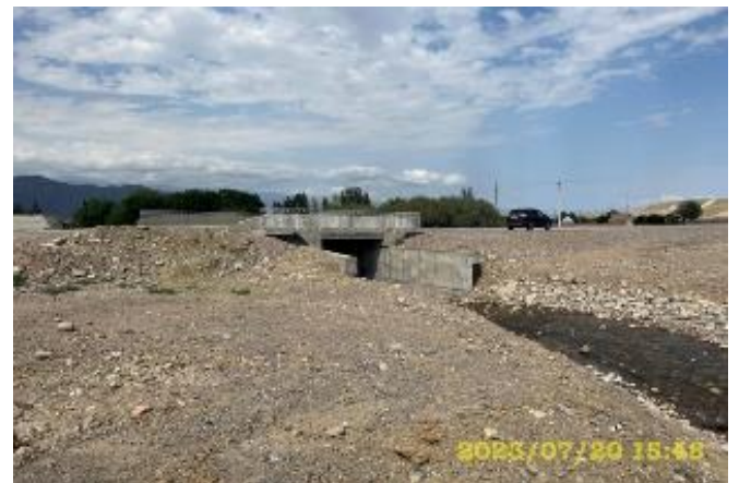
Photo 112. Bypass road of the bridge at km 86+261. r. Sazdyn-Suusuu, after reclamation
