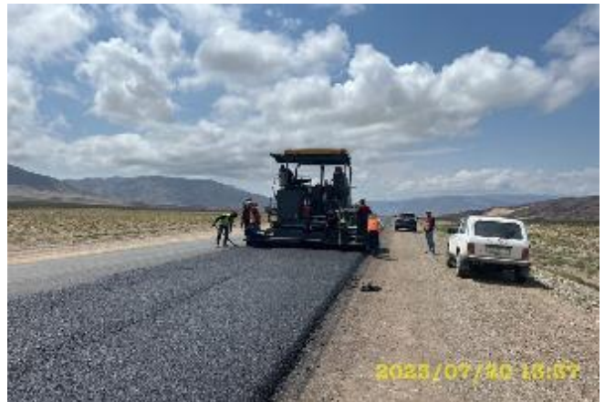
Photo 10. SMA paving at chainage 27-824--25+005 RHS. July
