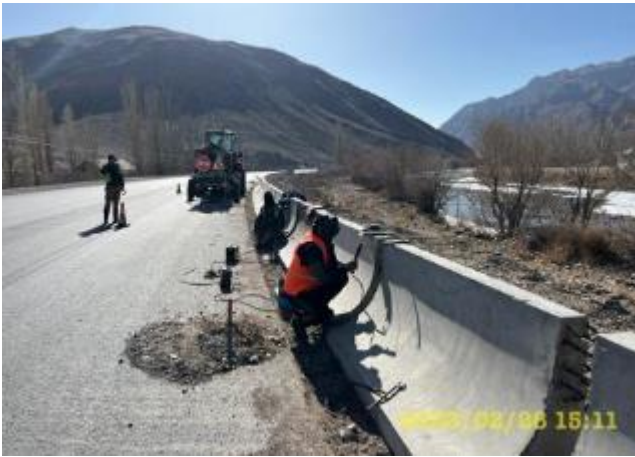
Photo 9. Lot 1. Assembling installed parapets from km 14+000-15+000. February
