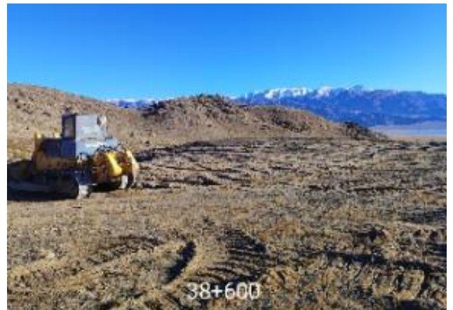
Photo 72. Levelling of the old asphalt spoil dump km. 38+600. September
