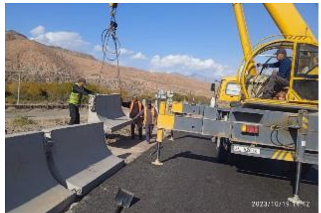
Photo 24. Parapets installation at km 11+200. October.
