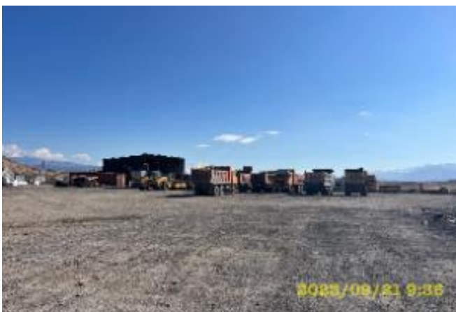
Photo 87. September. Sanitary condition of the construction equipment parking area is satisfactory.
