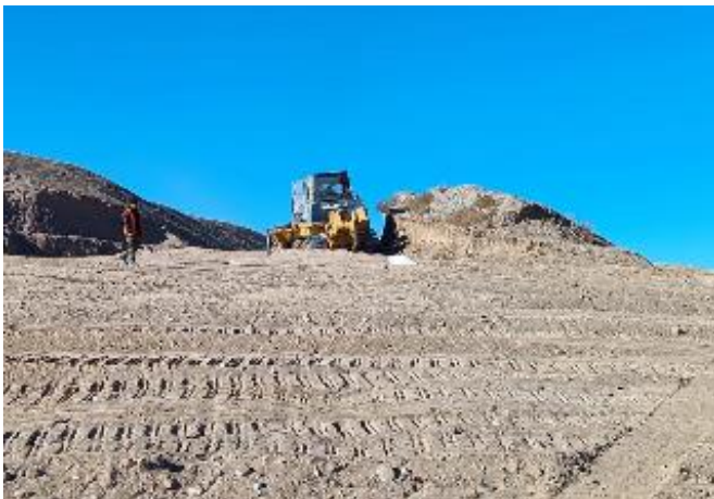
Photo 91. Quarry levelling at km. 75+400
