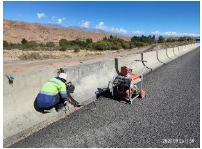
Photo 14. Parapets' reinforcements welding at km 13+240-13+480 RHS. September.
