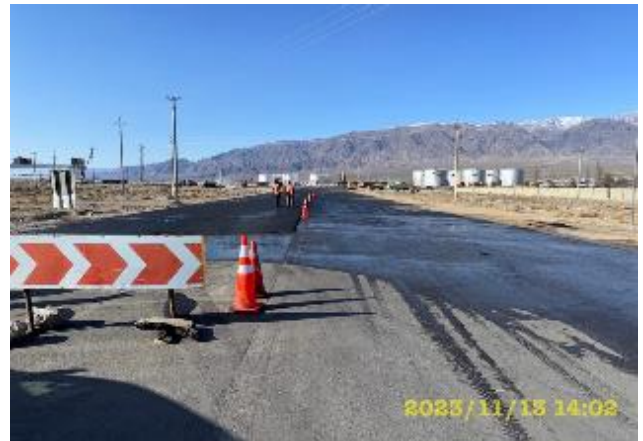
Photo 30. Asphalt paving preparation for on km 2+680 LHS exit. November
