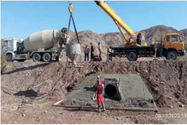
Photo 27. Culvert's inlet&outlet concrete reinforcement at km 18+326BS. October.
