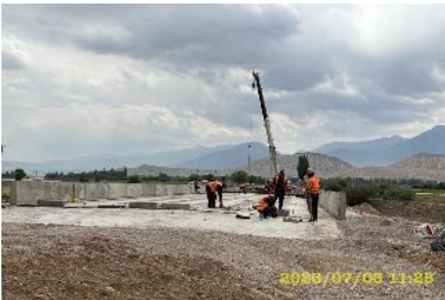
Photo 33. Bridge installation at km 65+410. July
