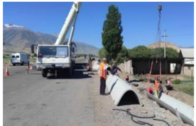
Photo 34. Installation of chutes at km 87-459-87+650 RHS. July
