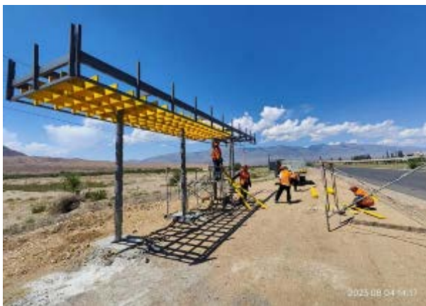
Photo 11. Lot 1. Stop shelter's construction at 9+070 km RHS. August
