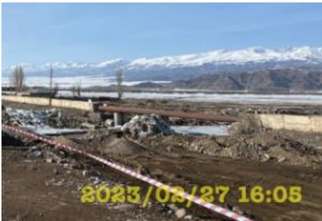
Photo 99. Spoil dump at km. 65+520 RHS before reclamation
