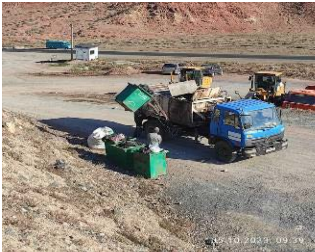
Photo 129. Lot 1. Removal of solid waste from Contractor's camp. October
