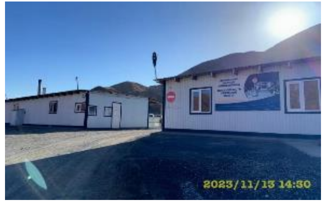
Photo 46. Lot 1. Accommodation camp and Subcontractor's office
