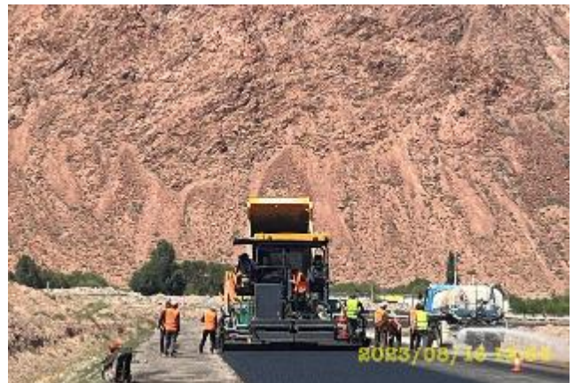
Photo 12. SMA paving at km 15+100 LHS. August.
