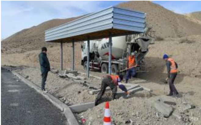
Photo 43. Parapets installation at bus stop on km 89+161. November.
