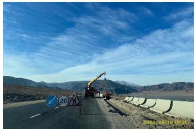
Photo 32. Parapets installation on km. 32+000-34+000. December
