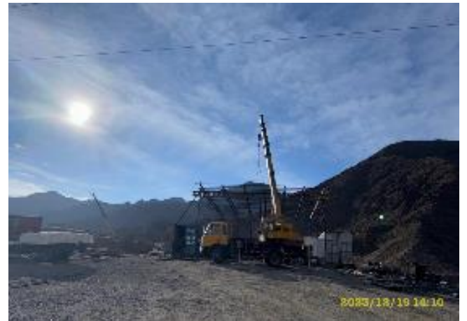
Photo 70. Production base. repair and mechanical block's dismantling
