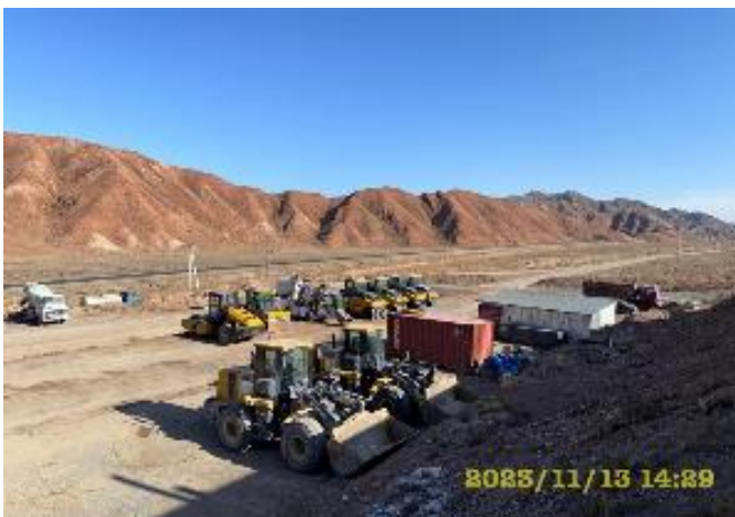
Photo 61. Sanitary condition of the construction equipment parking area is satisfactory. November.
