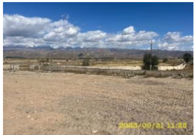
Photo 100. Spoil dump at km. 65+520 RHS after reclamation
