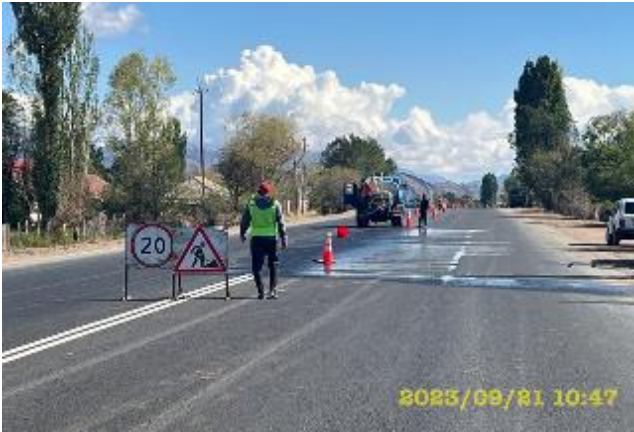
Photo 41. Chekildek village. Road marking. September.
