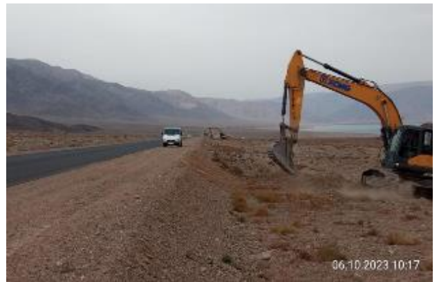
Photo 26. Slopes levelling at km 29+900-30+300 RHS. October
