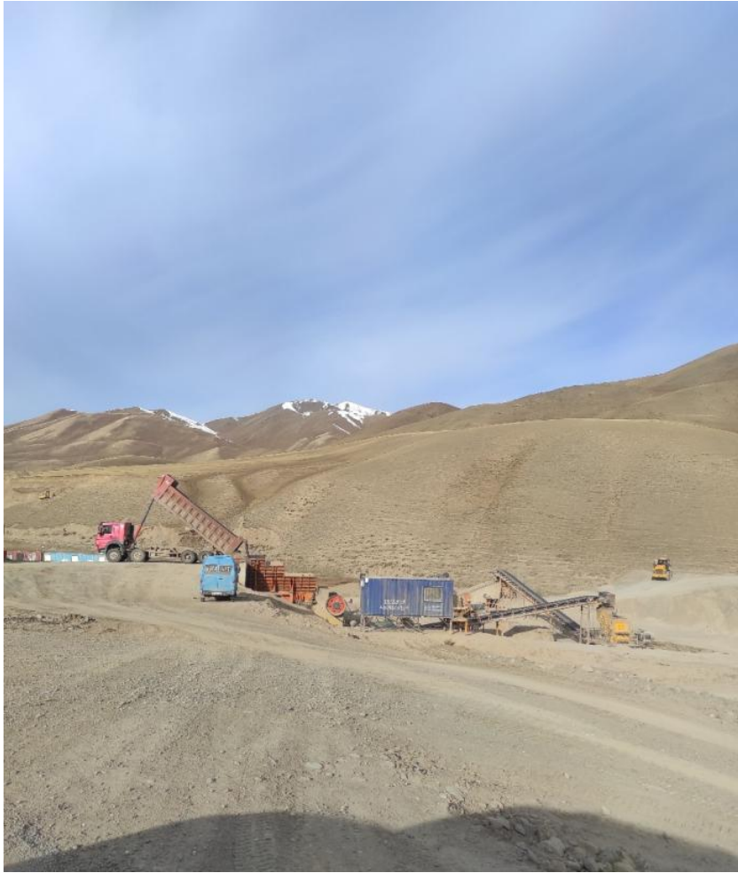
Figure 11: The production site (km 106+300)
