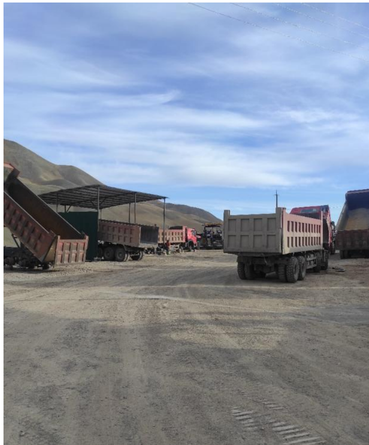
Figure 13: The area of the additional construction camp (km 106+300)
