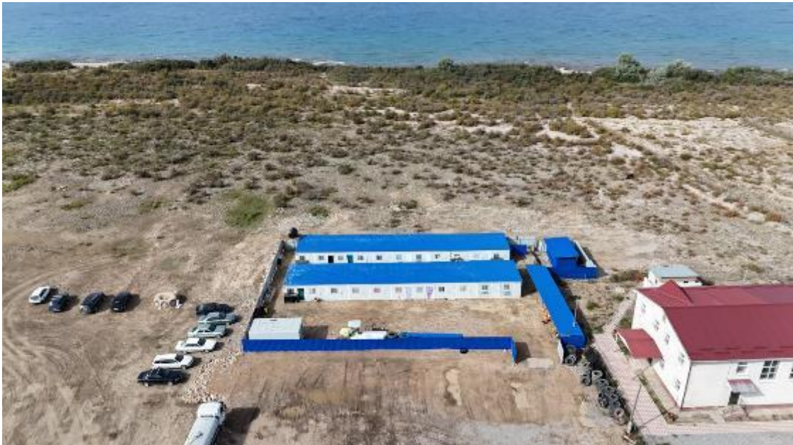
Figure 21: Aerial view of the Kichi-Jargylchak Camp area, km 150+610 LHS (Lot 1).
