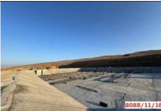
Photo 15. Production site, km 167+360 RHS, construction of a bitumen storage pit.
