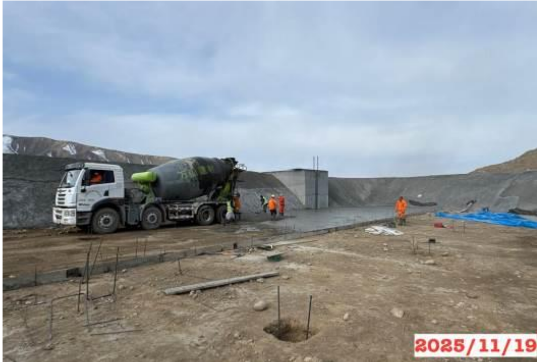
Figure 19: Production site, km 202+220 RHS, construction of a bitumen storage pit.
