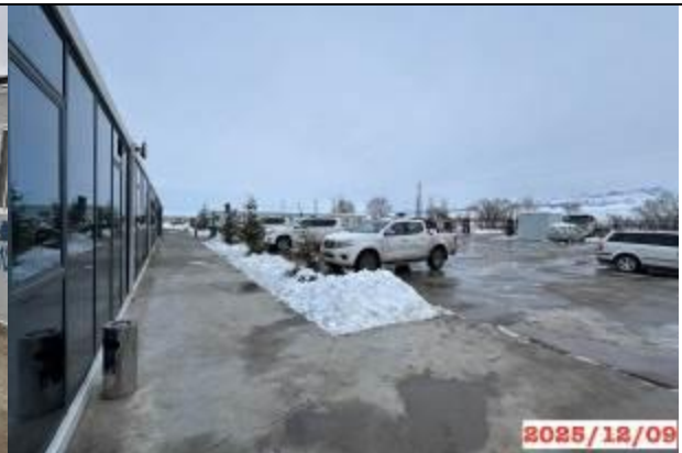
Photo 36. The Chyrak Camp, km 199+460 LHS. Contractor's office. The camp area is in satisfactory sanitary condition.
