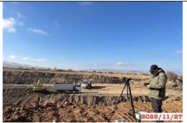
Photo 24. Noise and vibration measurements during quarry development at km 193+760, Lot 2.
