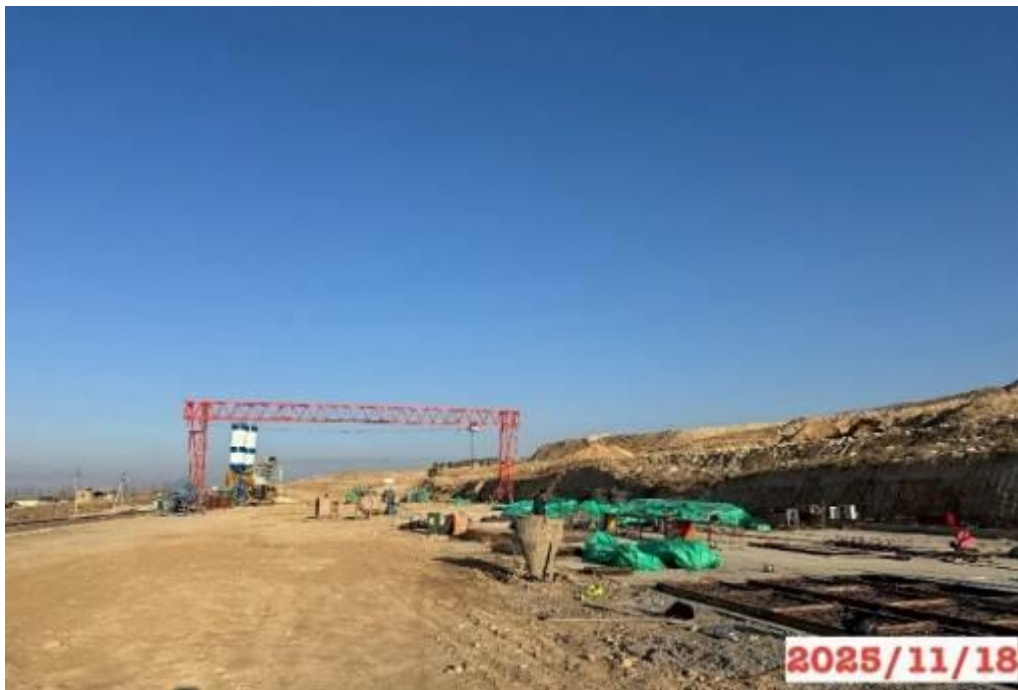
Figure 14: Production site, km 167+360 RHS. RCP section.
