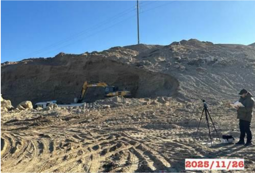
Figure 37: Noise and vibration measurements during quarry development at km 142+580, Lot 1
