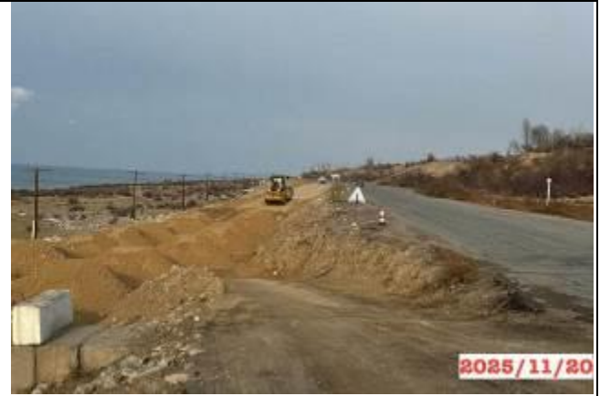
Photo 2. Earthworks for construction an embankment on the section at km 155+500
