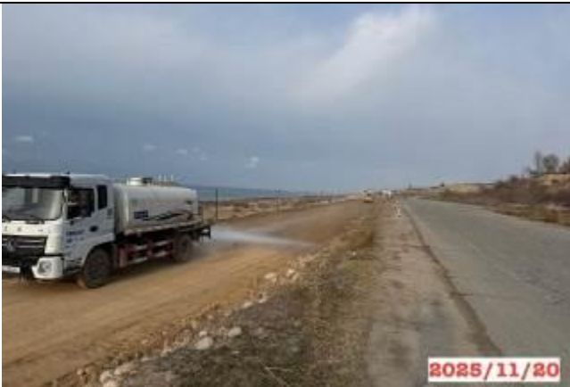
Photo 29. Dust suppression of construction sites at km. 155-km.156 LHS
