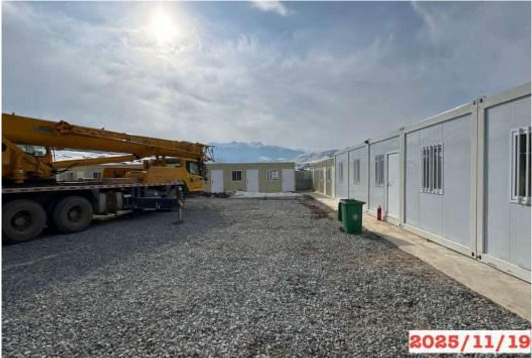
Figure 32: The Chyrak Camp area, km 202+220 RHS (Lot 2).
