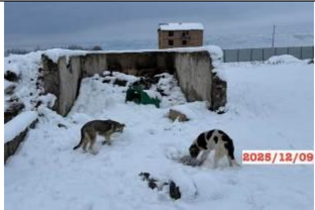
Photo 40. The Chyrak Camp, km 199+460 LHS. The storage conditions for solid waste do not comply with environmental and sanitary requirements.
