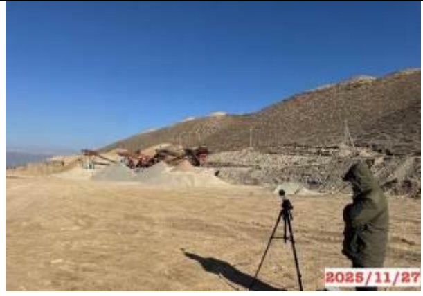
Photo 26. Noise and vibration measurements at the CSP production site, Lot 2, km 202+220
