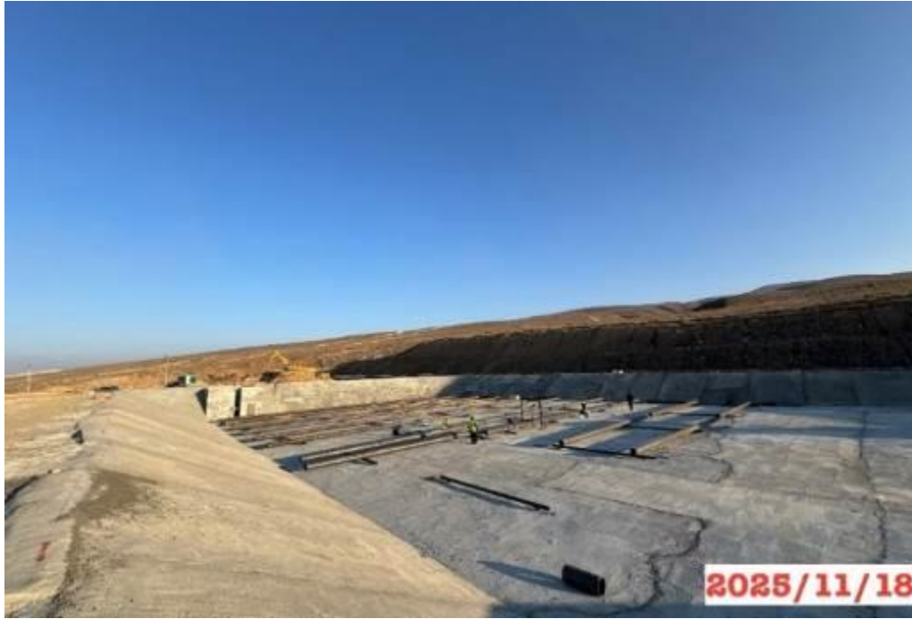
Figure 15: Production site, km 167+360 RHS, construction of a bitumen storage pit.
