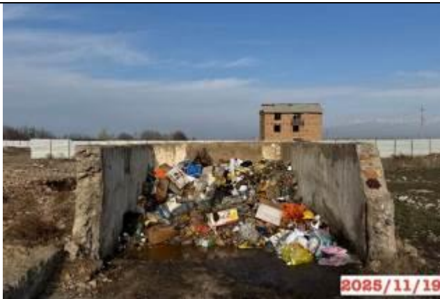
Photo 9. The Chyrak camp, km 199+460 LHS. The storage conditions for solid waste do not comply with environmental and sanitary requirements.
