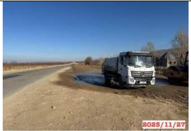
Photo 30. Dust suppression of construction sites at km 195 LHS
