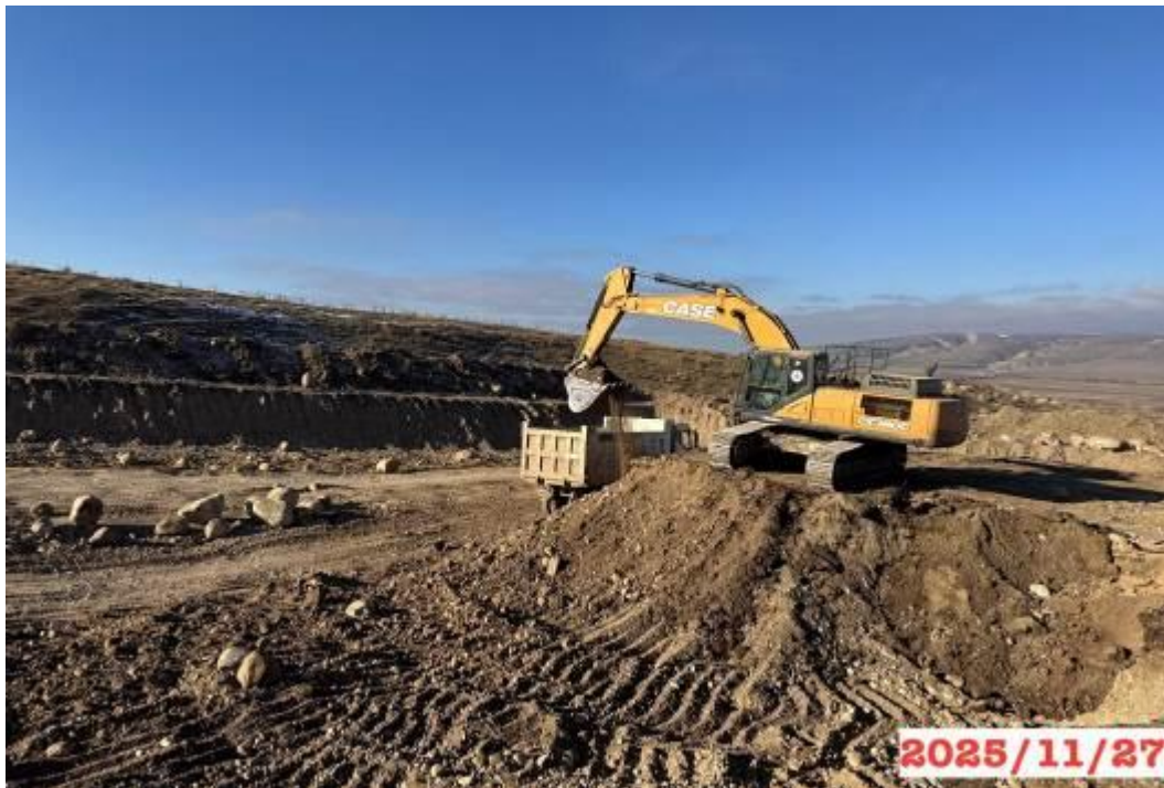
Figure 9: Quarry development km 191+384, RHS.
