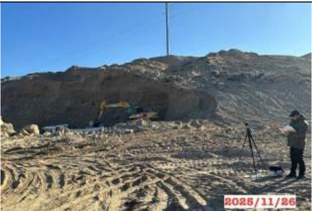
Photo 23. Noise and vibration measurements during quarry development at km 142+580, Lot 1.
