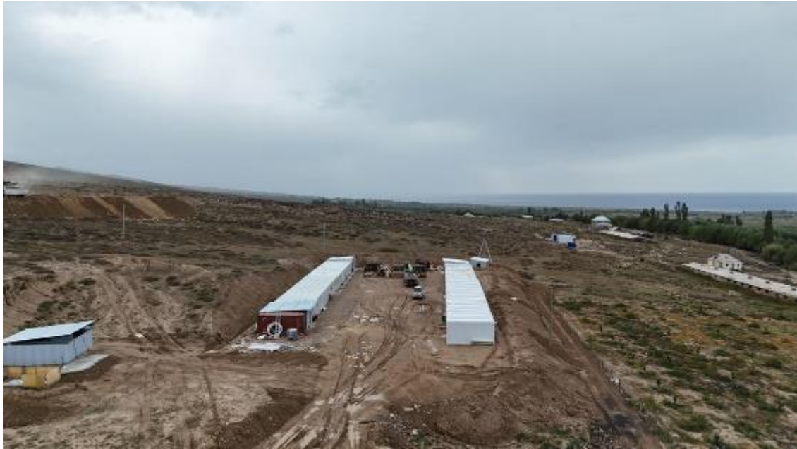
Figure 26: Aerial view of the Darkan camp area, km 167+360 RHS (Lot 1).
