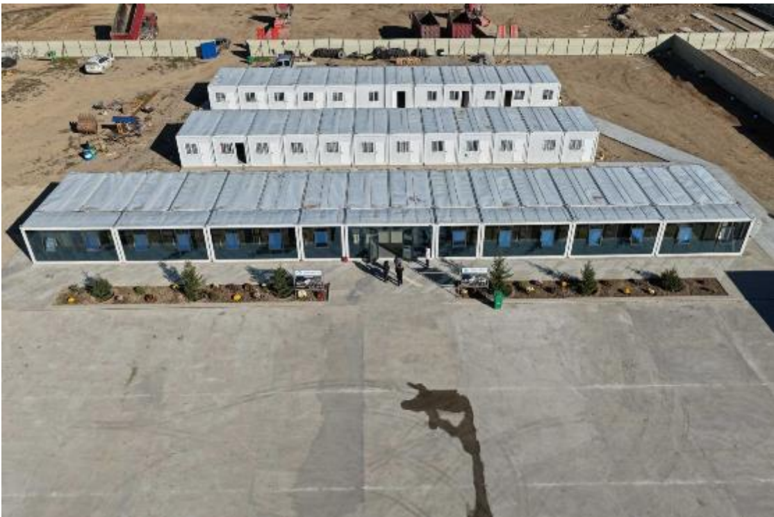
Figure 29: Aerial view of the Chyrak Camp office premises, km 199+460 LHS (Lot 2).
