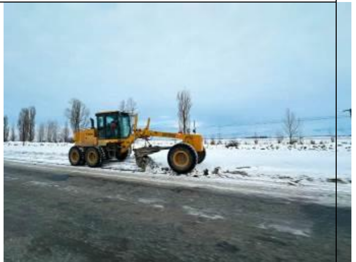
Photo 34. Lot 2. Clearing the road of snow, km 204
