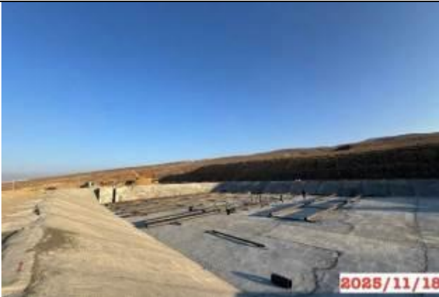
Photo 45. Production site, km 167+360 RHS, construction of a bitumen storage pit.
