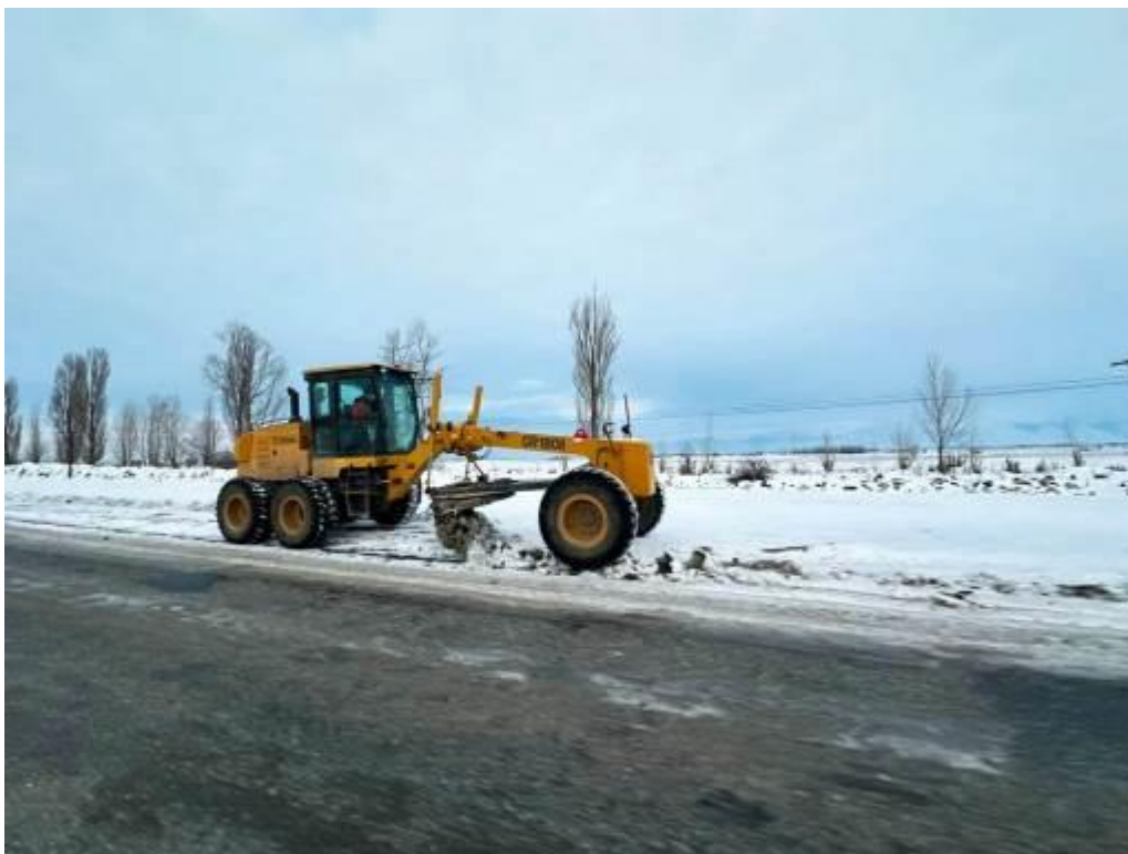
Figure 10: Winter maintenance of the road at km 204+000
