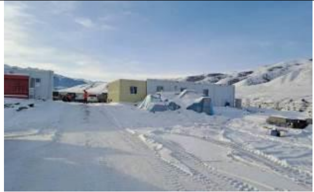
Photo 44. Production site, km 202+220 RHS, the camp territory is in satisfactory sanitary condition.
