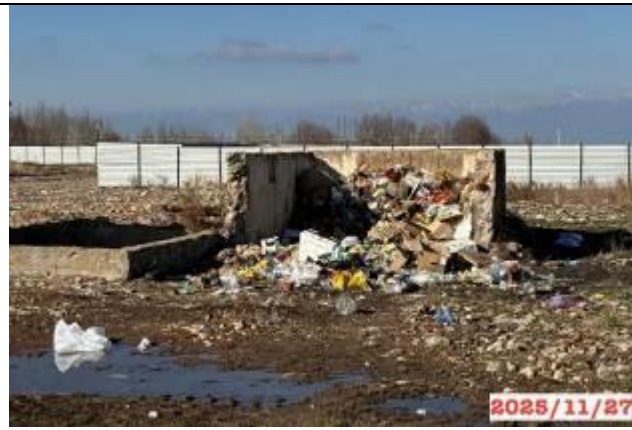
Photo 10. The Chyrak camp, km 199+460 LHS. The storage conditions for solid waste do not comply with environmental and sanitary requirements.
