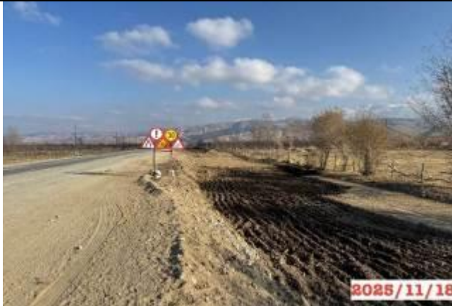
Photo 1. Earthworks for removal soil on the section at km 141-142.
