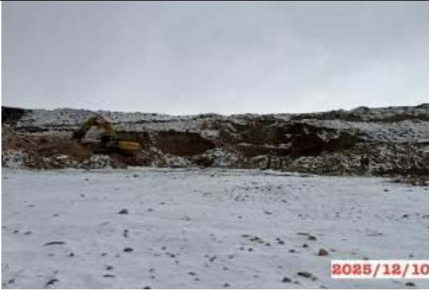
Photo 43. Quarry km 167+360 RHS. Not developed.
