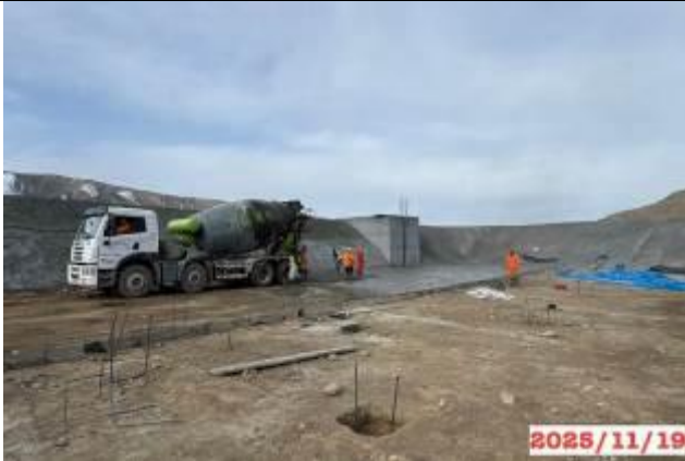
Photo 19. Production site, km 202+220 RHS, construction of a bitumen storage pit.
