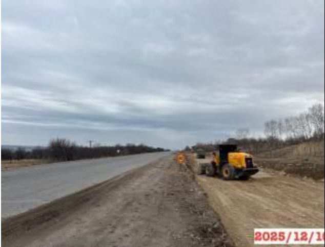
Photo 31. Lot 1. Earthworks for embankment construction
