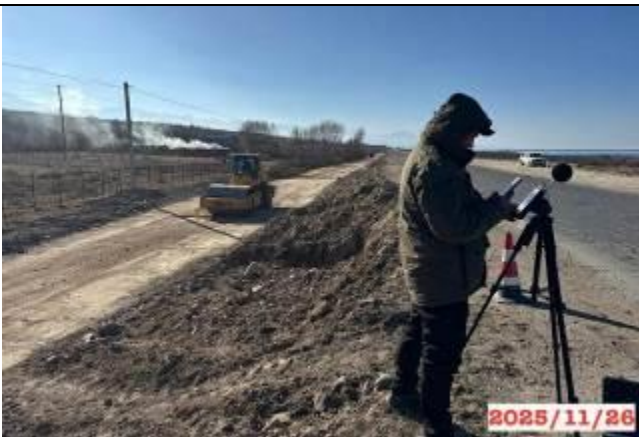
Photo 27. Noise and vibration measurements at the construction site, km 196, section 1
