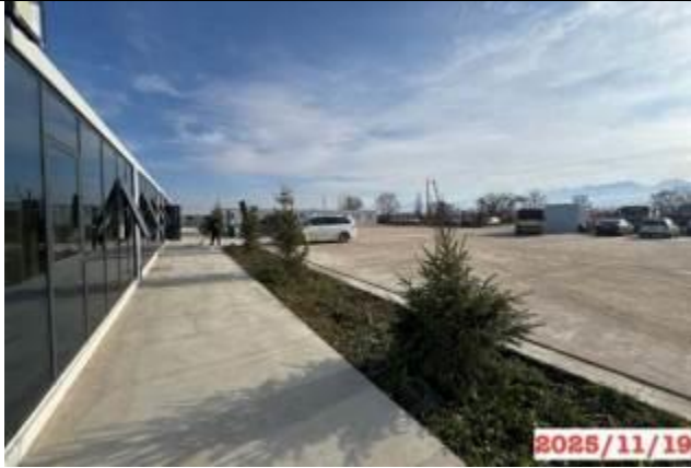
Photo 7. The Chyrak camp, km 199+460 LHS. Contractor's office. The camp area is in satisfactory sanitary condition.
