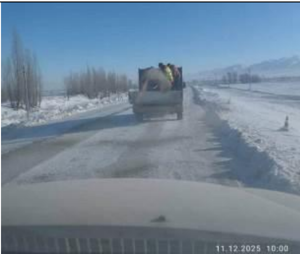
Photo 33. Lot 2. Road backfill along the entire section of Lot 2 from the village of Kyzyl-Suu to the town of Karakol
