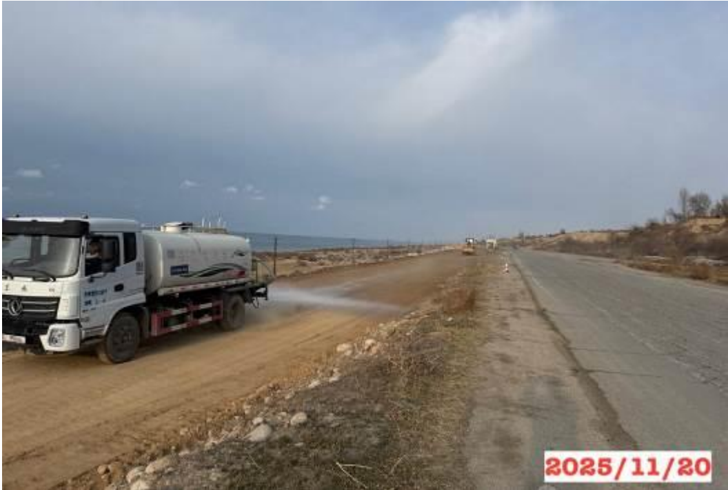
Figure 11: Dust suppression of construction sites at km 155+000 – km 156+000, LHS.
