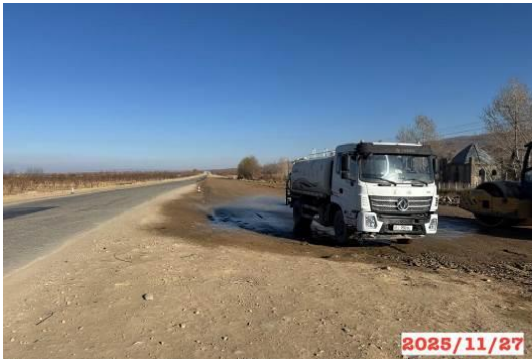
Figure 12: Dust suppression of construction sites at km 195+000, LHS.
