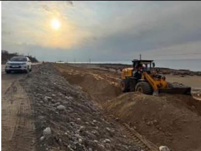
Photo 3. Earthworks for the construction of an embankment on the section km 154-156
