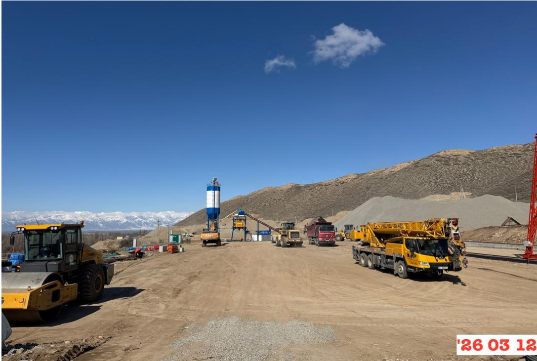
Figure 20: Production site, km 202+220 RHS.
