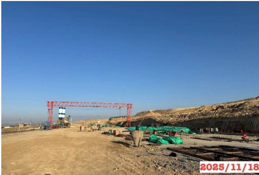
Figure 15: Production site, km 167+360 RHS. RCP section.
