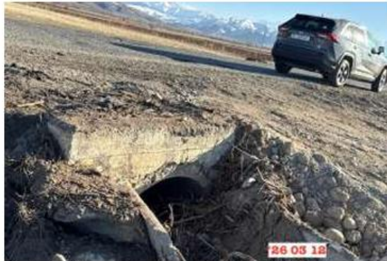
Photo 7. Water culvert pipe on km188+400 LHS, outlet
