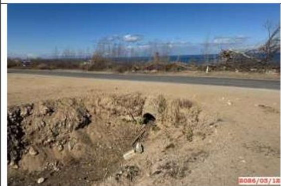
Photo 4. Debris flow passage on km151+260 RHS. inlet
