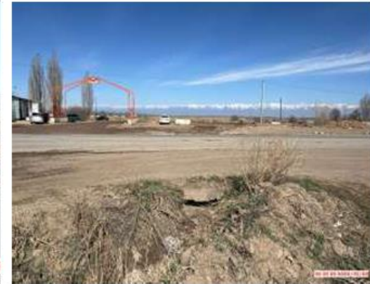
Photo 9. Water culvert pipe on km200+ RHS. inlet
