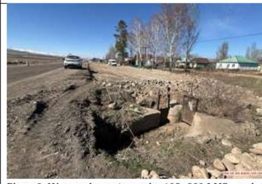
Photo 6. Water culvert pipe on km195+830 LHS, outlet.
