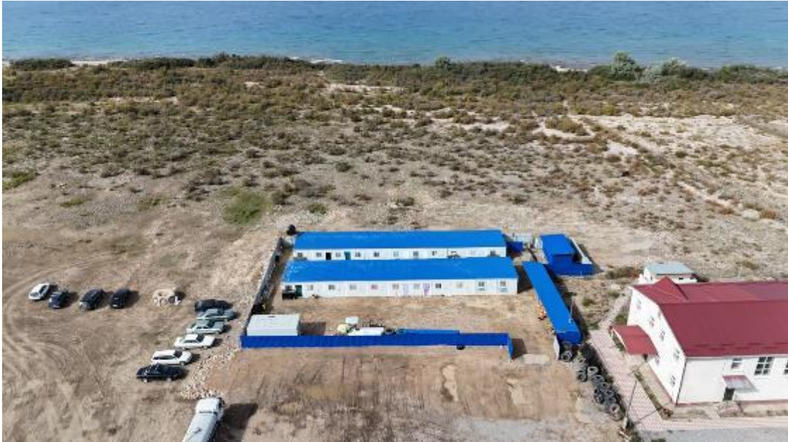
Figure 22: Aerial view of the Kichi-Jargylchak Camp area, km 150+610 LHS (Lot 1).
