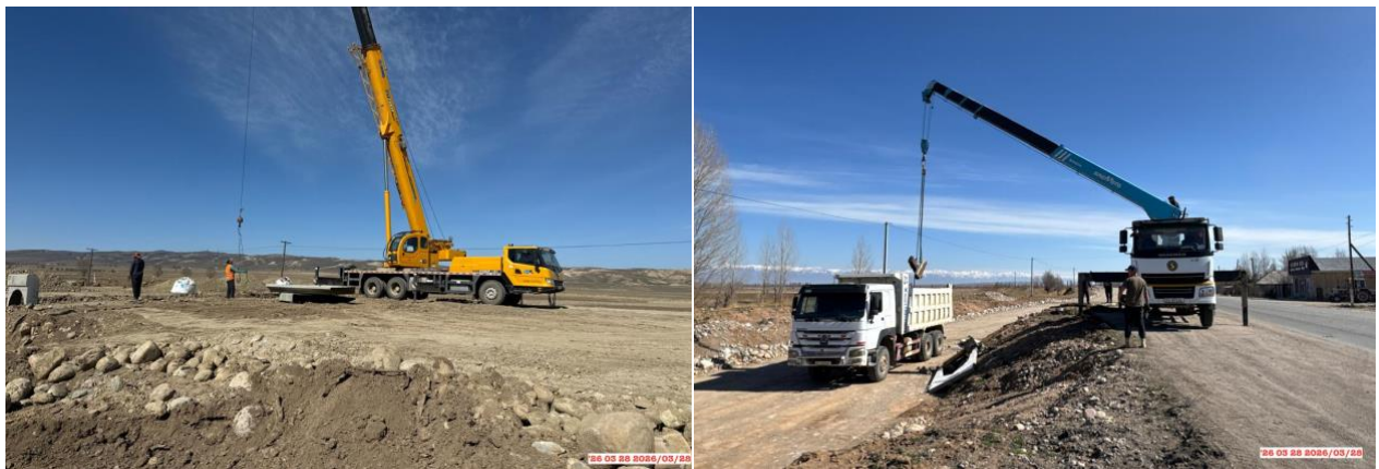
Figure 45: Removal of dismantled parts of the culvert at km 194
