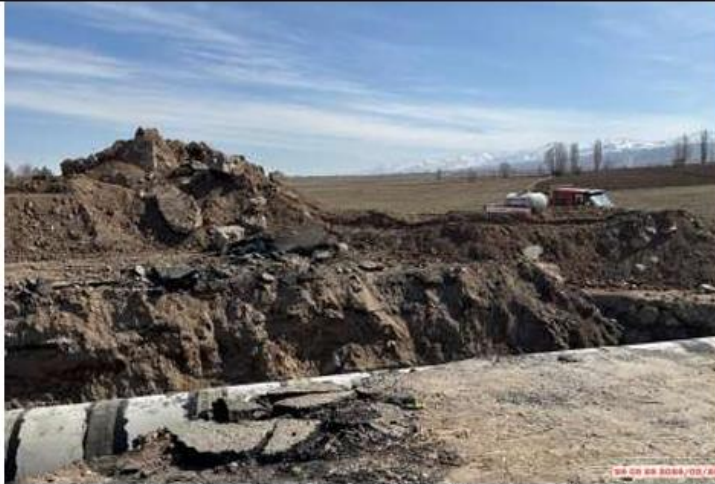
Photo 13. Wastes of shoveled asphalt on the construction sites.
