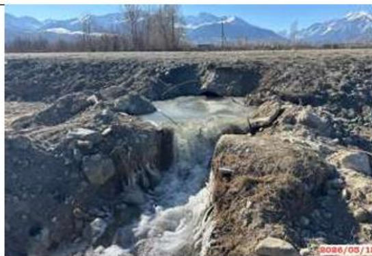
Photo 5. Water culvert pipe on km140+760, outlet
