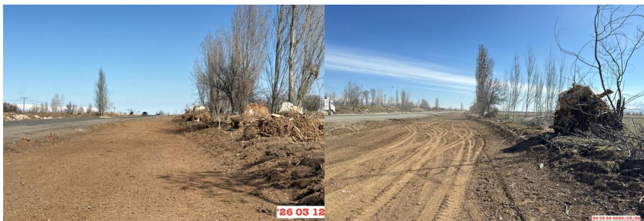
Figure 43: Large roots of felled trees left on the side of the road, km 202+700 and km 203+000
