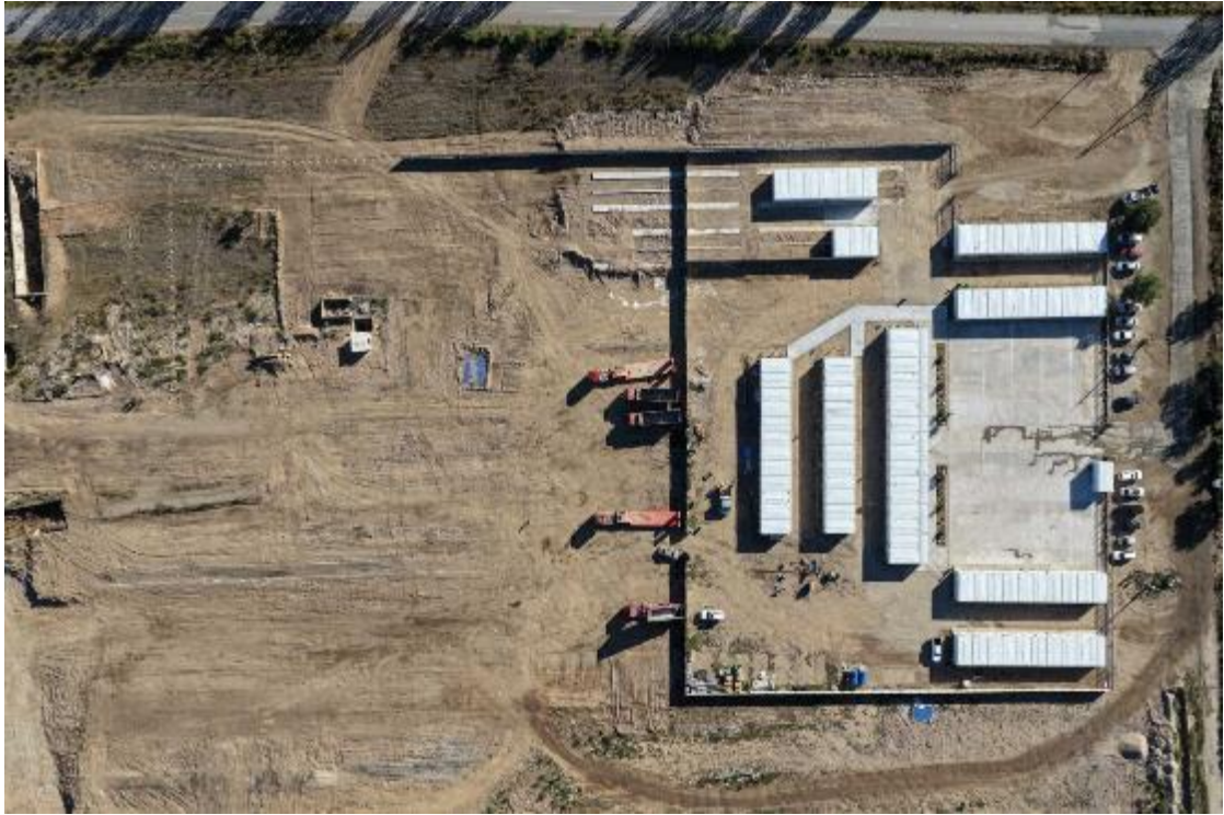
Figure 29: Aerial view of the Chyrak Camp area, km 199+460 LHS (Lot 2).
