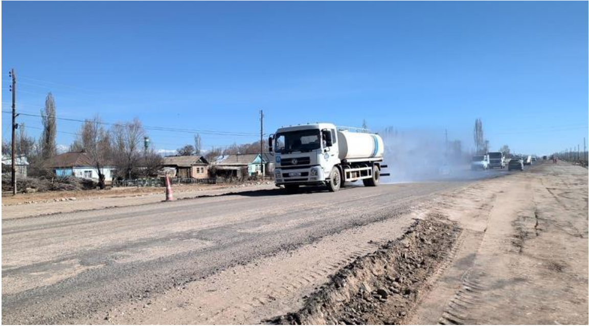
Figure 12: Dust suppression of construction sites at km 201+000.
