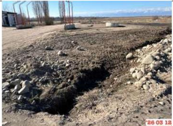
Photo 10. Water culvert pipe on km200+ RHS. Outlet
