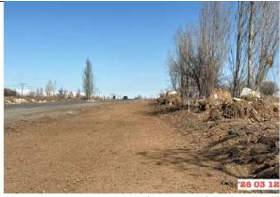
Photo 11. Km. 203. Big roots of cut trees, left on the edge of the road
