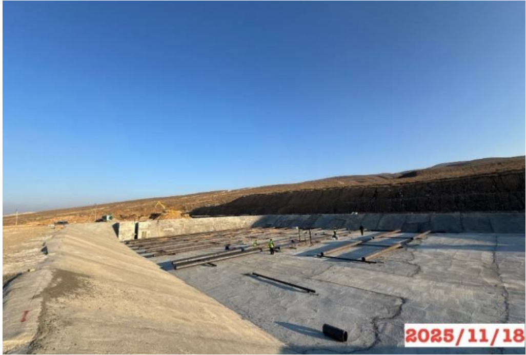
Figure 16: Production site, km 167+360 RHS, construction of a bitumen storage pit.
