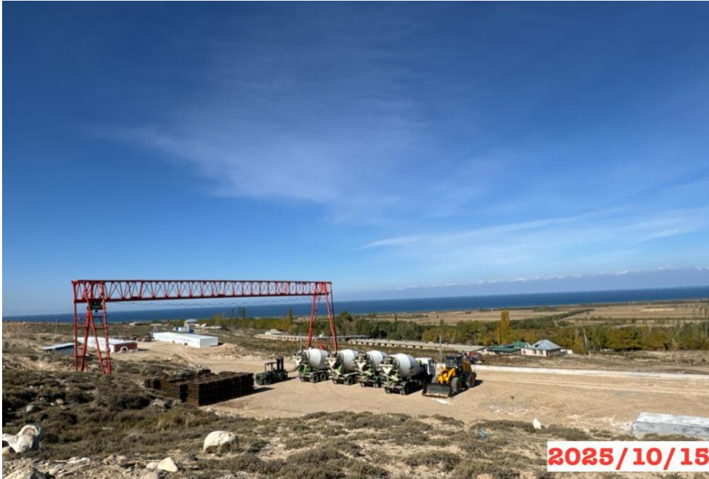
Figure 14: Production site, km 167+360 RHS
