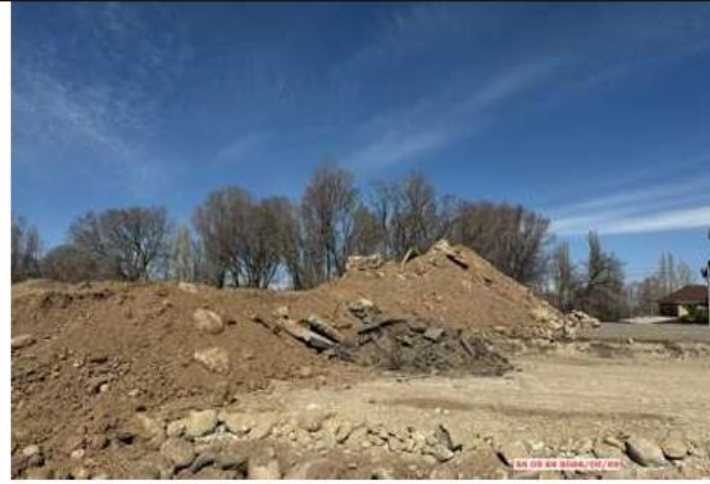
Photo 14. Storage of wastes of shoveled asphalt on the construction sites
