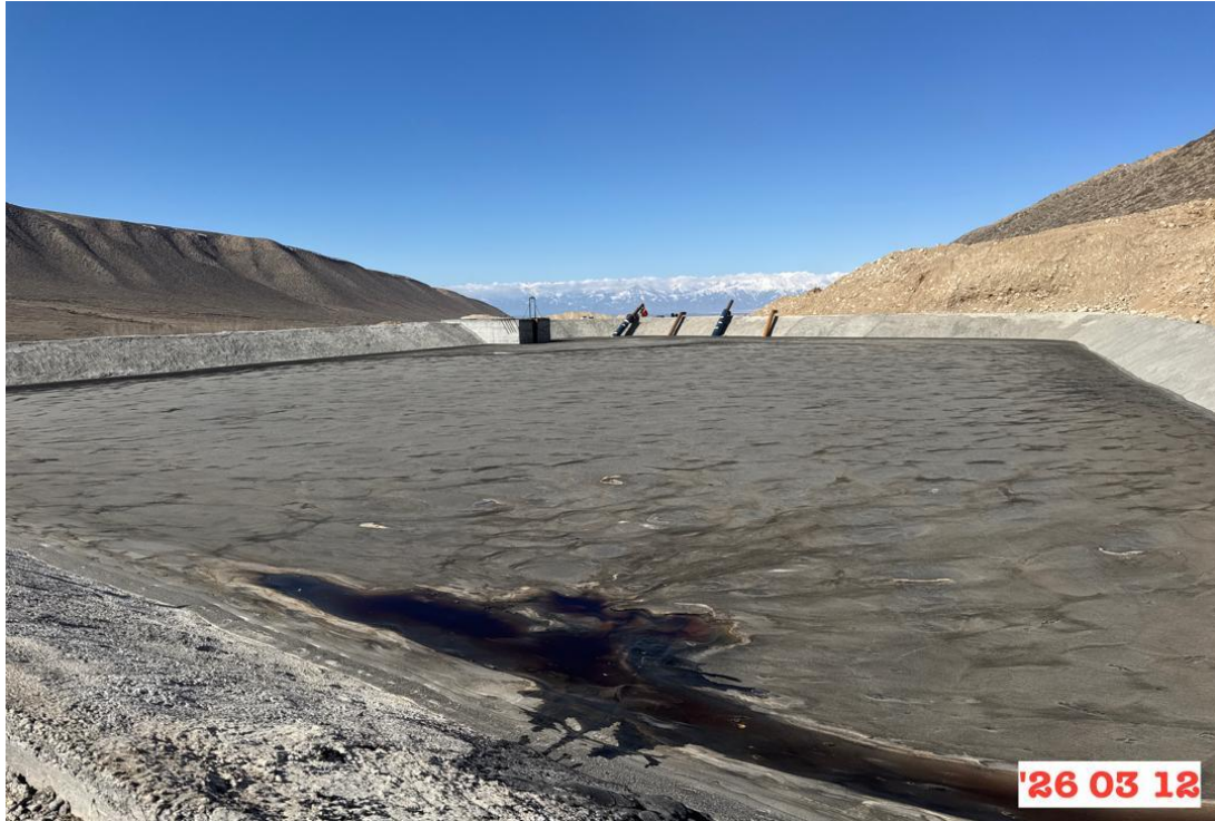
Figure 21: Production site, km 202+220 RHS, construction of a bitumen storage pit.
