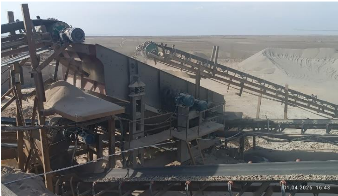
Figure 17: Operation of the CSP at the production site at km 167+360.
