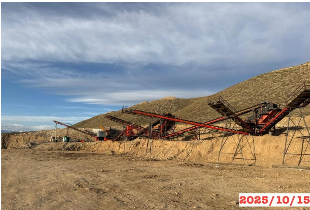
Figure 19: Production site 202+220 RHS, CSP
