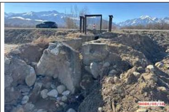
Photo 1. Water culvert pipe, on km .141+140 LHS. Outlet
