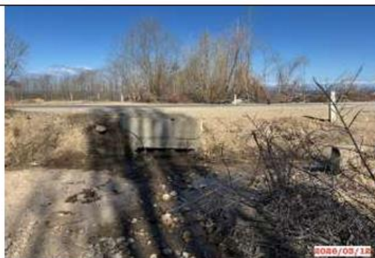
Photo 2. Debris flow passage on km.151+020 RHS. inlet
