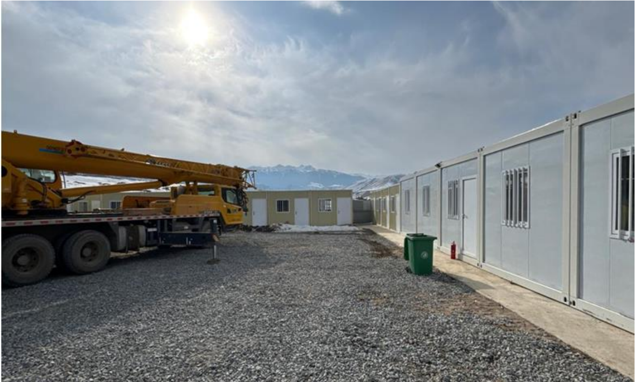
Figure 33: The Chyrak Camp area, km 202+220 RHS (Lot 2).
