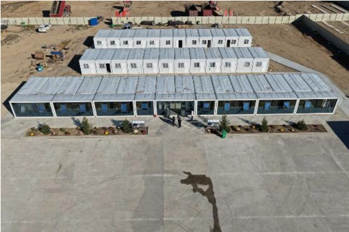
Figure 30: Aerial view of the Chyrak Camp office premises, km 199+460 LHS (Lot 2).
