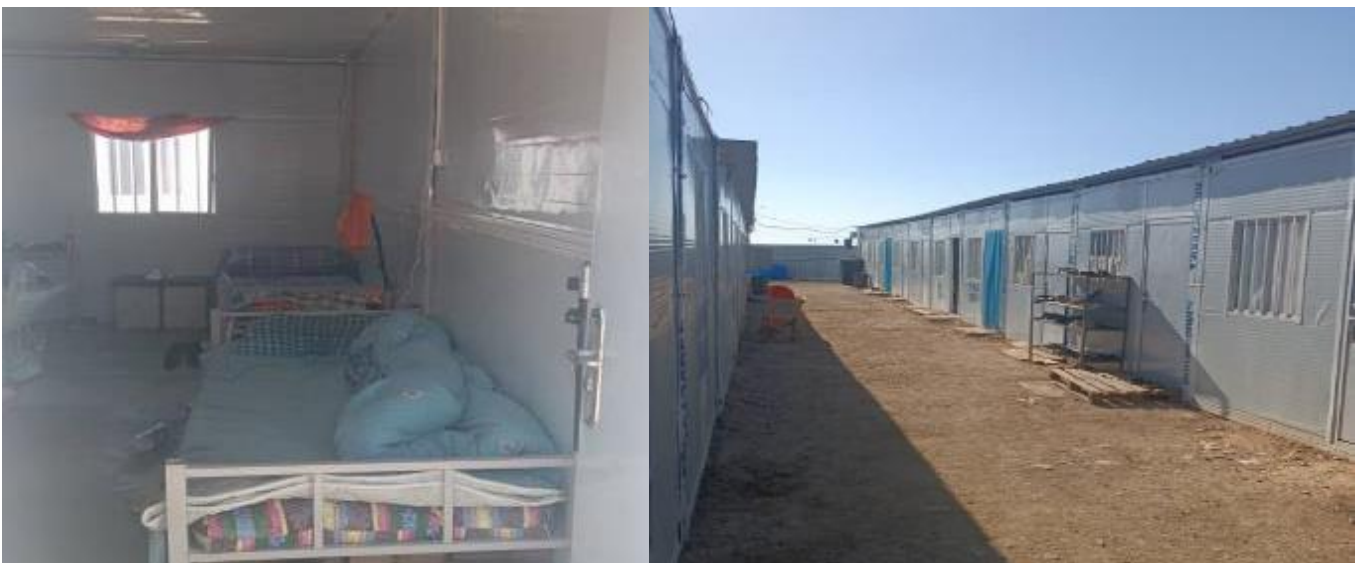
Figure 23: Dormitory for the Contractor's workers of the Kichi-Jargylchak camp, km 150+610 LHS (Lot 1).
