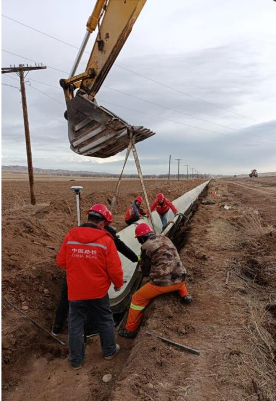
Figure 6: Installation of LR 6 trays at km 187, LHS.
