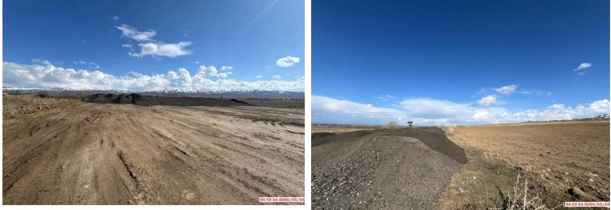
Figure 44: Storage of milled asphalt materials at construction sites km 194+600 and km 199+500
