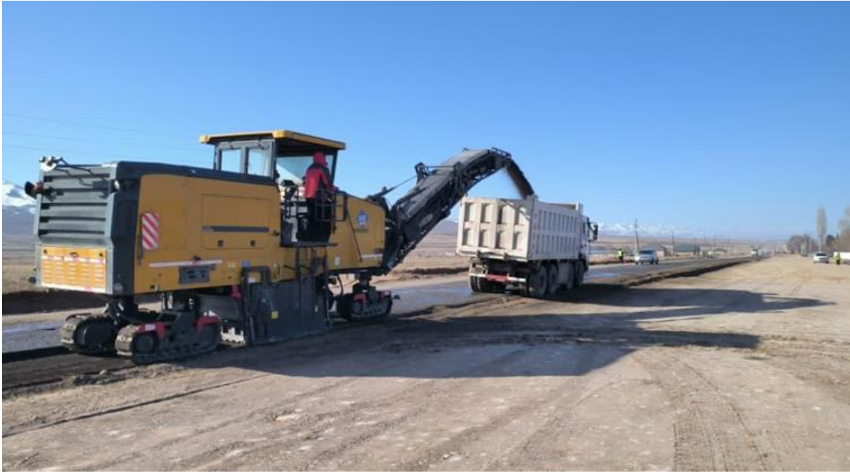
Figure 7: Milling of the existing asphalt concrete pavement at km 200.
