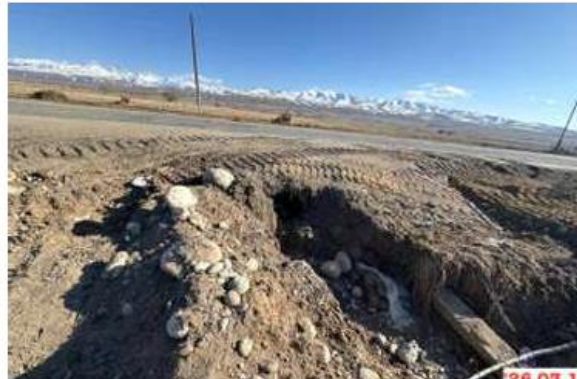
Photo 8. Water culvert pipe on km198 LHS, outlet
