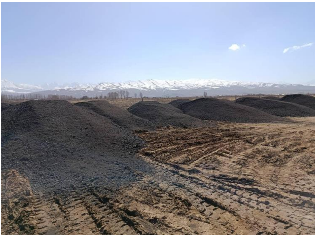
Figure 8: Stockpiling of existing asphalt concrete material after milling at km 195, RHS.
