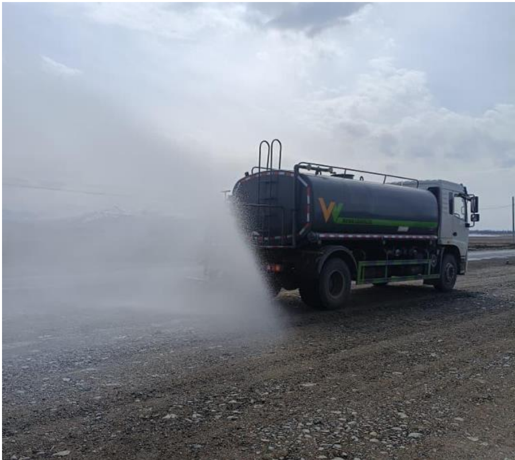
Figure 13: Dust suppression of construction sites at km 198+000.
