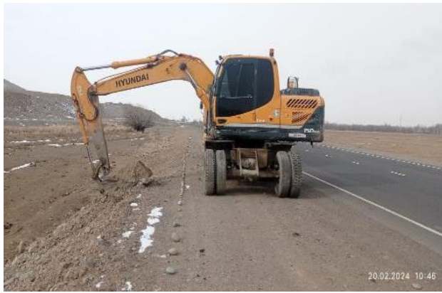
Photo 24. Slope cutting km. 80+600 LHS. February 2024.
