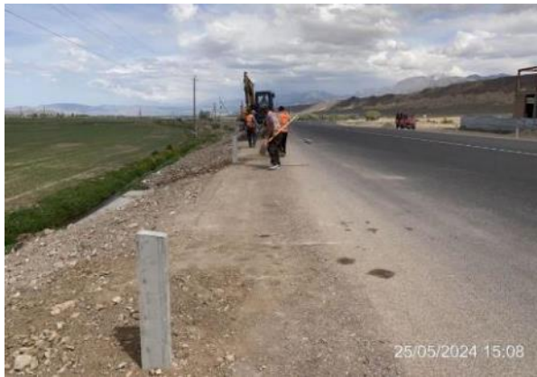
Photo 30. Installation of signal posts km 73+000-76+000 BS, May 2024.
