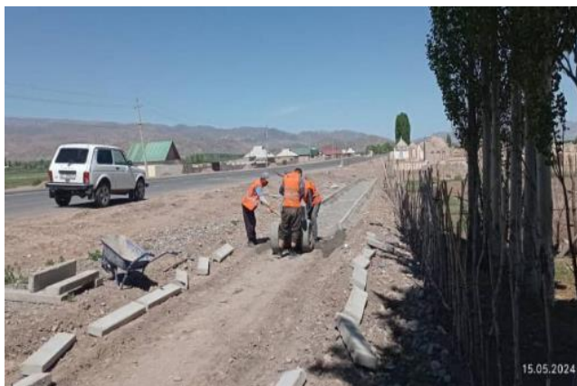
Photo 32. Installation of sidewalk curbs km 69+850-70+000 LHS. May 2024.
