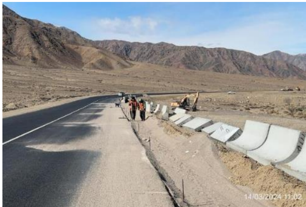
Photo 11. Construction and leveling of sand cushion 36+530-36+820 RHS. March 2024.
