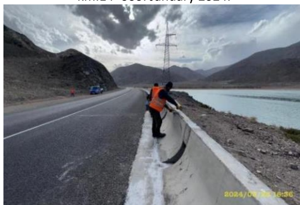
Photo 8. Lot 1. Installation of parapets at km 39+000 March 2024.
