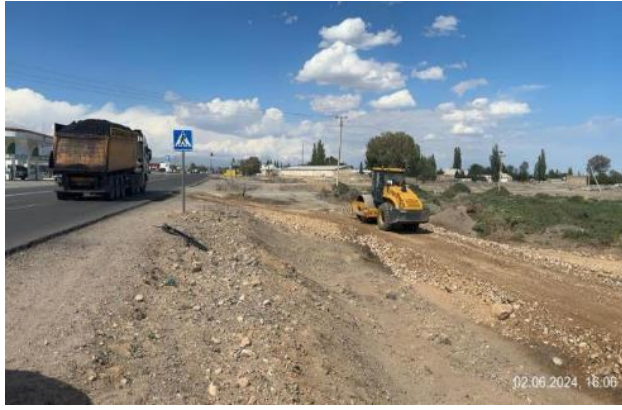
Photo 21. Preparation of sidewalk embankment km 0+600-0+750 LHS. June 2024.
