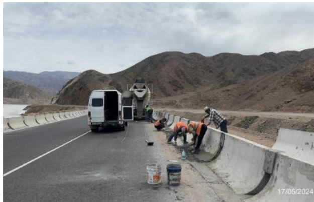
Photo 17 . Concreting of parapet joints at 41+920-42+095 LHS. May 2024.
