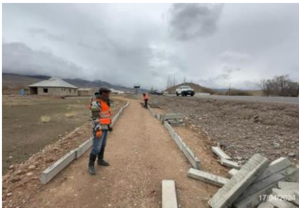
Photo 28. Installation of curbs for sidewalks, km. 86-87. April 2024.
