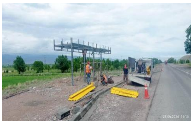
Photo 32. Installation of sidewalk curbs km 69+850-70+000 LHS. May 2024.
