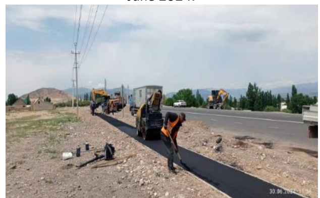
Photo 33. Construction of a sidewalk in Kok-Zhar v. June 2024.
