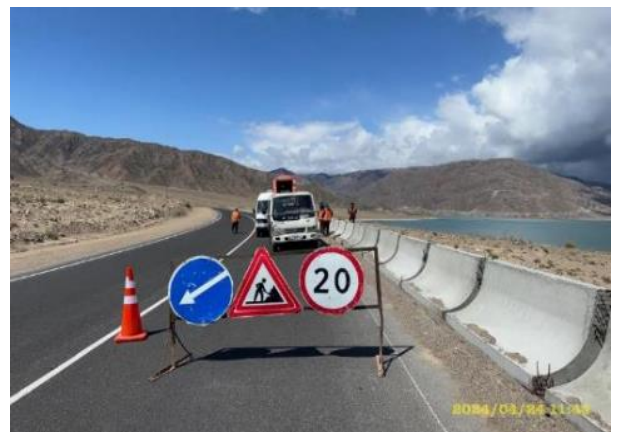
Photo 14. Parapet installation, km.41 April 2024.
