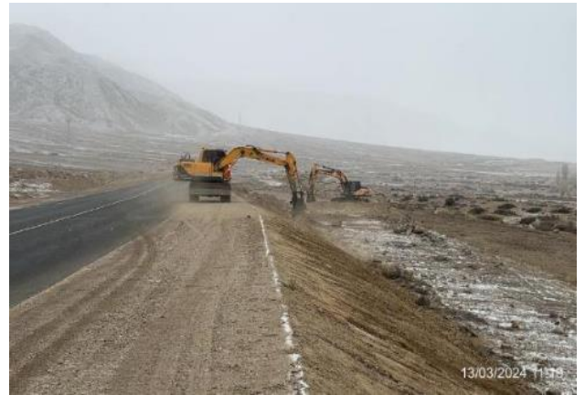
Photo 10. 36+000-38+000 RHS slope cutting. March 2024.
