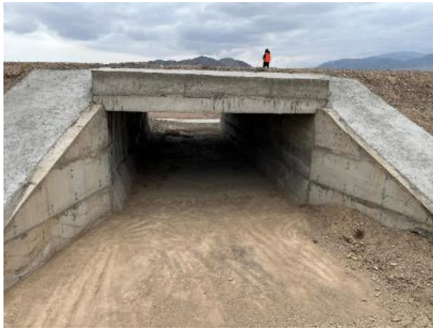
Photo 15. Lot 1, km 22+575, culvert cleaning. April 2024.
