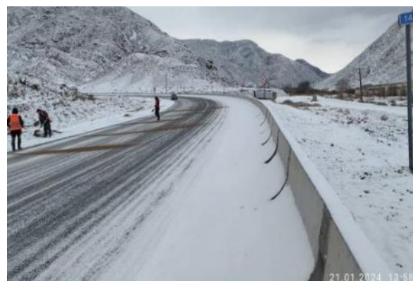
Photo 6. Sprinkling of mixture against icing, km.14+000. January 2024.
