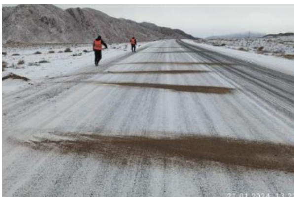
Photo 5. Lot 1. Sprinkling of sand-salt mixture against icing, January 2024.
