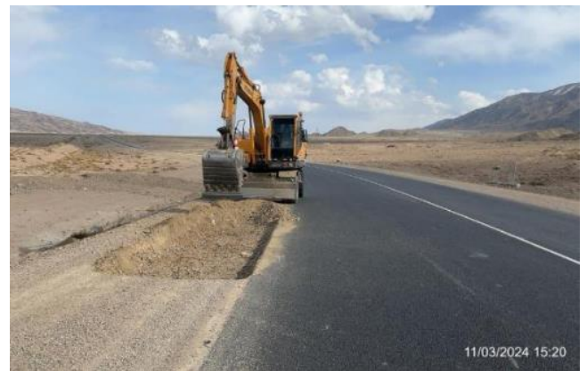
Photo 12. Installation of parapet foundation 34+680-34+905 RHS. March 2024.
