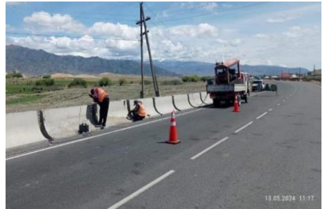
Photo 31. Welding of parapets km 88+860-88+790 RHS. May 2024.
