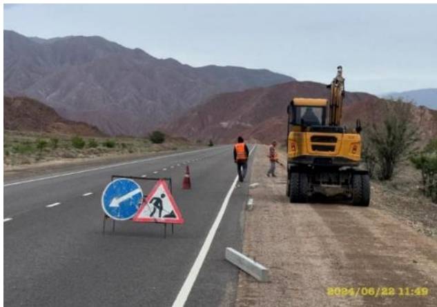
Photo 19. Lot 1. Installation of roadside posts 18+500 RHS June 2024.
