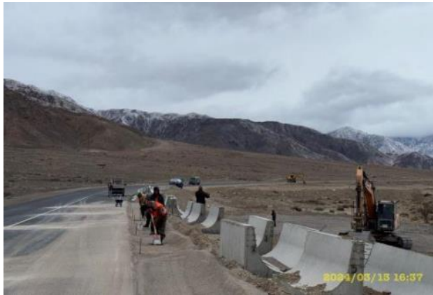
Photo 9. Lot 1. Installation of parapets km. 37+540. March 2024.
