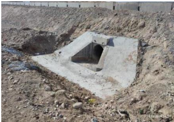
Photo 26. Construction of pipe inlet reinforcement, km.88+692. March 2024.
