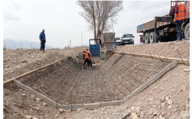
Photo 27. Concrete pouring for slope reinforcement km 64+860. April 2024.
