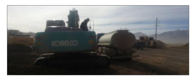
Figure 32: Onsite refueling of plant by dedicated refueling truck
