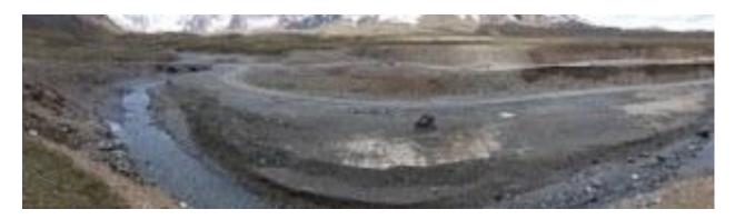
Figure 30: Muz Tor River Borrow Area – Note regrading on far bank, levelling forground
