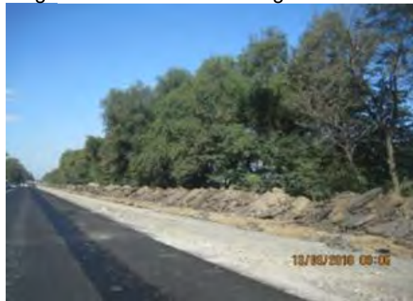
Figure 3 Removal and taking out of excess soil
