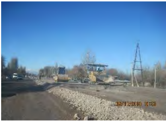
Figure 4 Roadbed compaction
