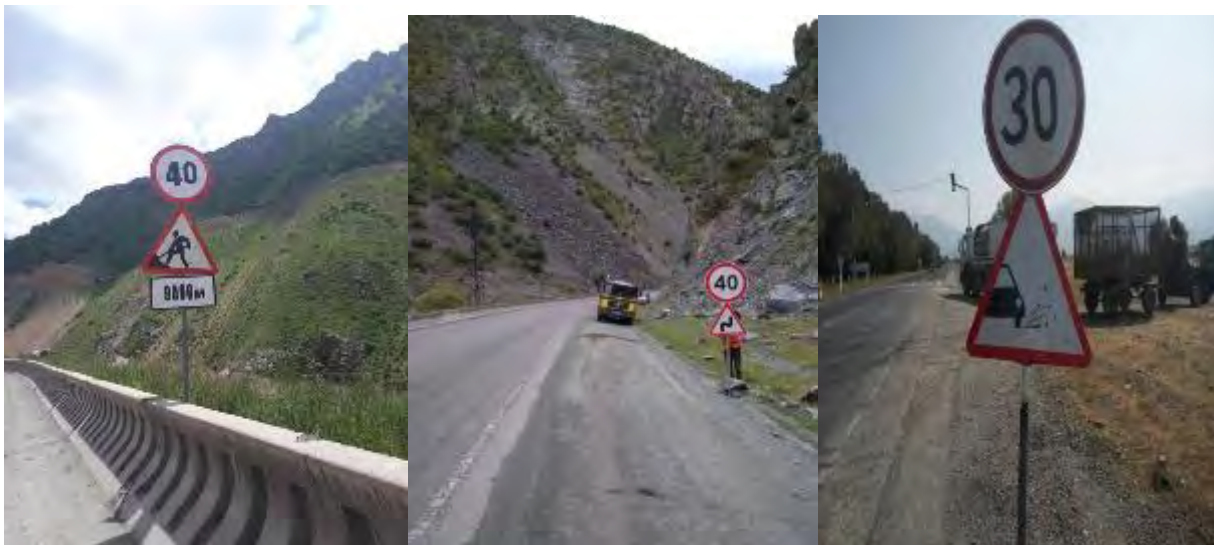
Figure 3 Installation of road signs
