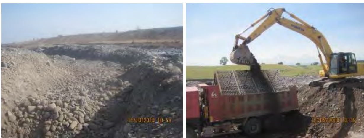
Figure 15 Development of Ak-Suu 2 borrow-pit
