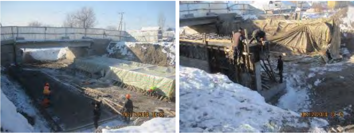
Figure 11 Construction of the bridge at KM 44+641
