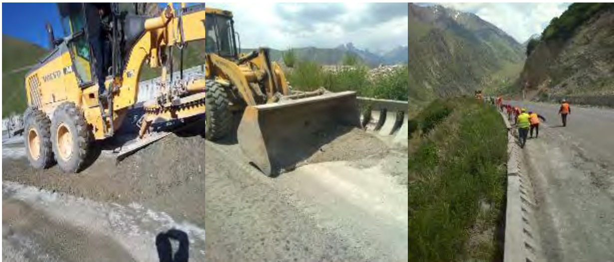
Figure 4 Works along the parapets
