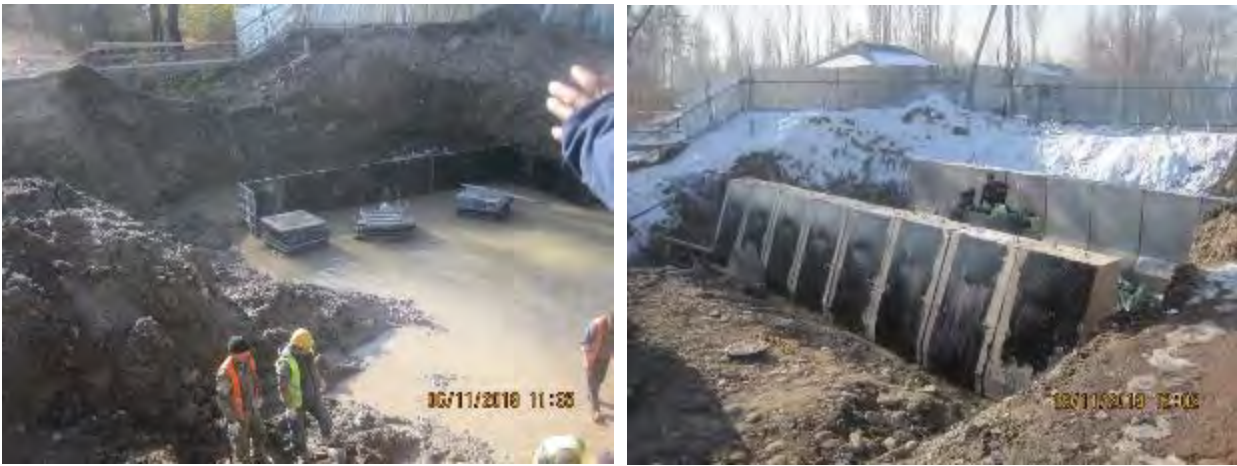
Figure 12 Construction of the bridge over Jantay canal
