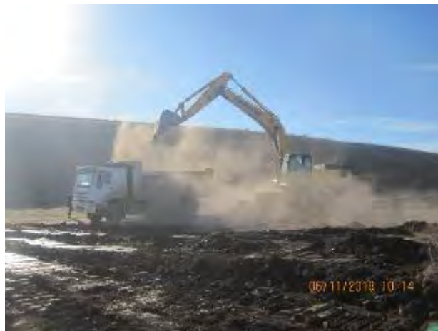
Figure 66 Operation of equipment without water sprinkling, with causing harm to the health of workers
