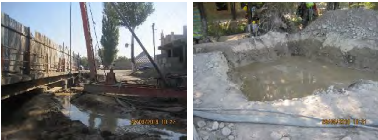
Figure 7 Construction of the bridge over Sokuluk River. Bentonite pit
