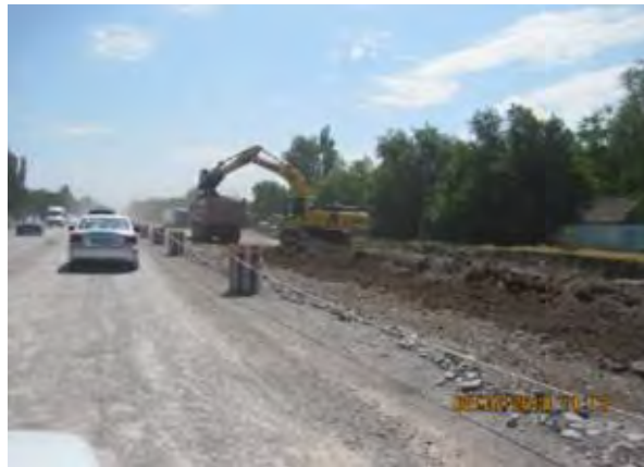
Figure 3 Removal and taking out of excess soil
