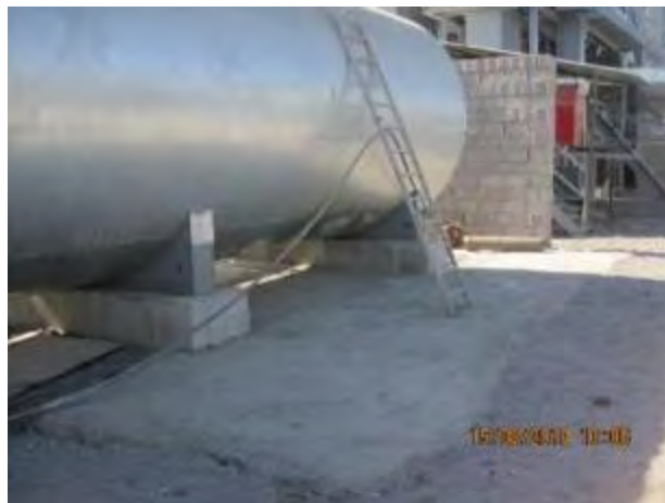
Figure 45 Impermeable protective coating around the tanks with chemicals
