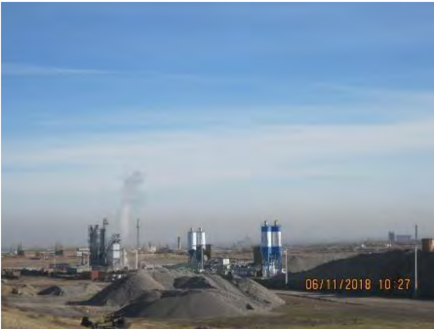
Figure 18 Production site of the asphalt plant
