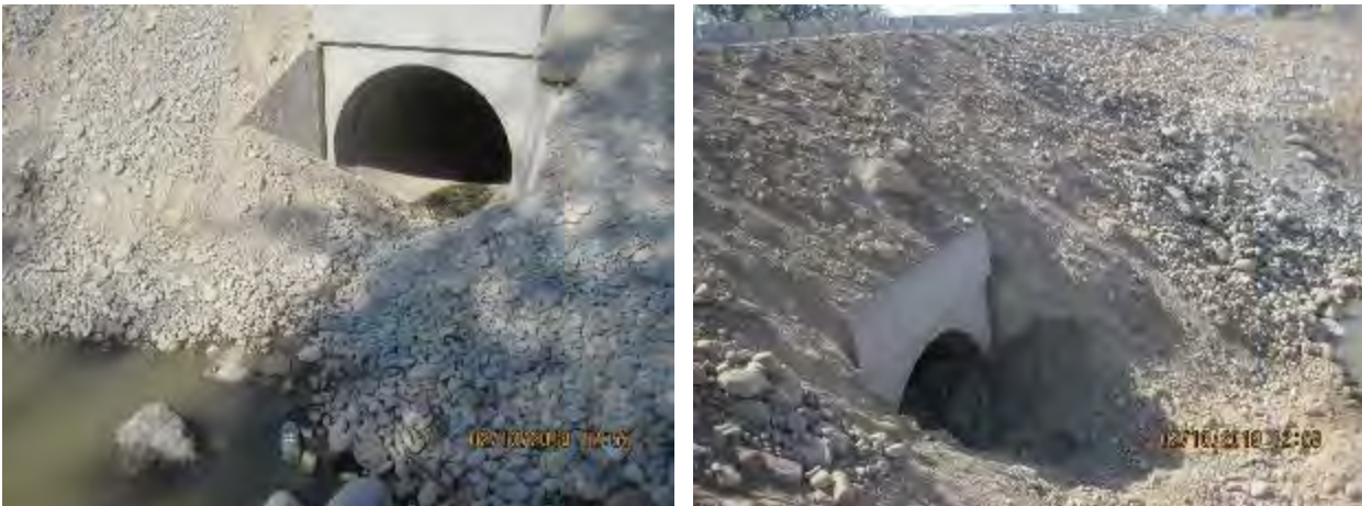
Figure 32 Overlapping of inlet and outlet holes of the pipe caused by gravel shedding
