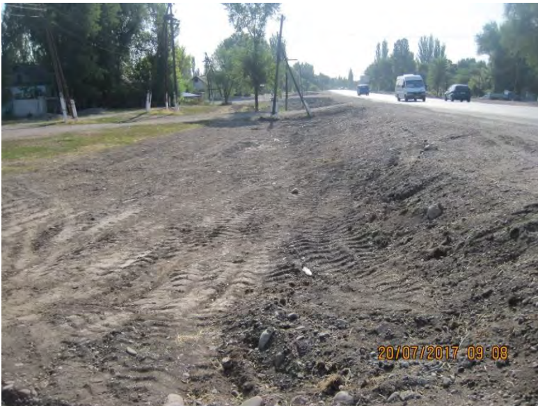
Figure 26 Road section with the removed topsoil
