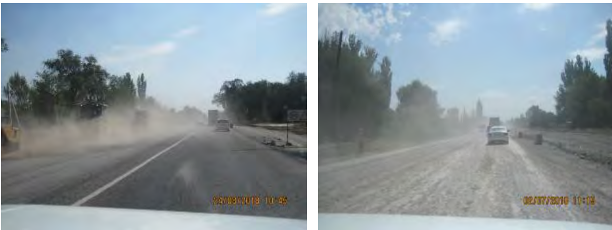
Figure 30 Increased dust formation at construction sites
