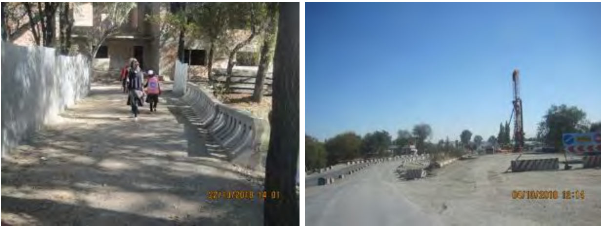
Figure 8 Pedestrian crossing over Sokuluk River. Road on the northern side of the bridge
