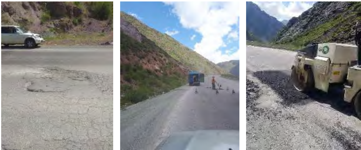
Figure 2 Current repair of the roadbed
