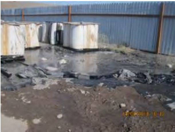
Figure 42 Leakage of bitumen to the soil
