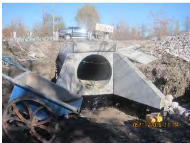
Figure 13 Construction of culverts
