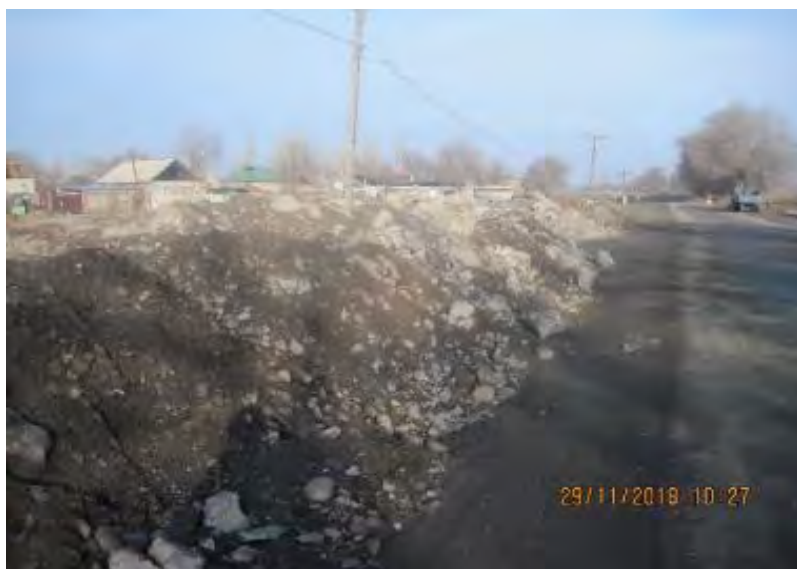
Figure 35 Construction waste at the northern side of the bridge under construction
