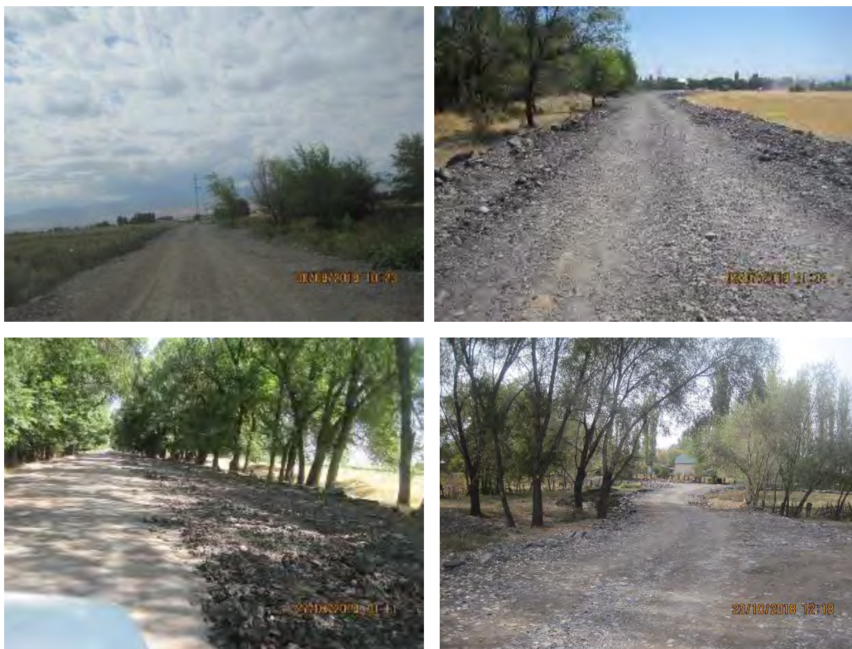
Figure 62 Taking out of old asphalt for backfilling of rural streets
