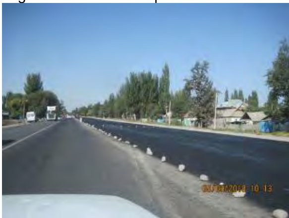
Figure 5 Laying of new asphalt
