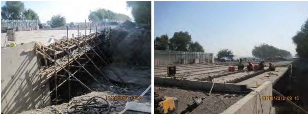
Figure 6 Construction of the bridge over Jelamysh river
