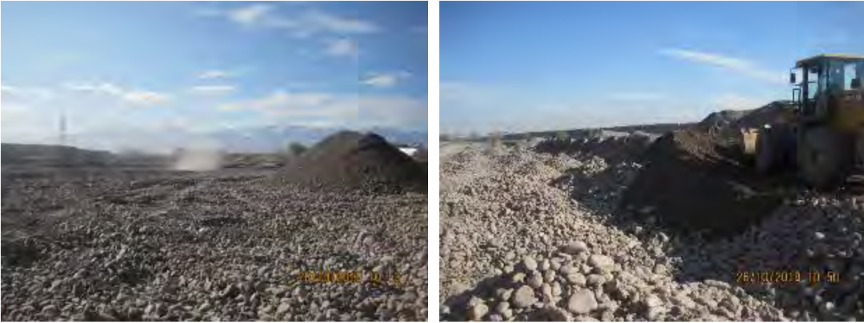
Figure 40 Development of Kara-Balta borrow-pit
