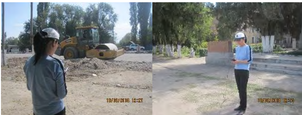
Figure 57 Vibration monitoring at the construction sites
