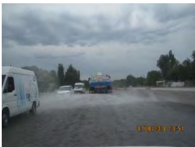
Figure 14 Water sprinkling at work sites
