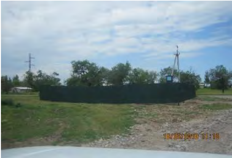
Figure 25 Restored well for water supply to the plant
