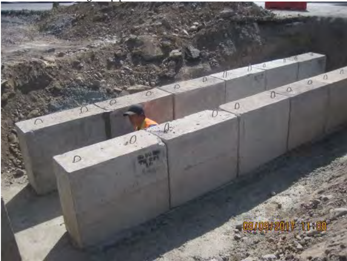
Installation of rectangular pipes
