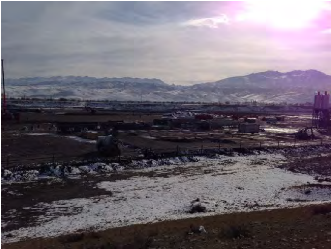
Figure 16 Ak Suu2 site for materials processing operation. Note start of fencing.
