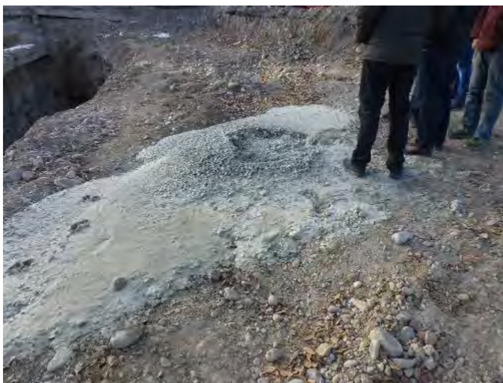
Figure 13 Zhelhamish River: A-major work while river is active and B-concrete spill on the bank
