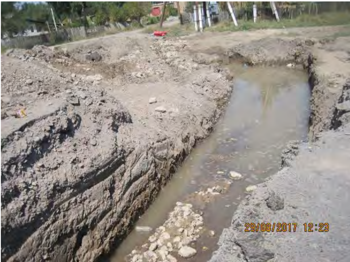
Driven out a wedge groundwater causes problem.
