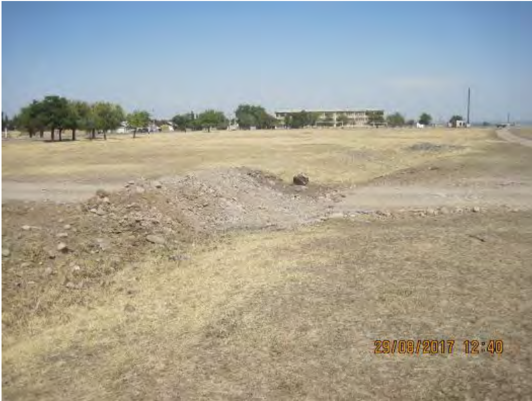
On the Aksu 1 borrow pit no work was done. All equipment from the borrow pit is taken out.
