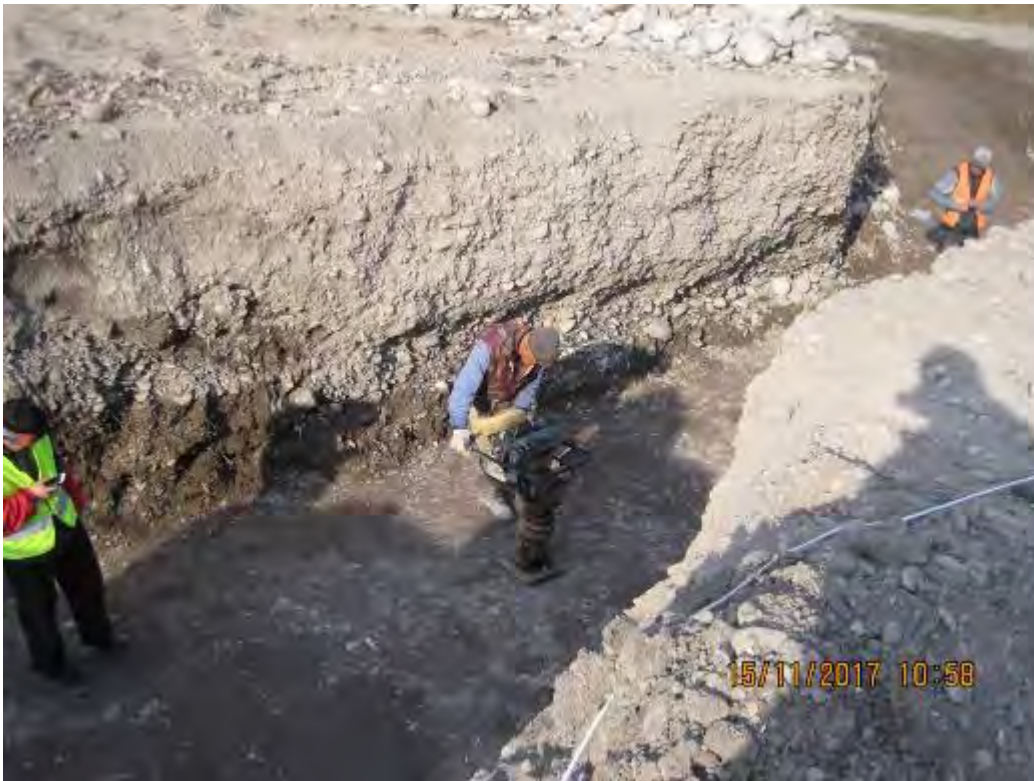
The photo shows the tamping of the base under the culvert
