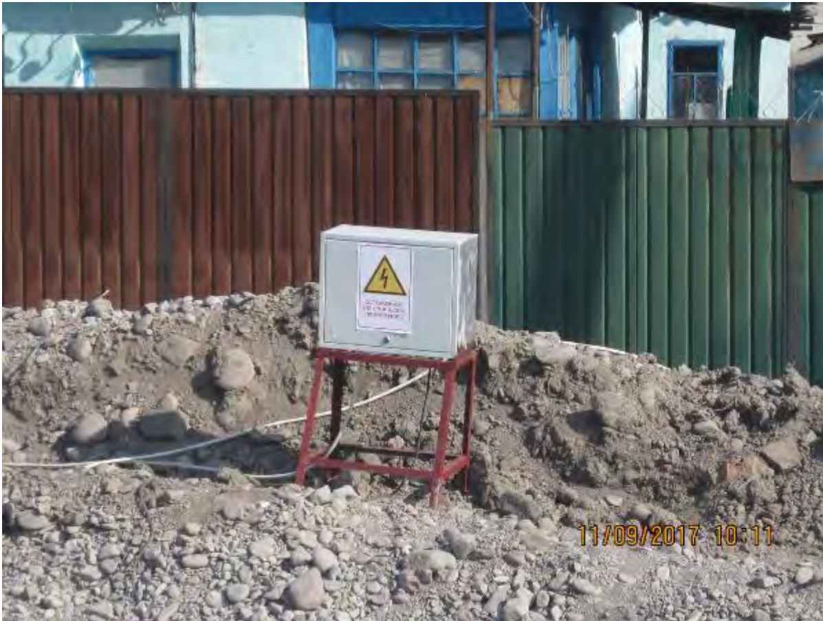
Transformer for providing night-time lighting of problem zones on roads (where pipes are installed).
