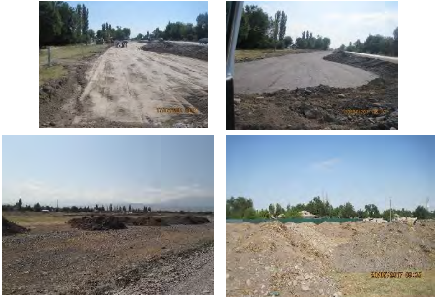
Figure 10. Subgrade preparation and topsoil storage Section 3.
