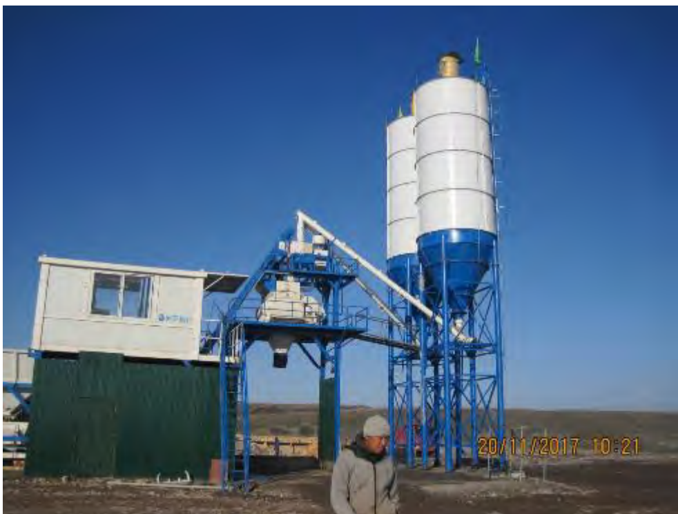
The construction of a concrete plant
