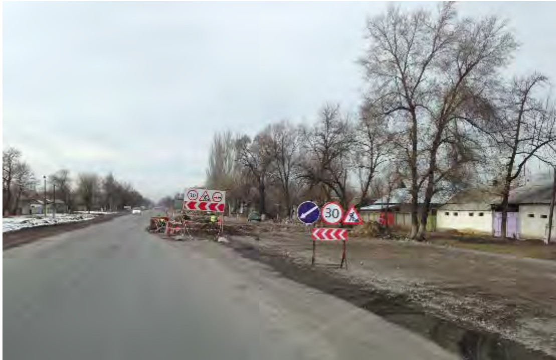
Figure 12. Culvert construction site in Section 3 showing standard diversion
