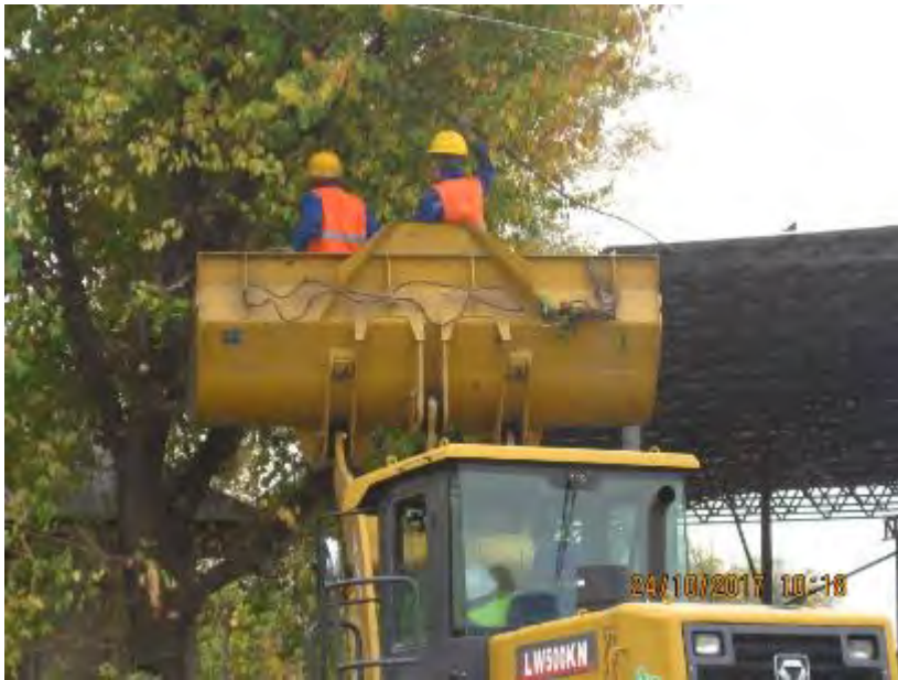
In violation of safety regulations, due to the lack of a lift, workers are working at a height in the loader bucket
