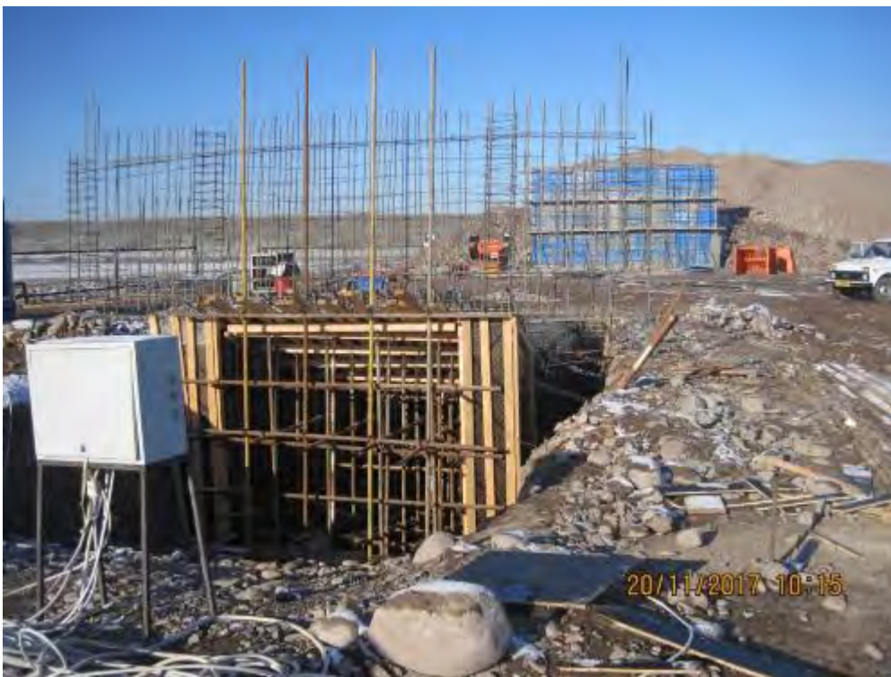
Photographs shows the construction of a foundation for a stone crusher
