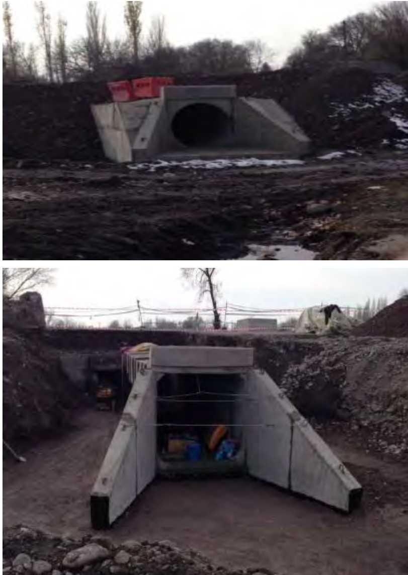
Figure 14. Two types of poured-in-place culverts under construction
