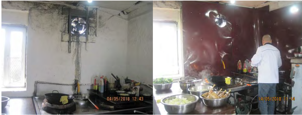
A washable plastic non-combustible coating on kitchen wall at Sokuluk Construction Camp
