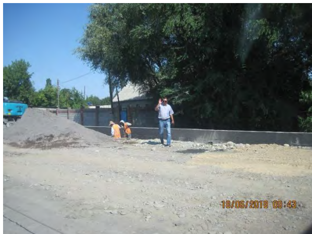
Figure 10. Retaining wall construction site
