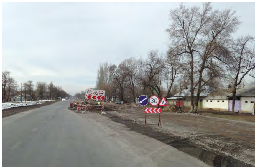
Figure 9. Culvert construction site in Section 1.3 showing standard diversion signage
