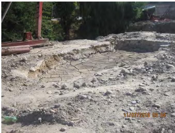
Pit for dehydration of bentonite clay to be removed to secure landfill site for burial.
