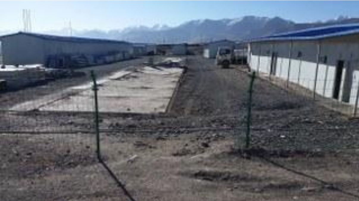
Figure 2: Accommodation units being dismantled (23 rd September 2016)
