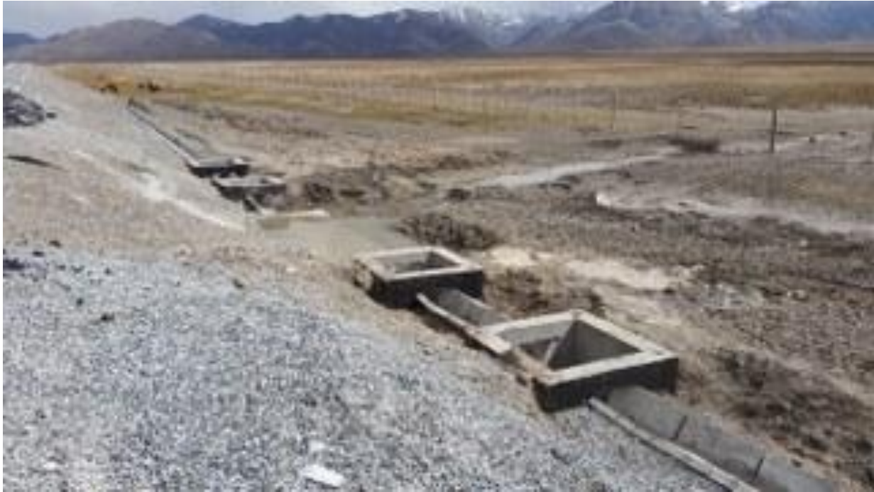
Figure 12: Spill Controls under construction (June 2016)
