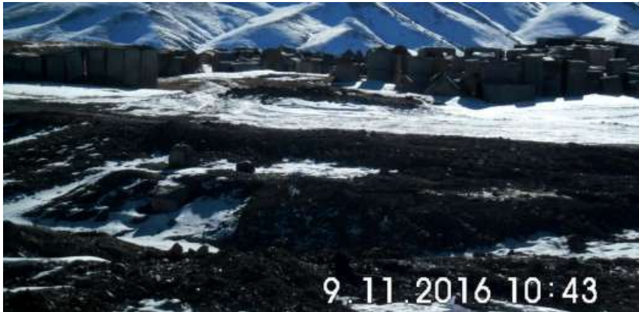
Figure 4: Salvaged culvert units / unused precast for MoTC use. Entrance to old camp Km501
