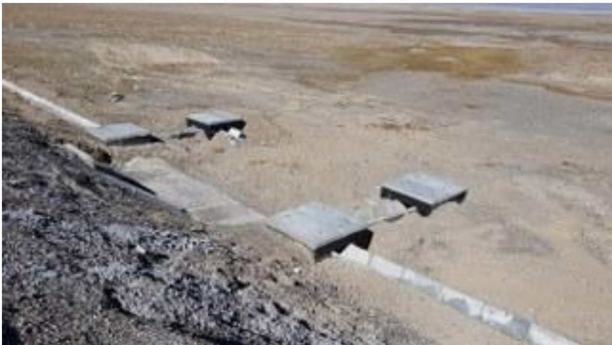
Figure 13: Spill control completed (September 2016)
