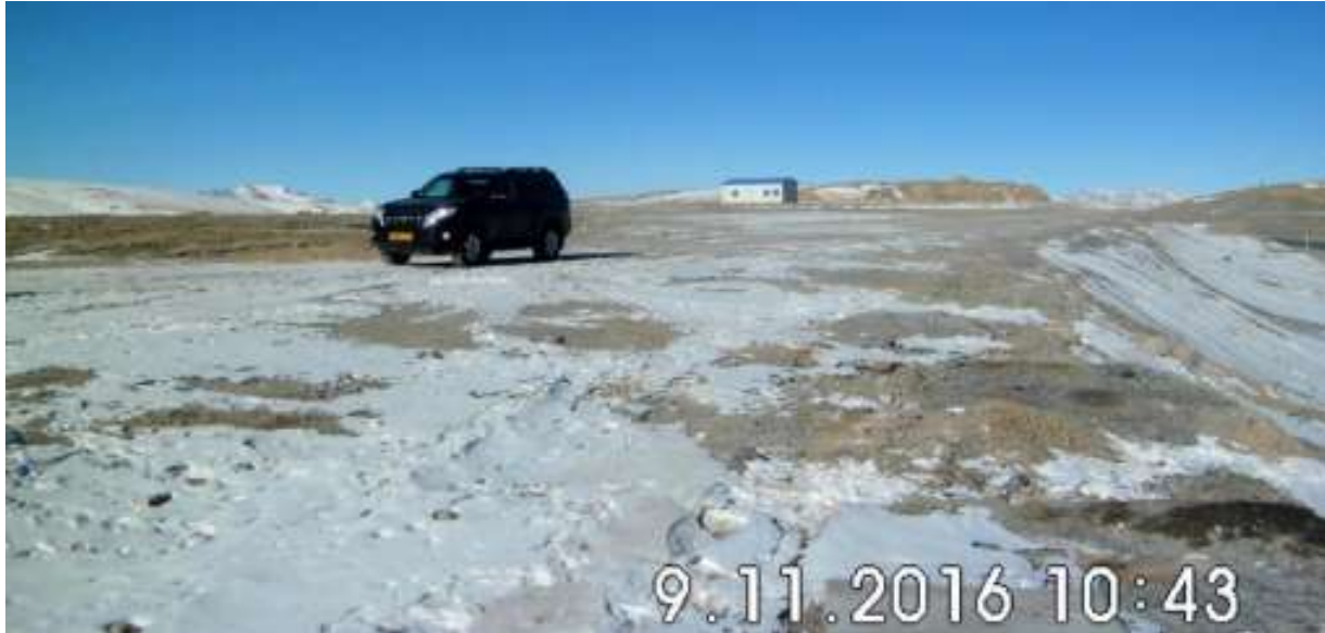
Figure 3: Camp buildings at Km501 cleared. One accommodation building retained for MoTC use and as emergency refuge
