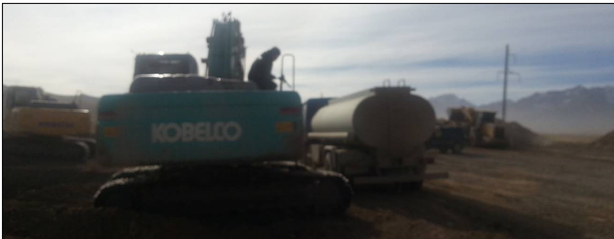
Figure 19: Onsite refuelling of plant by dedicated refuelling truck
