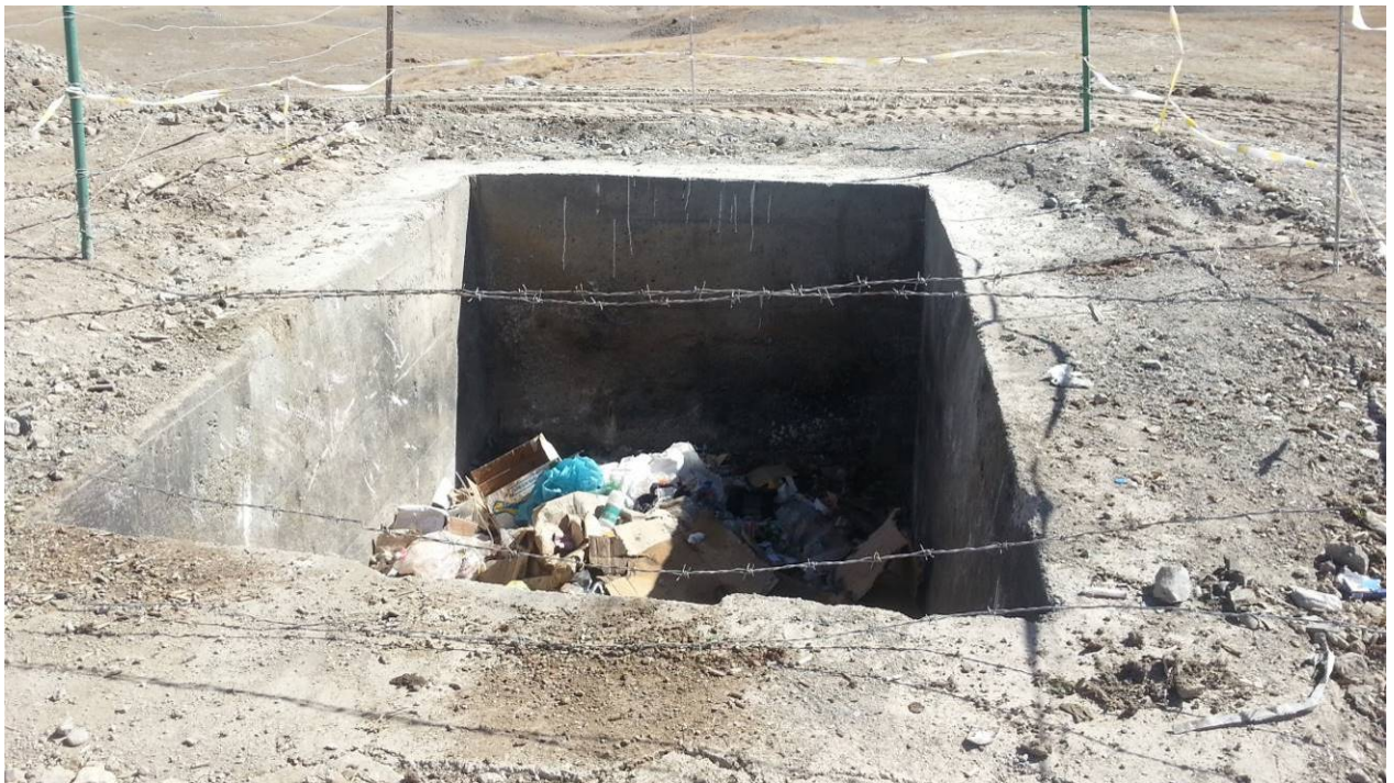
Figure 23: Fenced solid waste transfer point – Waste is collected and disposed to At-Bashy
