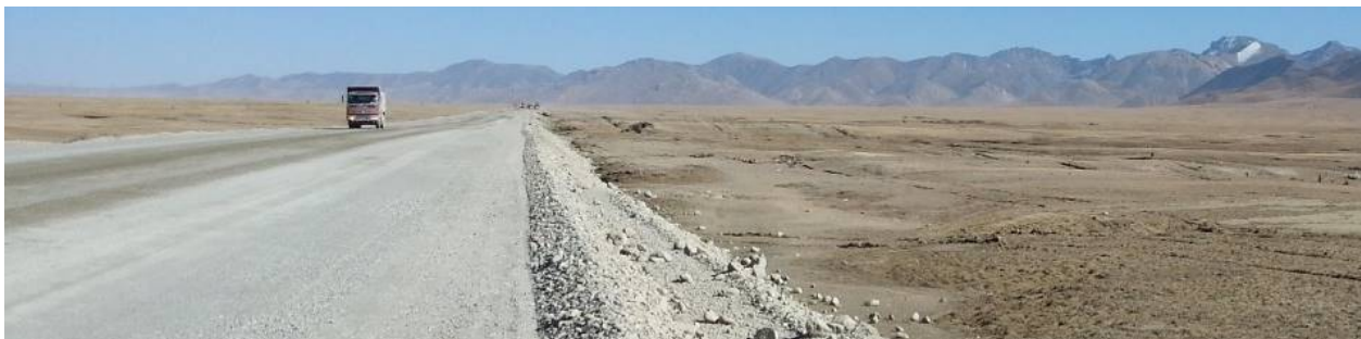
Figure 4: Typical Road Alignment after 2013 works on road foundation (around Km 502)
