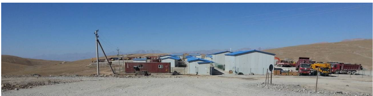
Figure 2: Construction Camp at Km500 looking North across Maintenance Area
