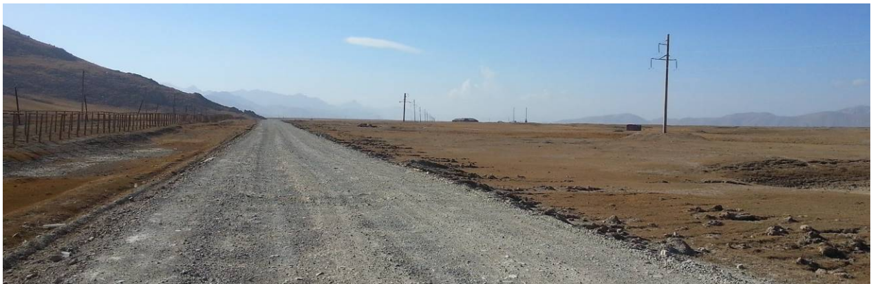
Figure 3: Typical Road Alignment prior to works (around Km520)
