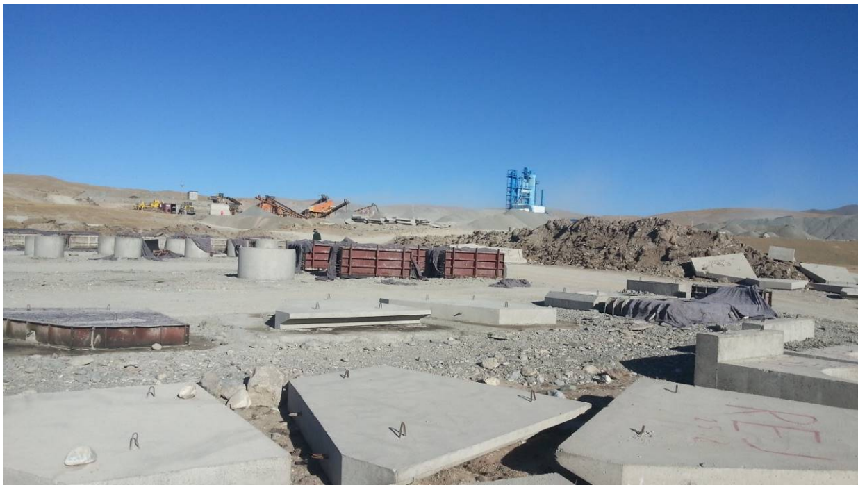
Figure 16: Precast Concrete production, asphalt plant, crushing and grading areas
