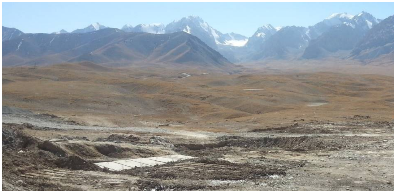
Figure 21: Septic Tank installed behind Camp – Emptied to facility at Naryn
