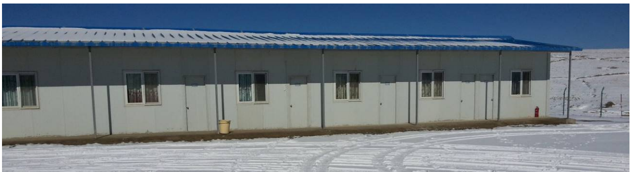
Figure 24: Waste bins and fire extinguishers provided at Camp
