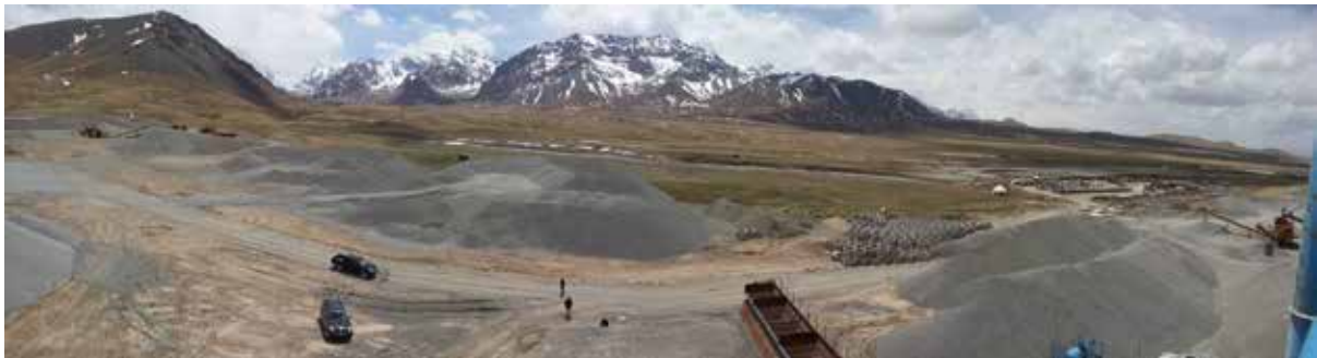
Figure 8: Manufacturing Area looking south-west from Asphalt Plant across Muz Tor River
