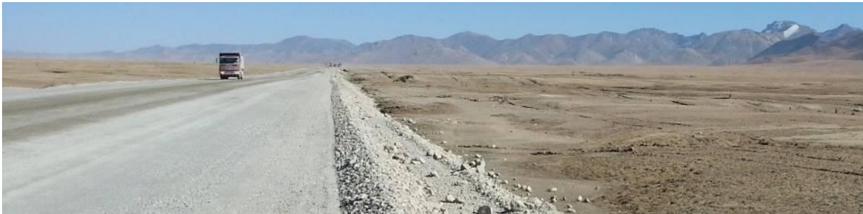
Figure 11: Typical Road Alignment after works creating road foundation (around Km 502)
