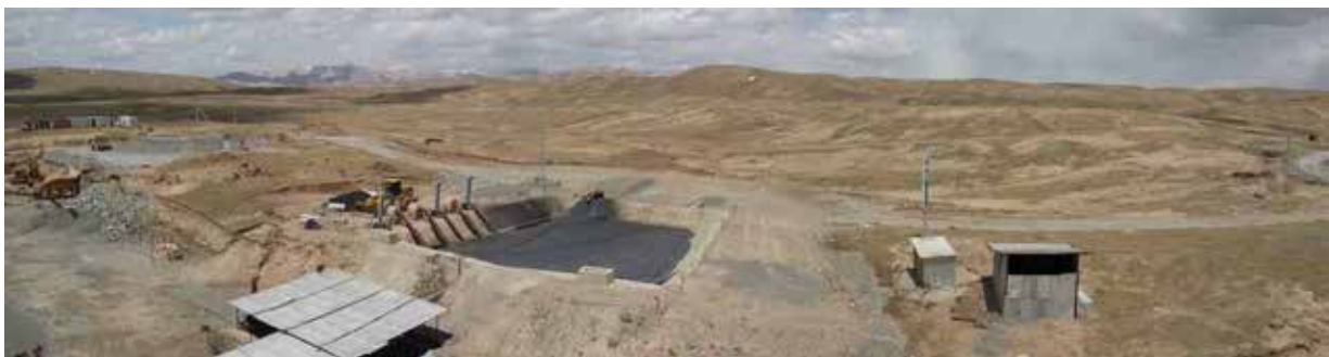
Figure 9: Manufacturing Area looking north-east from the asphalt plant
