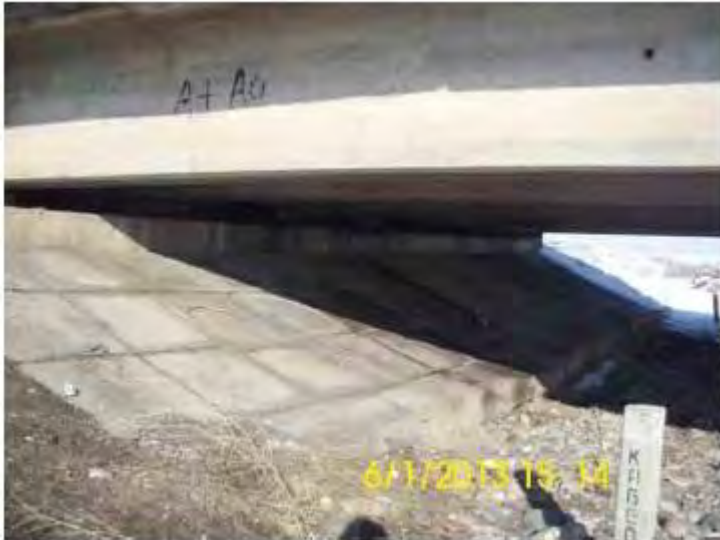
Fig. 6: An example of bridge slope protection for Kara-Unkur river bridge.
