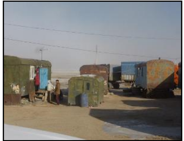
Photograph 4 View of dilapidated caravan-trailers from south (looking north-)
