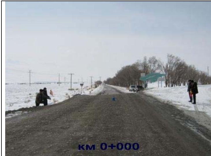
Photo 1 The turn-off from the main road to At-Bashy village. Zero reference point. The blue cone – indication of the center line.
