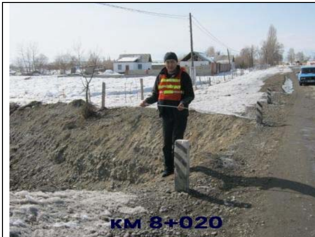
Photos 76 and 77 The crossover of the road with the drainage channel is both on the left and the right shots, the carriageway is slightly narrowed (down to 8.5 m)
