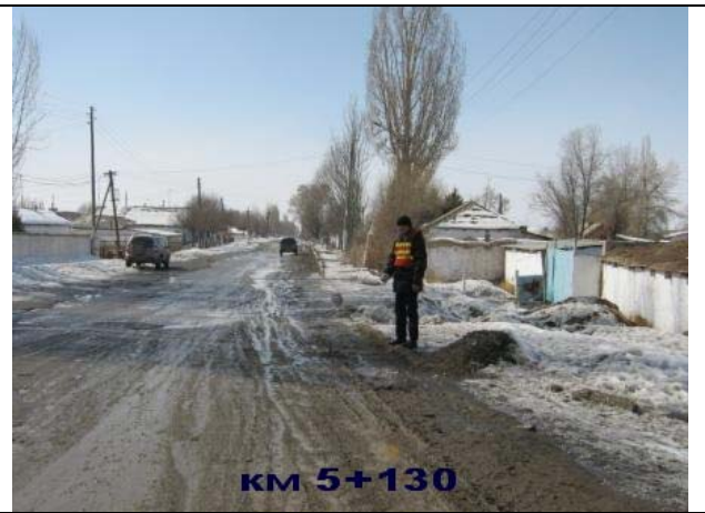
Photos 39 and 40 The condition of the sidewalks can be seen on the right and on the left sides of the road, the sidewalks are covered with snow and damaged in some areas. A cob fence on the left is 2 m away from the road edge.
