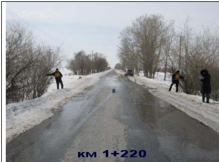
Photo 15 Roadside plantings. The specified points on the left and on the right have isolated bushes growing at a distance of almost 1 m from the road edge
