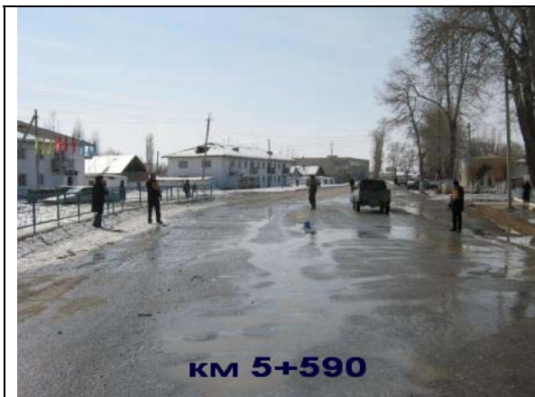
Photos 47 and 48. 10 m wide paved carriageway section
