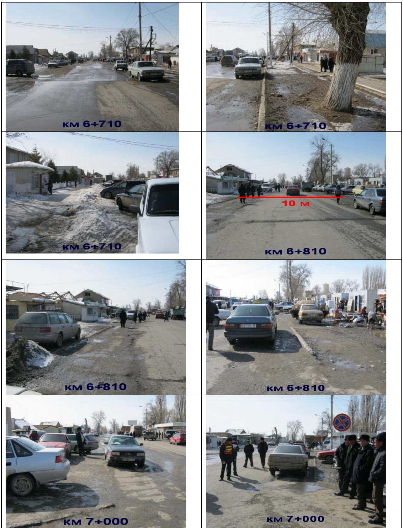
Photos 56, 57, 58, 59, 60, 61, 62 and 63 The rayon marketplace is located in the center of the village, the measurements were not possible due to the high traffic intensity. However, the distance between the curbs makes 10 m and is seen on the pictures above. The vehicle parking spaces, the sidewalks, plantings and etc. are observed to be outside the road carriageway.
