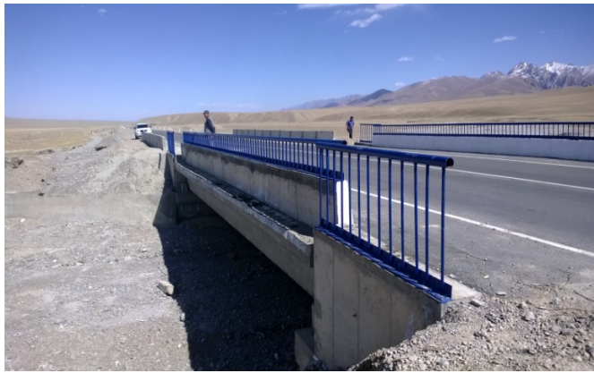
Bridge at km 460
