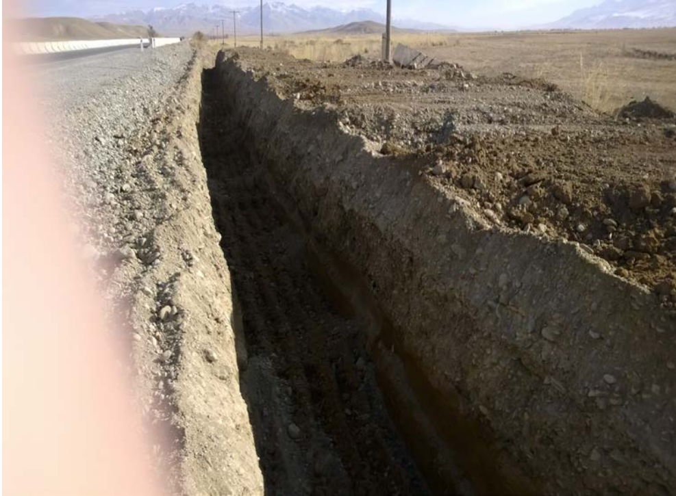
Additional drainage at km387+200
