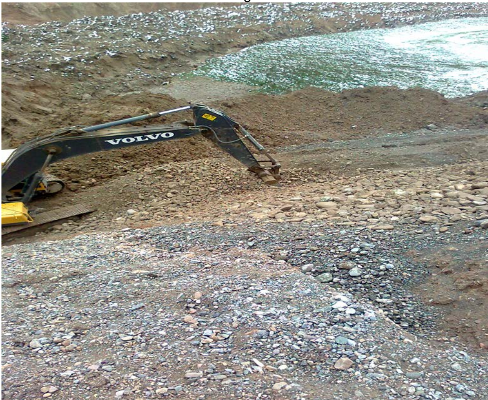
Slope stabilization against erosion at km368
