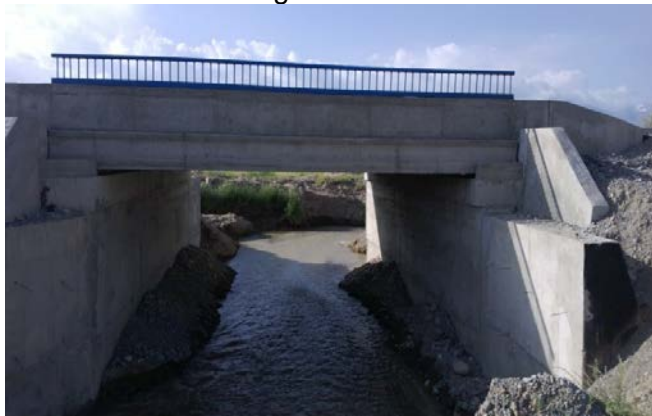
Bridge at km389+200
