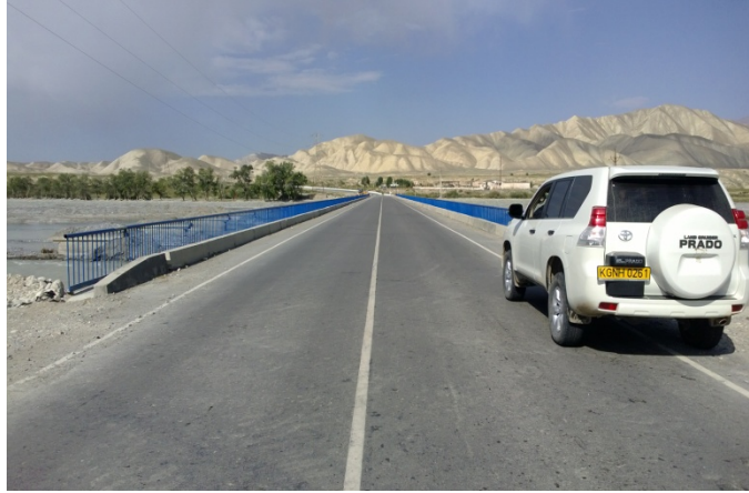
Bridge at km 400
