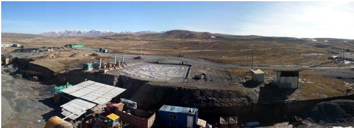
Figure 12: Manufacturing Area looking north-east from the Asphalt Plant (May 2015)
