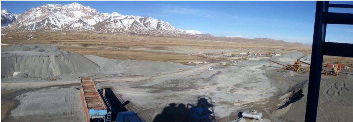
Figure 11: Manufacturing Area north-west from Asphalt Plant across Muz Tor (May 2015)
