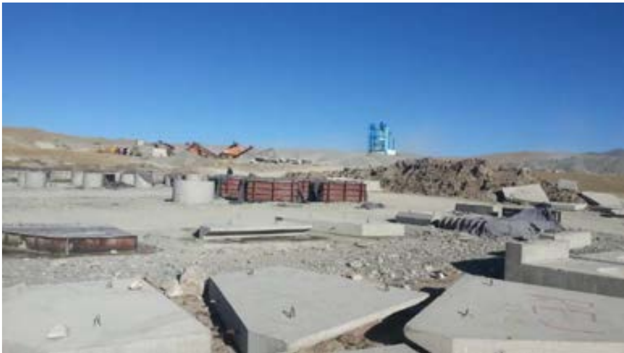
Figure 46: Precast Concrete production, asphalt plant, crushing and grading areas
