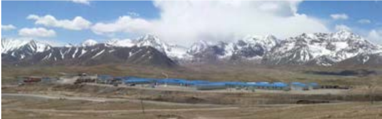
Figure 9: Construction Camp at Km501 - Looking South across Tuz Bel Pass (June 2014)
