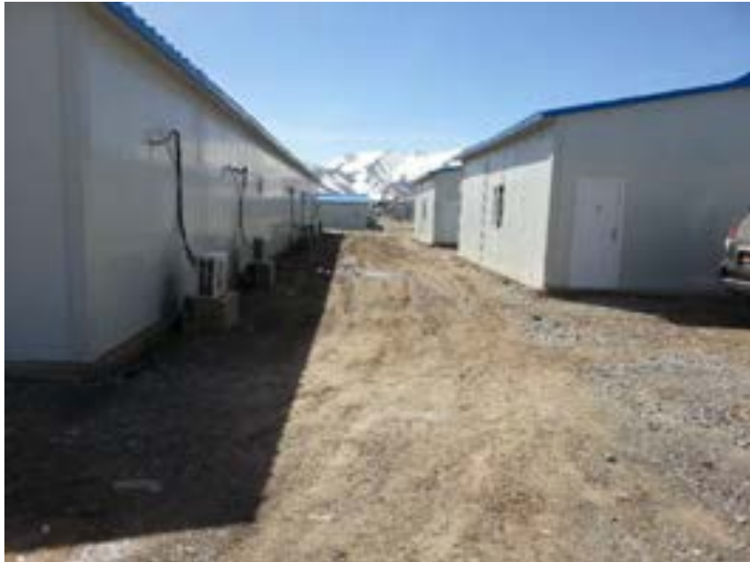
Figure 55: Camp accommodation. Note heat pumps and absence of litter
