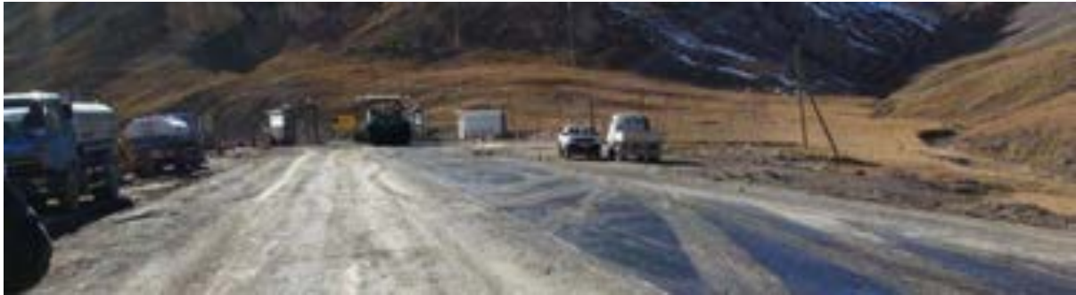
Figure 16: Asphalt upto the PRC Border (Km 539)
