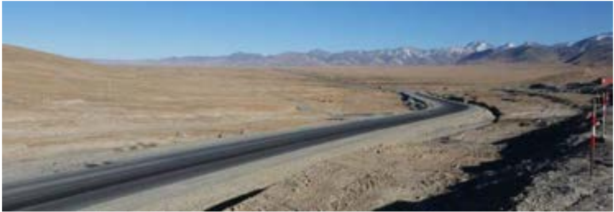
Figure 1: View from Camp on 29 Sept 2015 - note asphalt surface
