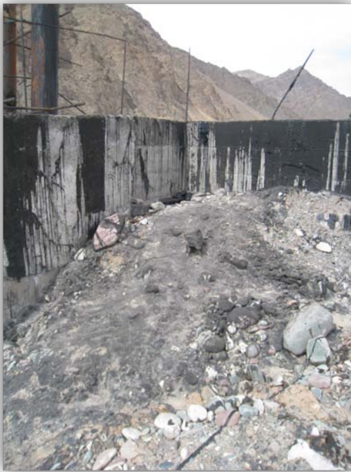
Picture 7. Asphalt plant at Team 2: numerous and big enough spots of tar at the ground
