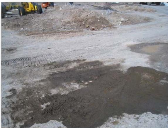
Picture 9. Spillages of fuel and oil materials at Team-2 location.
