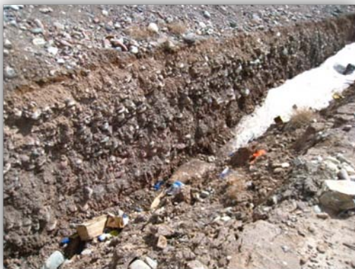
Picture 5. The enclosing ditch at Team 2 gates with garbage
