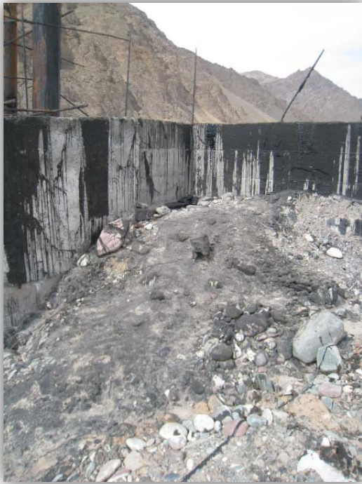
Picture 7. Asphalt plant at Team 2: numerous and big enough spots of tar at the ground
