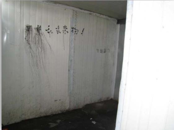
Picture 1. Toilet at Team 1 is clean
