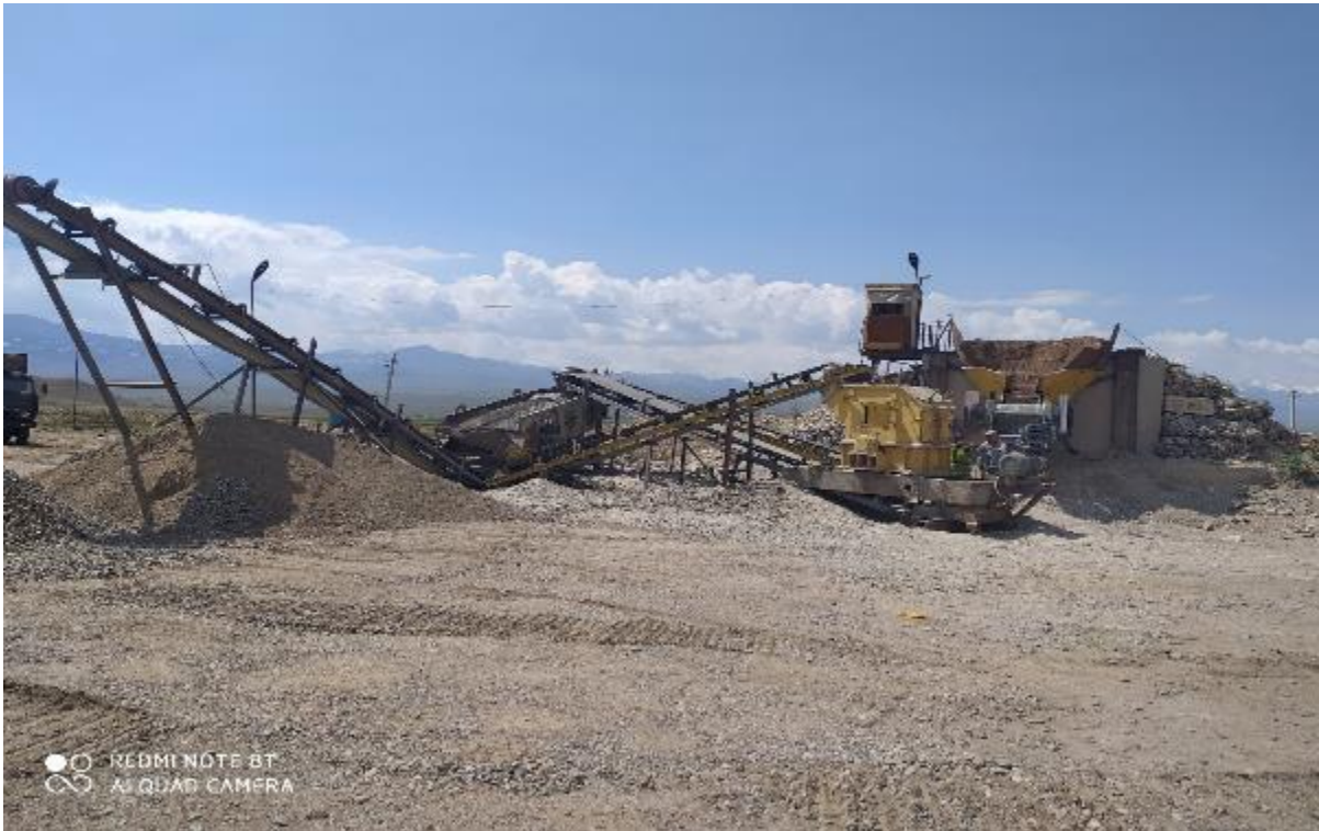
Figure 11. Crushing and screening plant on the production base
