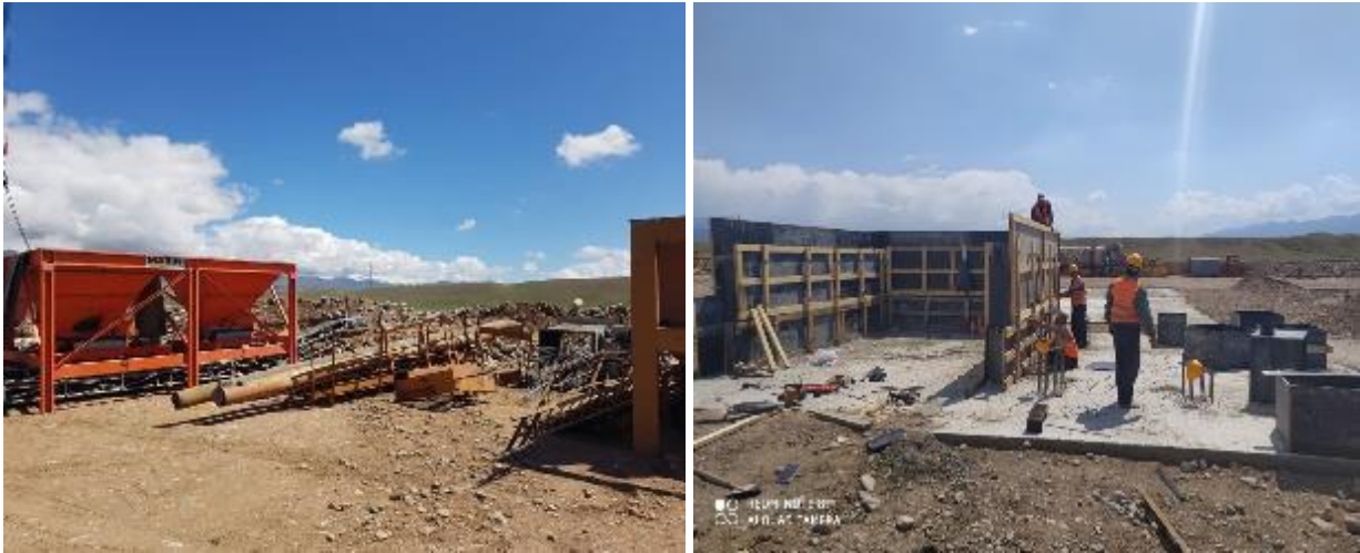
Figure 12. Mobilization and site preparation for the Asphalt Plant
