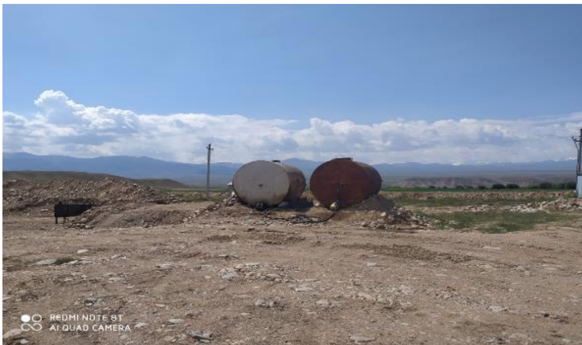
Figure 24. Tanks for fuels and lubricants
