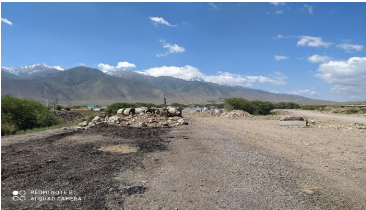
Figure 19. Stockpiling of old culverts
