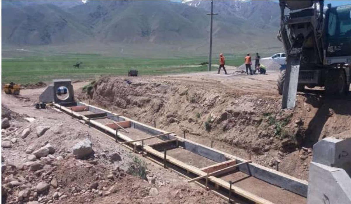
Figure 9. Culvert foundation concreting, km 93 + 280
