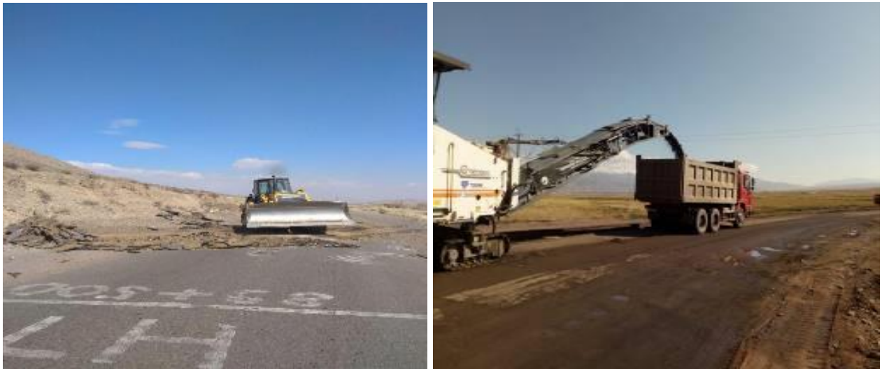
Figure 4. Removal of Old Asphalt and Unusable Soil
