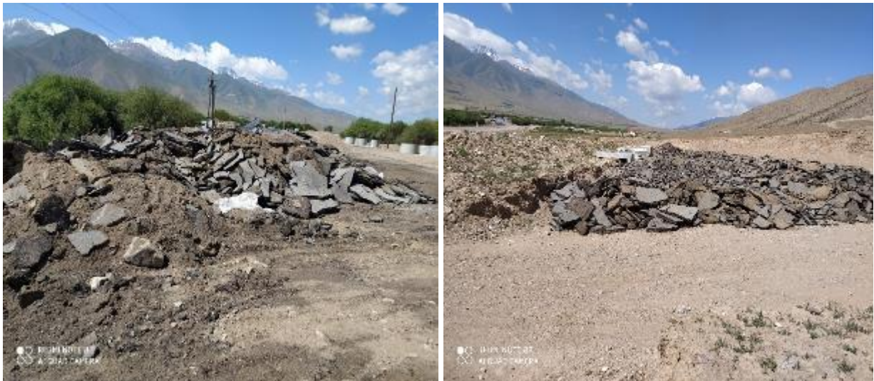
Figure 27. Old asphalt at km 91+600
