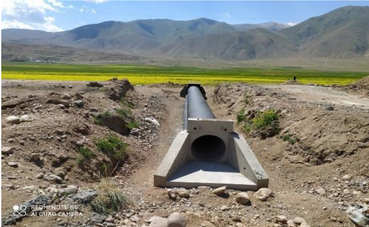
Figure 7. Construction of a culvert at km 96 + 032
