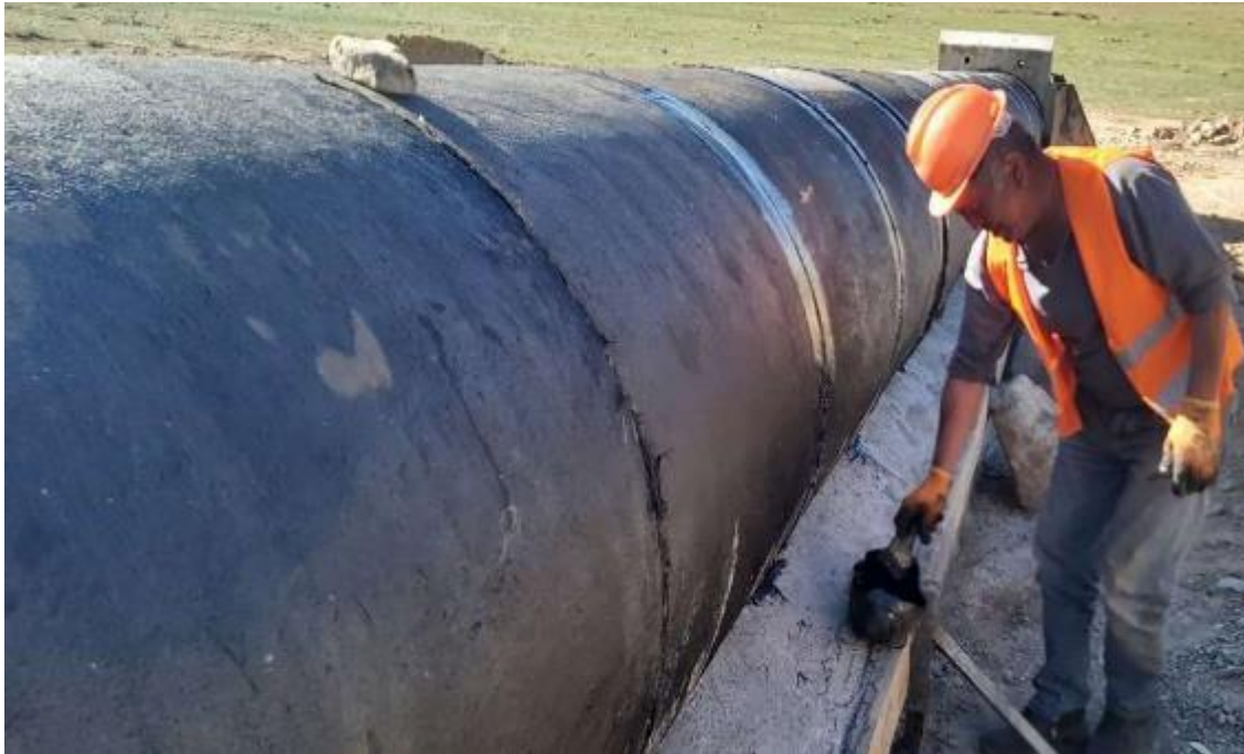
Figure 17. Waterproofing culverts with bitumen
