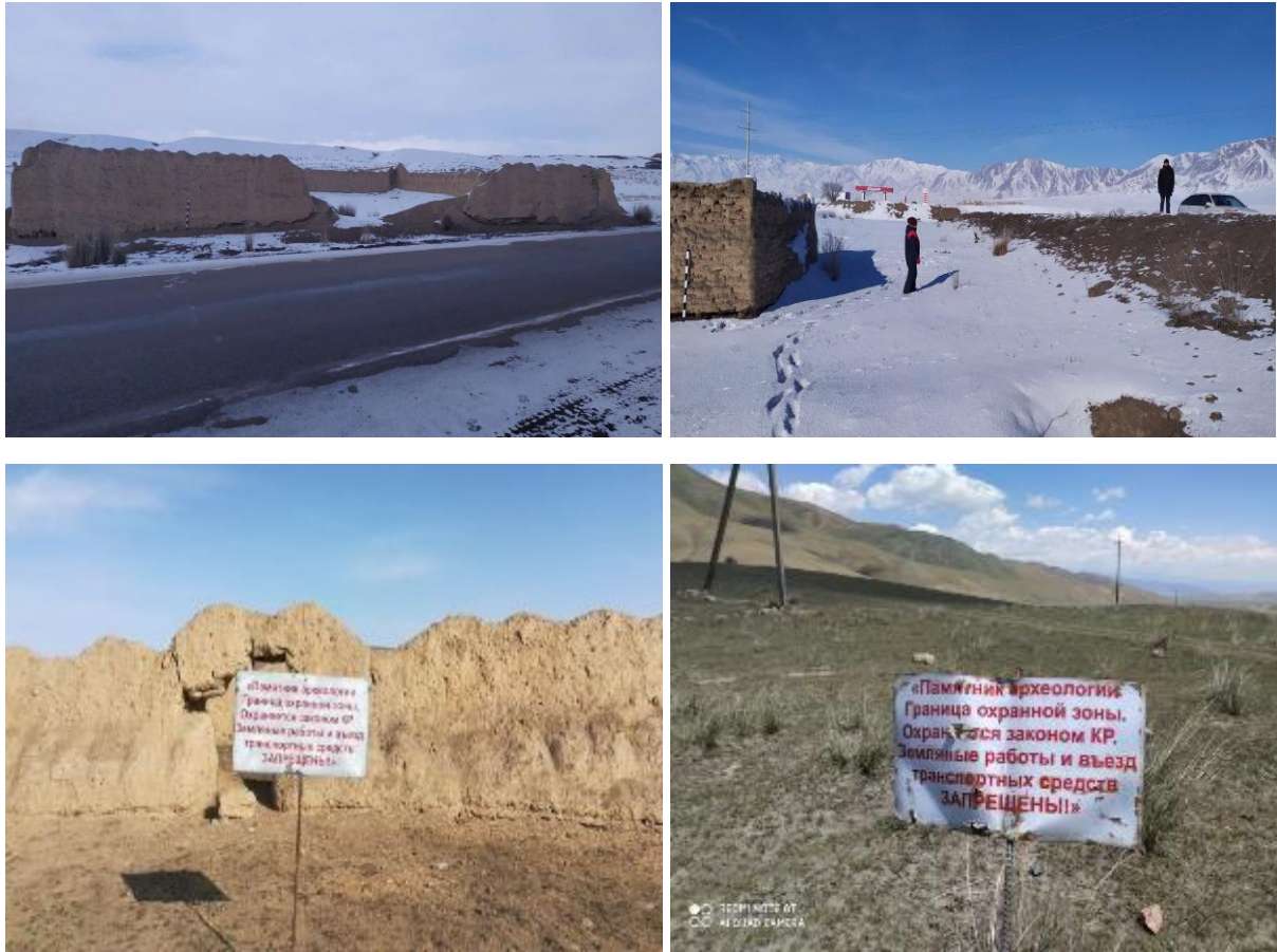
Figure 26. HCHS and protective measures
