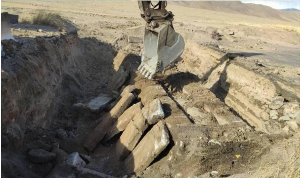
Figure 18. Existing Culverts Removal
