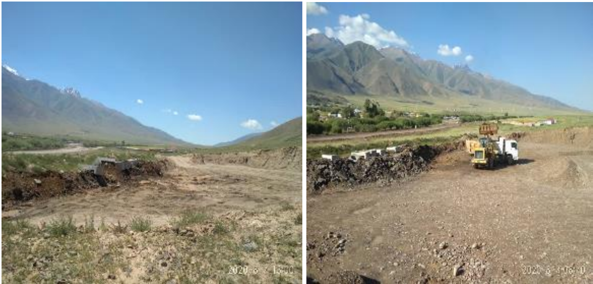
Figure 43. Old asphalt removed and cleared at km 91+360
