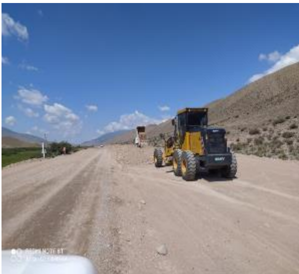
Figure 6. Embankment Raising with Inert Material
