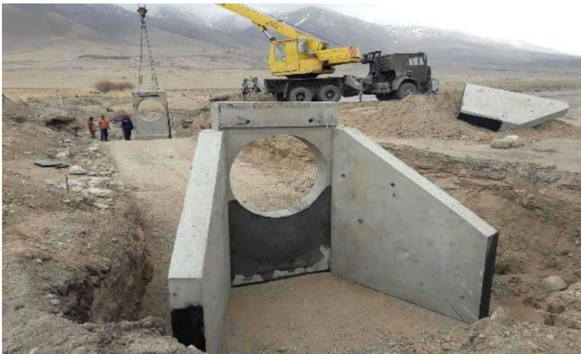
Figure 8. Installation of prefabricated cast elements
