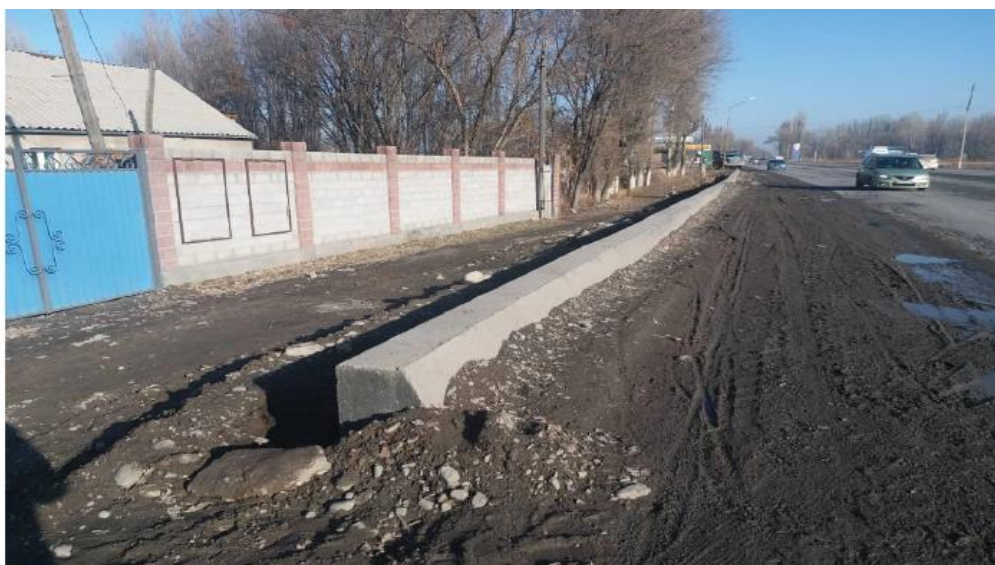
Photo 1 Retaining wall in Gavrilovka village (km 20+080)
