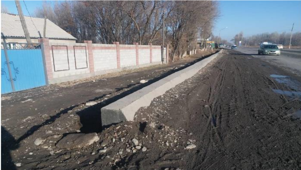
Photo 1 Retaining wall in Gavrilovka village (km 20+080)
