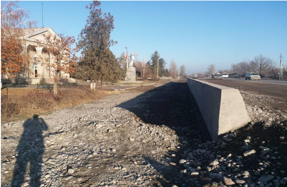
Photo 4 Retaining wall in Poltavka village (km 54+296)
