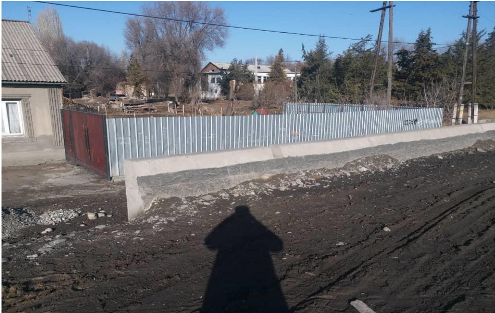
Photo 2 Retaining wall in Romanovka village (km 21+570)
