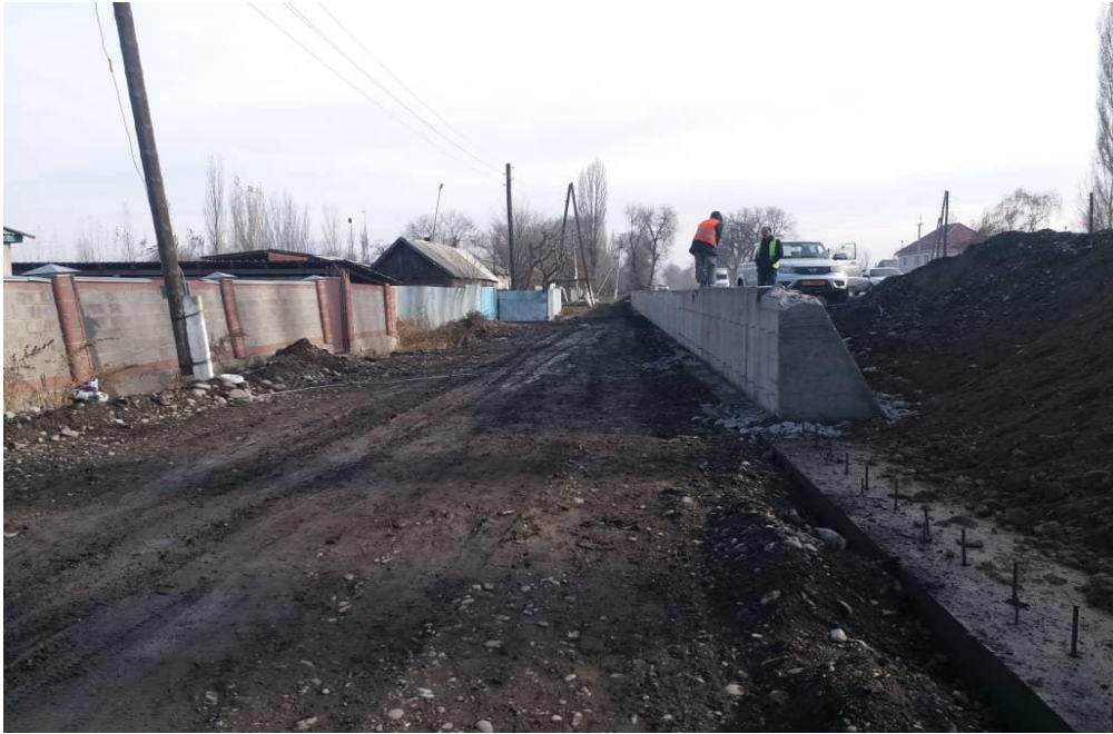
Photo 3 Retaining wall in Petrovka village (km 45+419)
