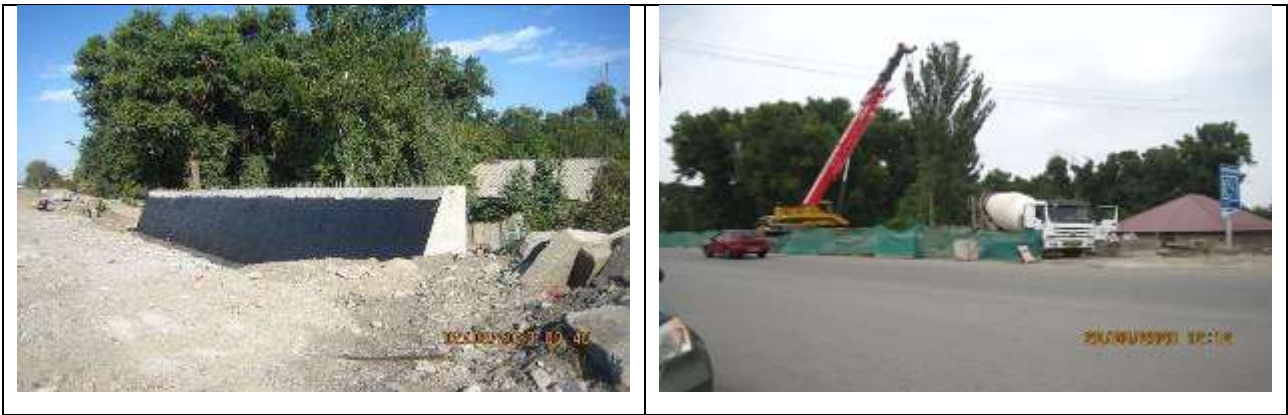
Figure 37 Construction of a retaining wall at km 26+500
