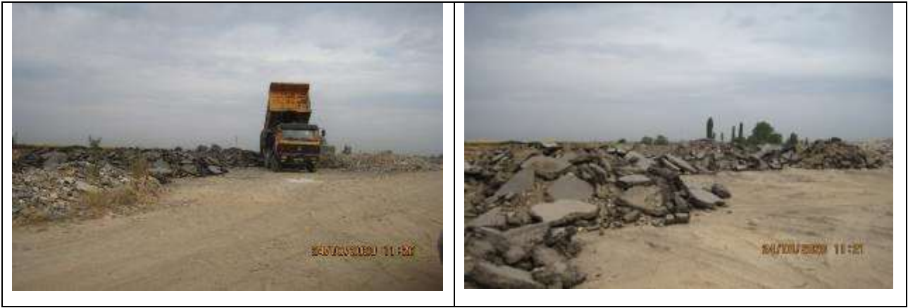
Figure 24 Dumping old asphalt on designated sites for further use
