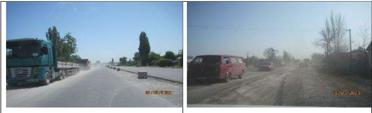
Figure 30 Increased dust formation at construction sites
