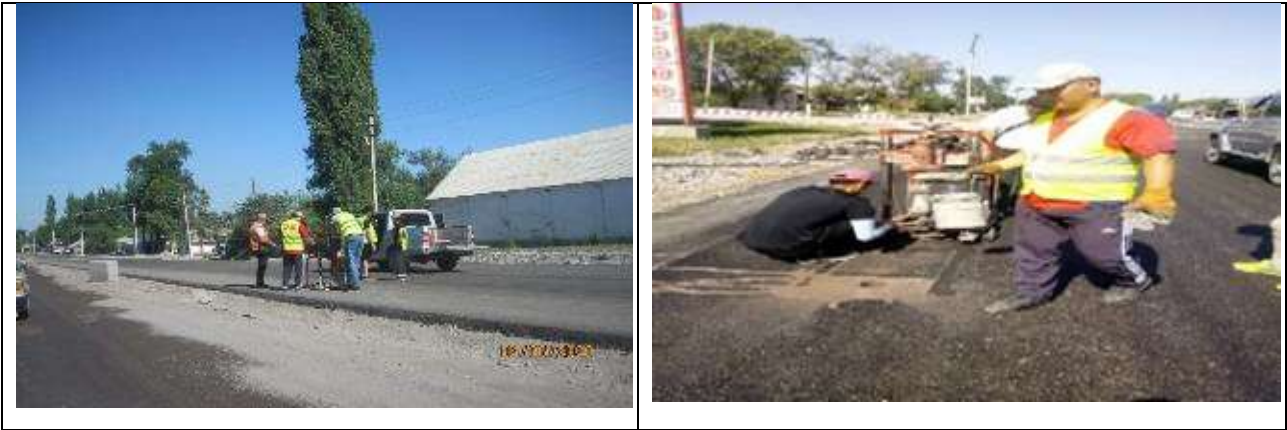
Figure 6 Sampling works for asphalt quality control
