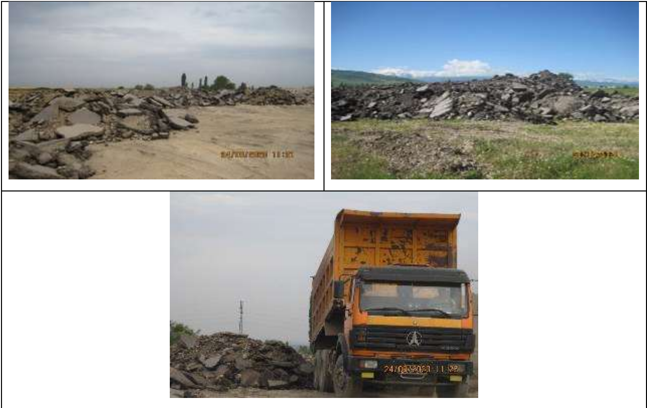
Figure 53 Dumping of old asphalt on a dedicated area for further use
