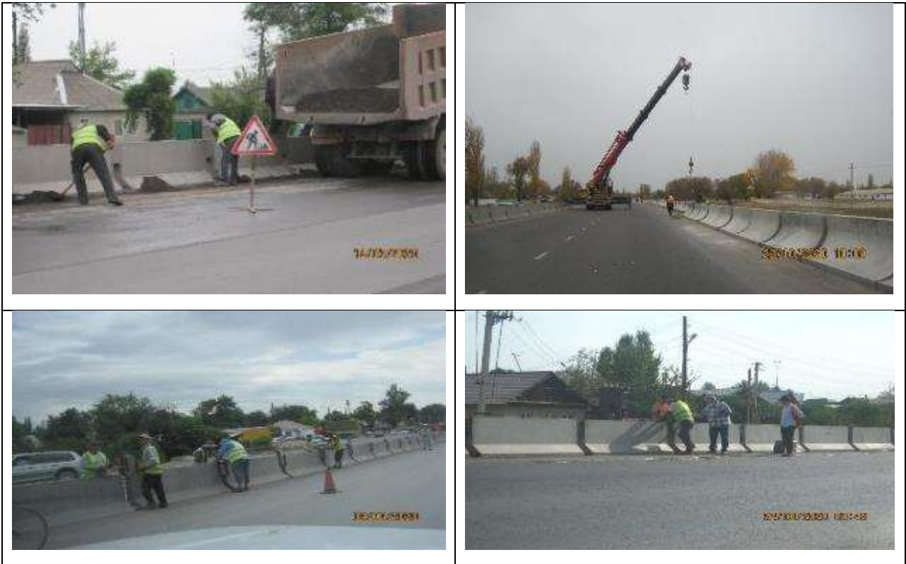
Figure 8 Installation and strengthening of New Jersey type parapets
