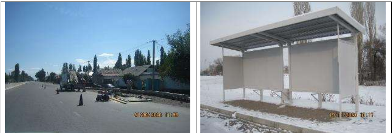
Figure 12 Construction of bus stops
