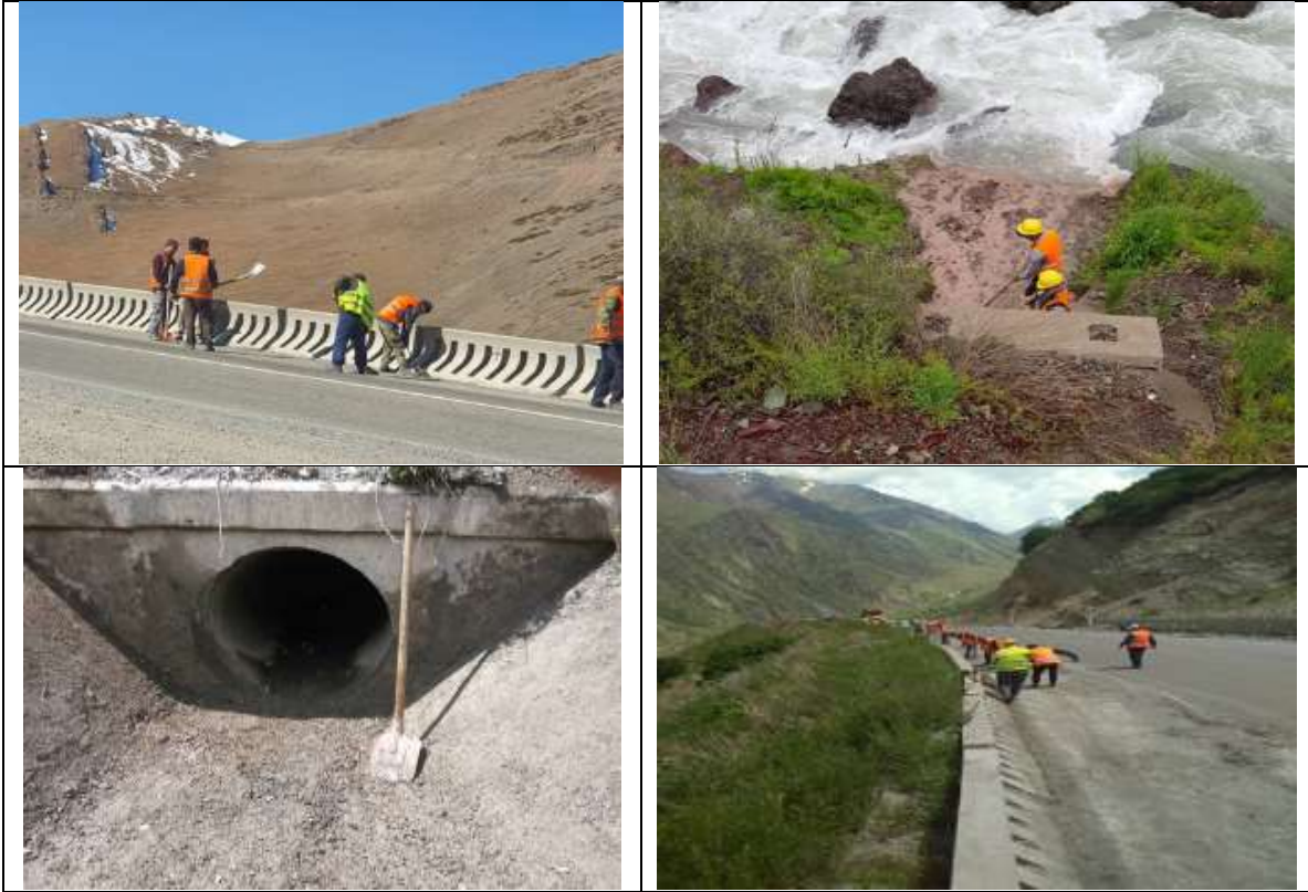
Figure-6. Culvert cleaning along parapets
