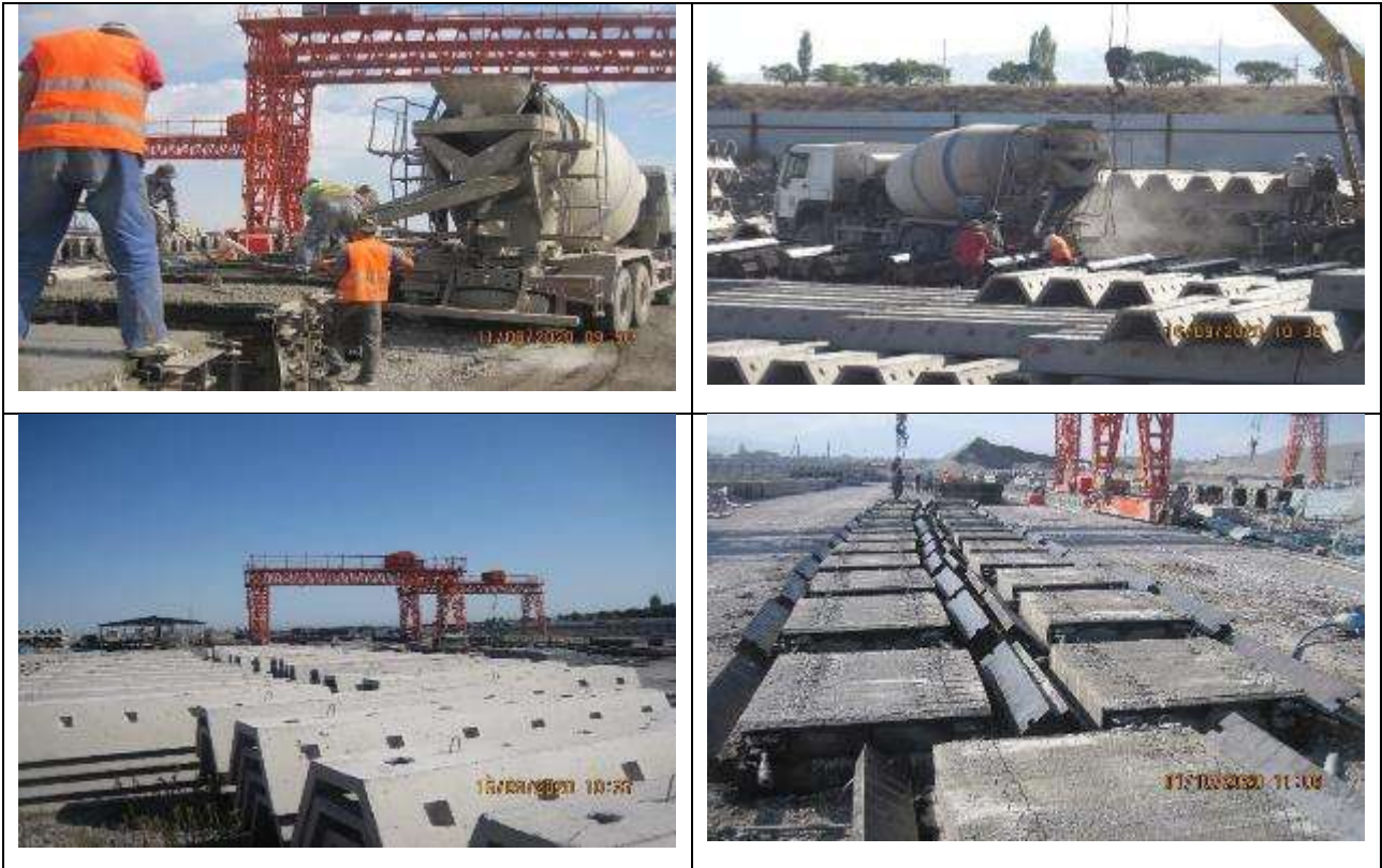
Figure 16 Production of reinforced concrete structures
