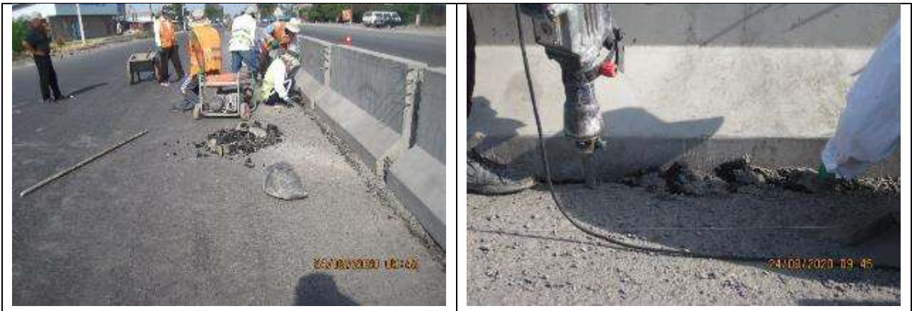
Figure 34 Cleaning of parapets from accumulated soil
