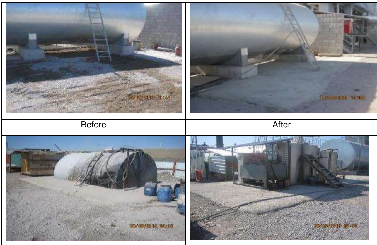
Figure 43 Impermeable protective coating around chemical containers
