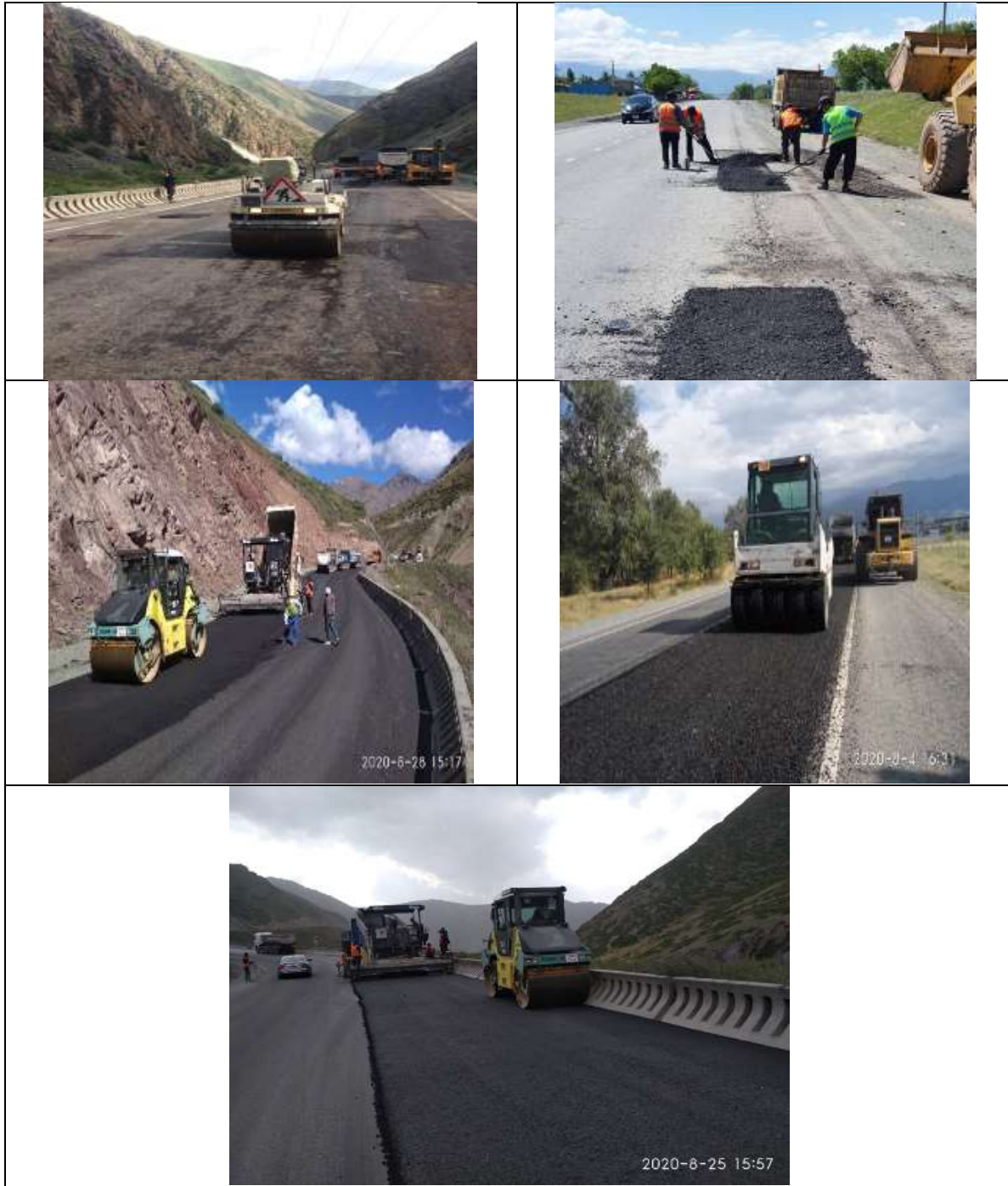
Figure-5. Current pavement repair.
