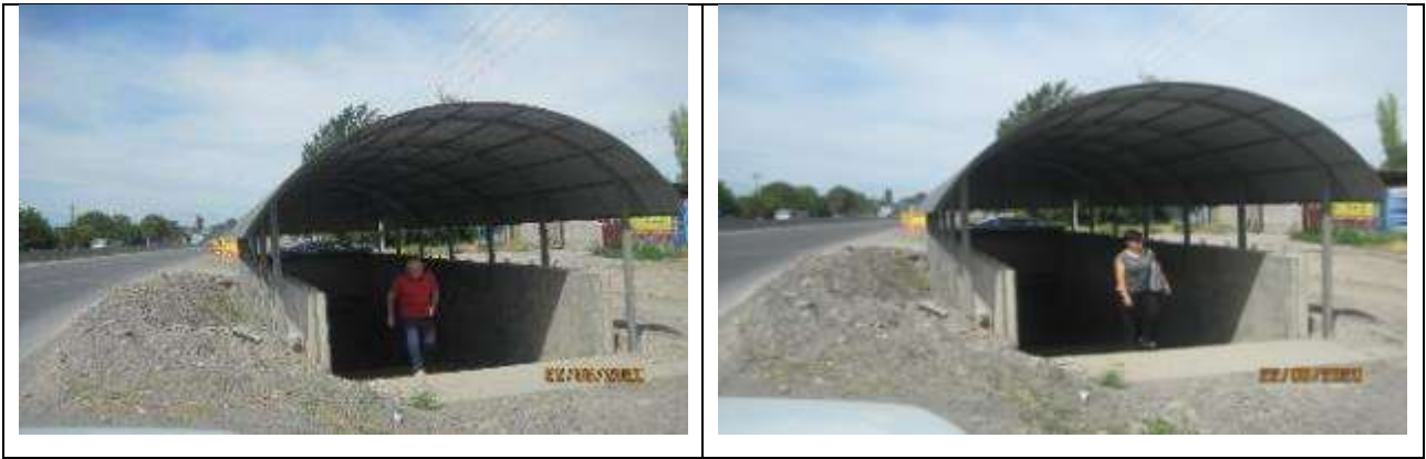
Figure 11 Construction and rehabilitation of underground passages
