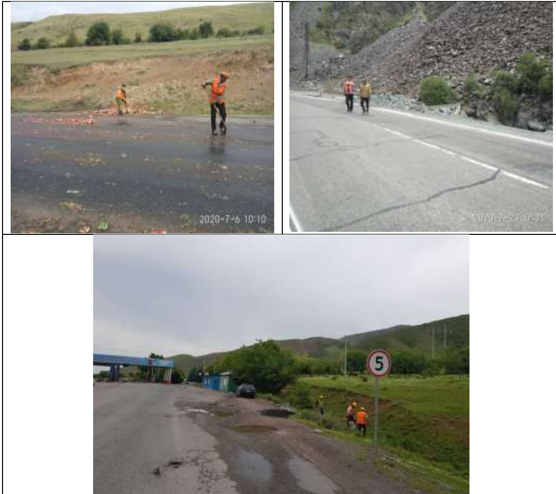
Figure-4. Cleaning roads from rubbish and rockfalls
