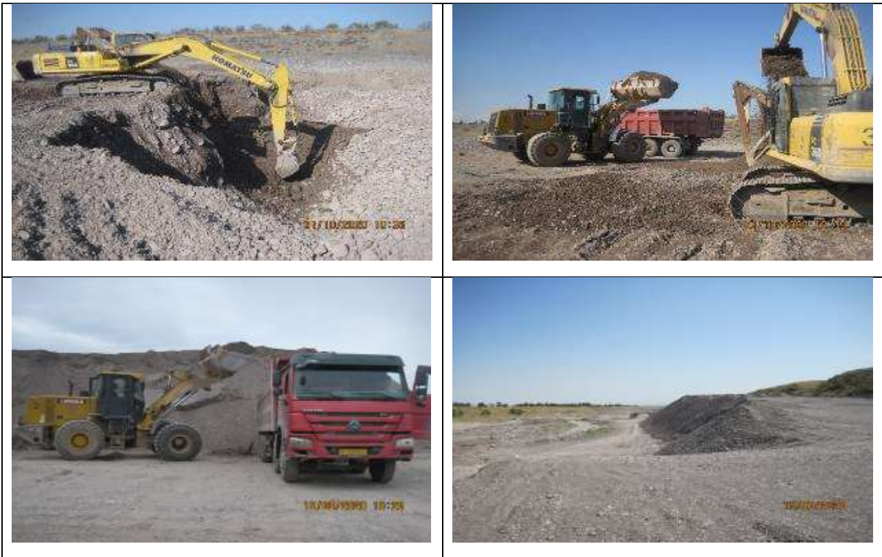
Figure 15 Development of Ak-Suu 2 borrow pit
