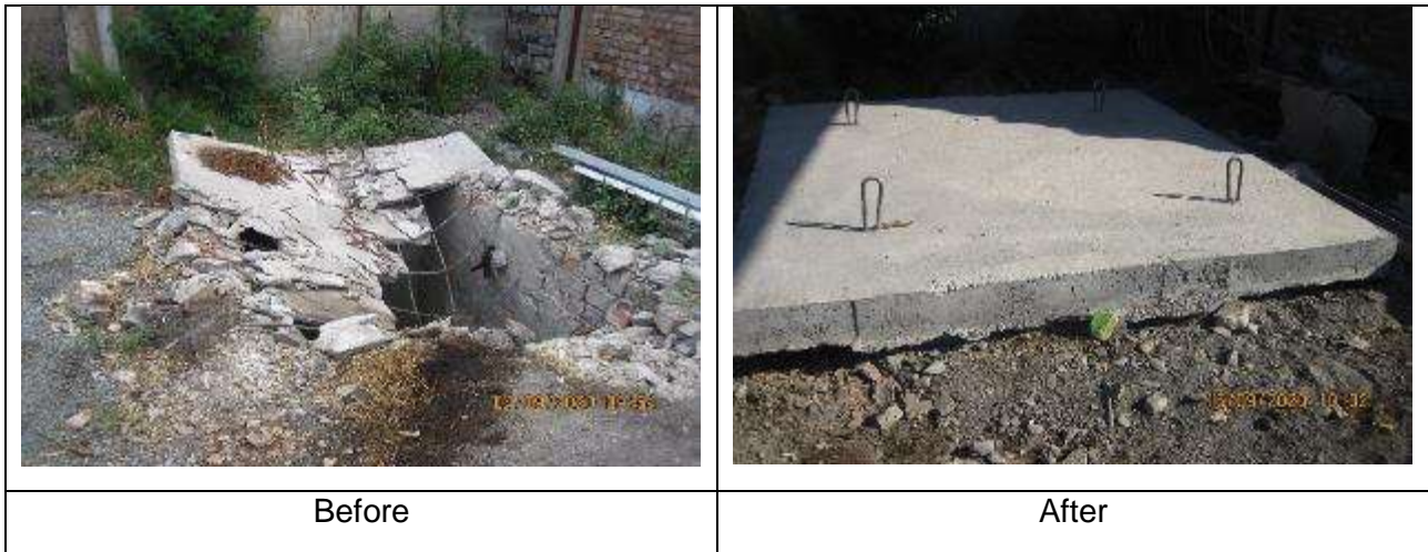
Figure 57 Top slab on the drain pit
