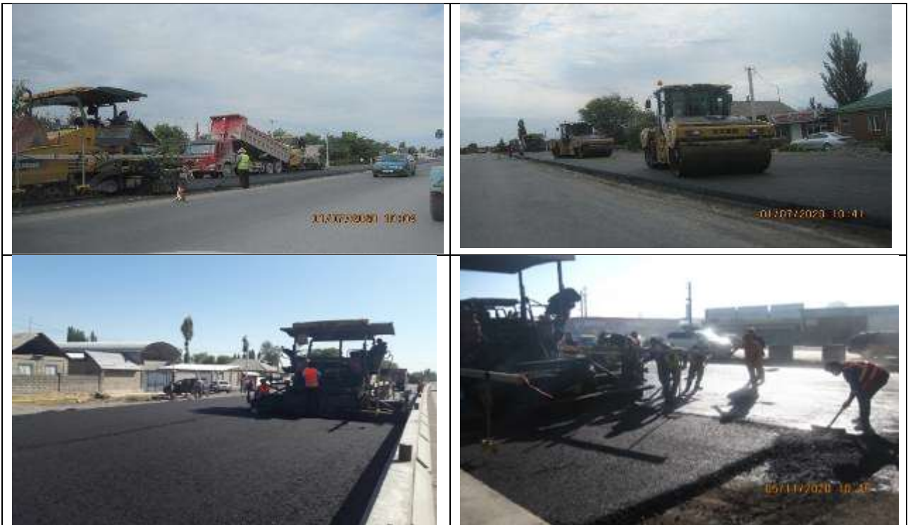
Figure 5 Asphalt laying
