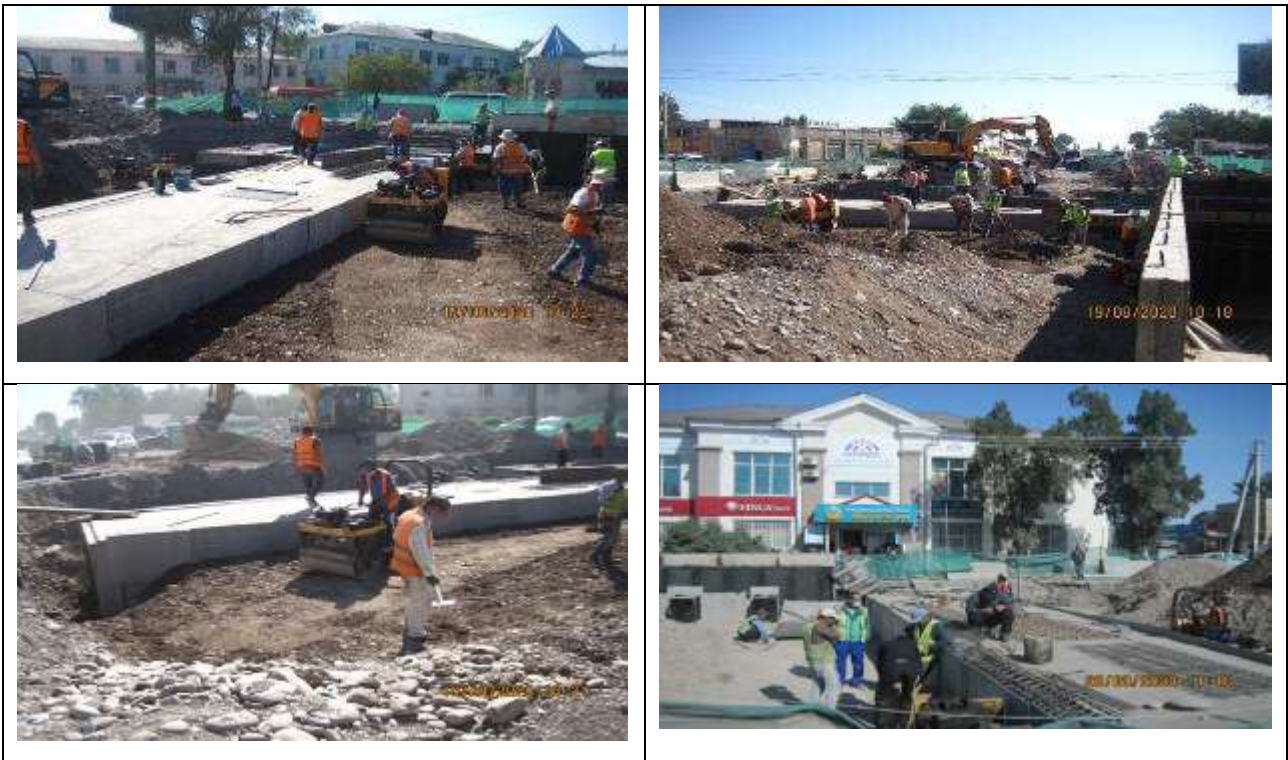
Figure 10 Construction of an underground passage in the village of Belovodskoye
