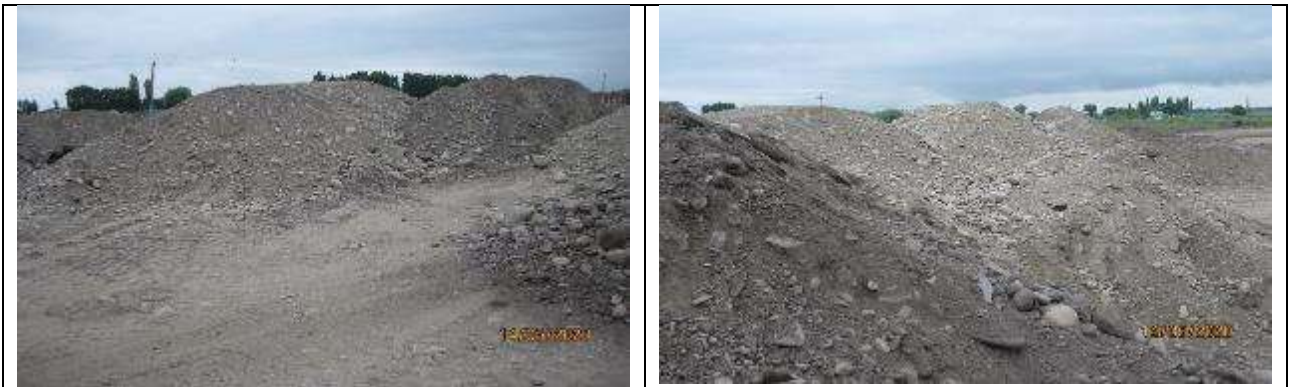
Figure 25 Storage of unsuitable soil for further use
