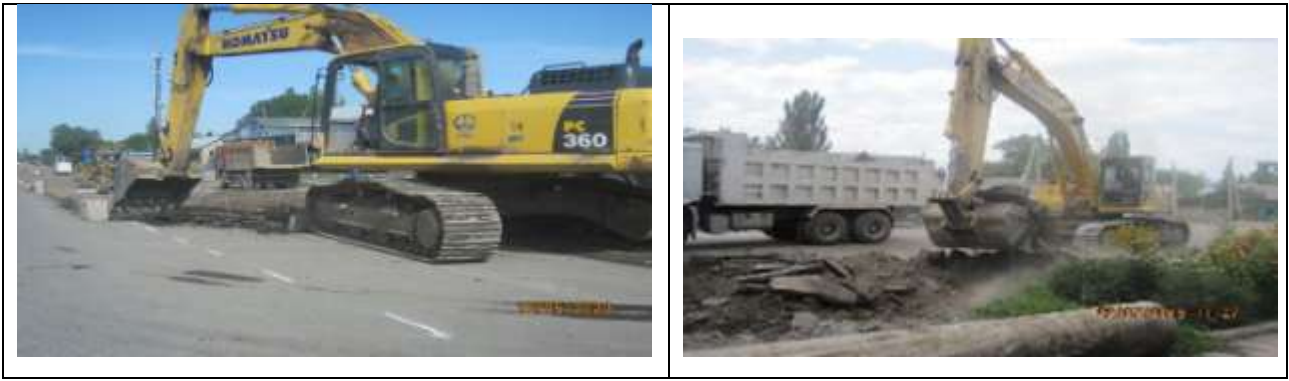
Figure 4 Removal of old asphalt and unsuitable soil
