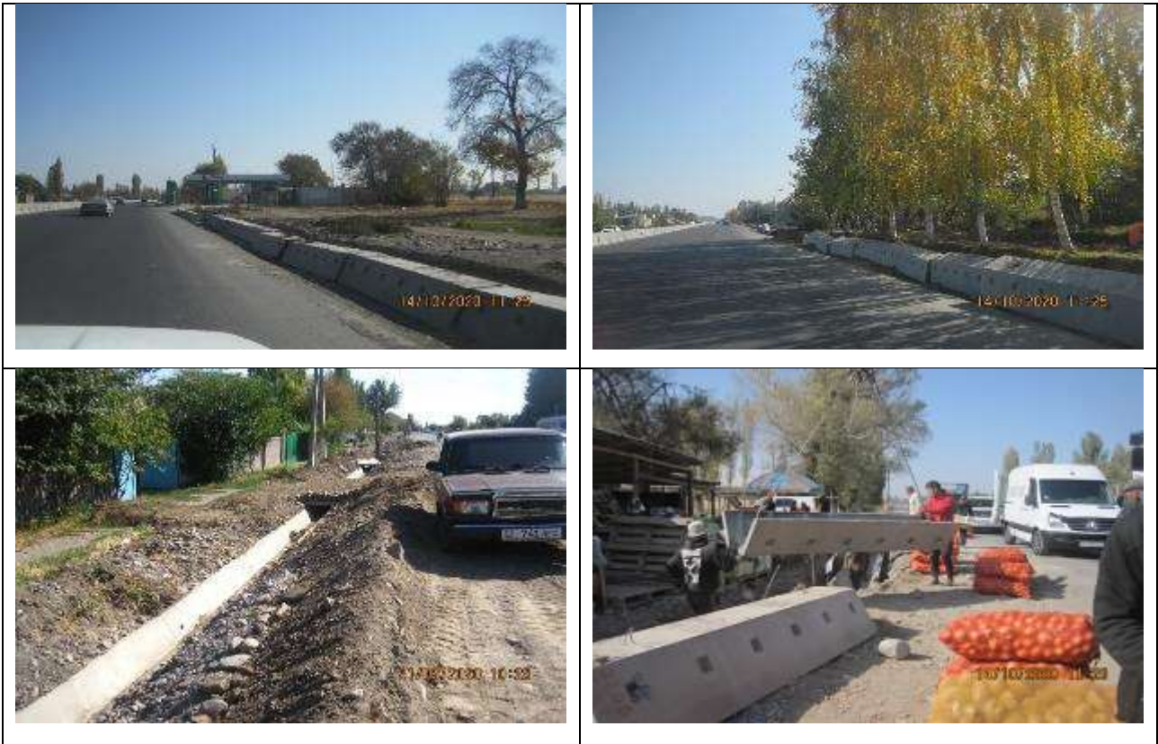
Figure 32 Installation of culvert chutes
