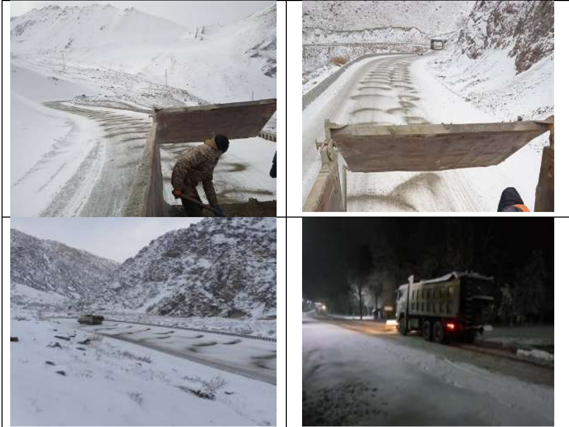
Figure-3. Sand bedding of the road
