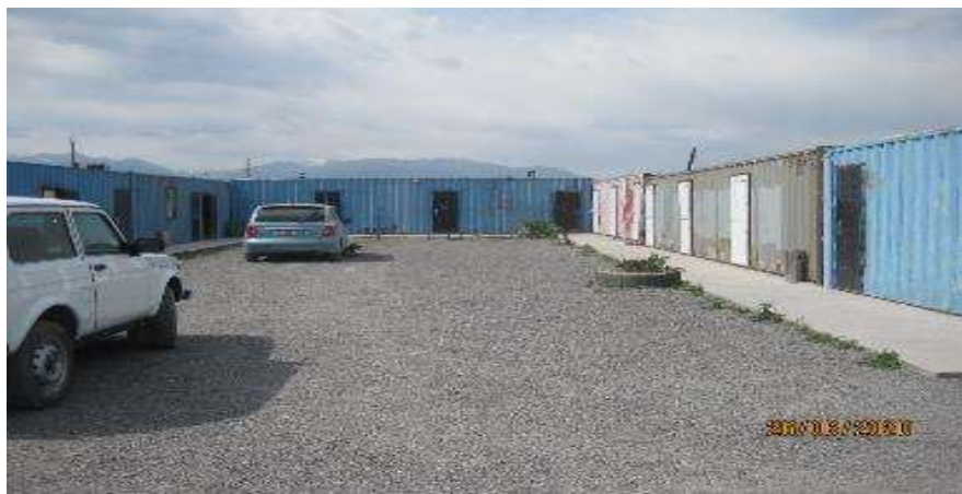
Figure 21 Workers ' accommodation camp on the territory of the production site
