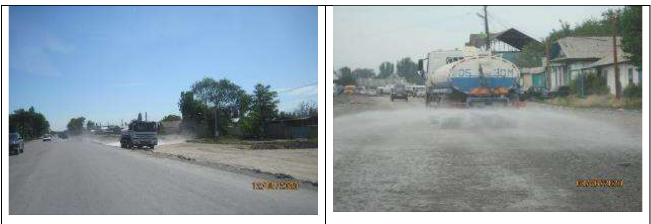
Figure 13 Water-sprinkling of the road to avoid dusting.
