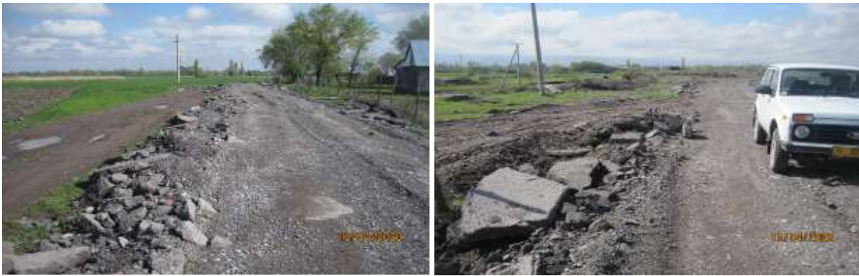
Figure 50 Removal of old asphalt to the streets of the village of Belovodskoe at the request of residents and local administration
