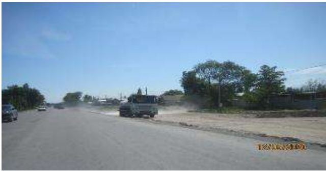
Figure 7 Water sprinkling at the road
