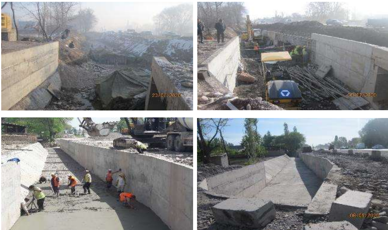
Figure 10 Bridge construction at the Jantai canal
