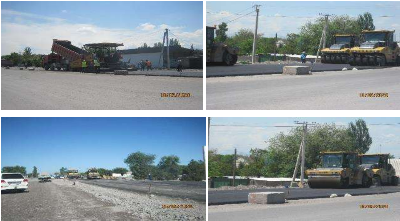
Figure 5 Asphalt laying
