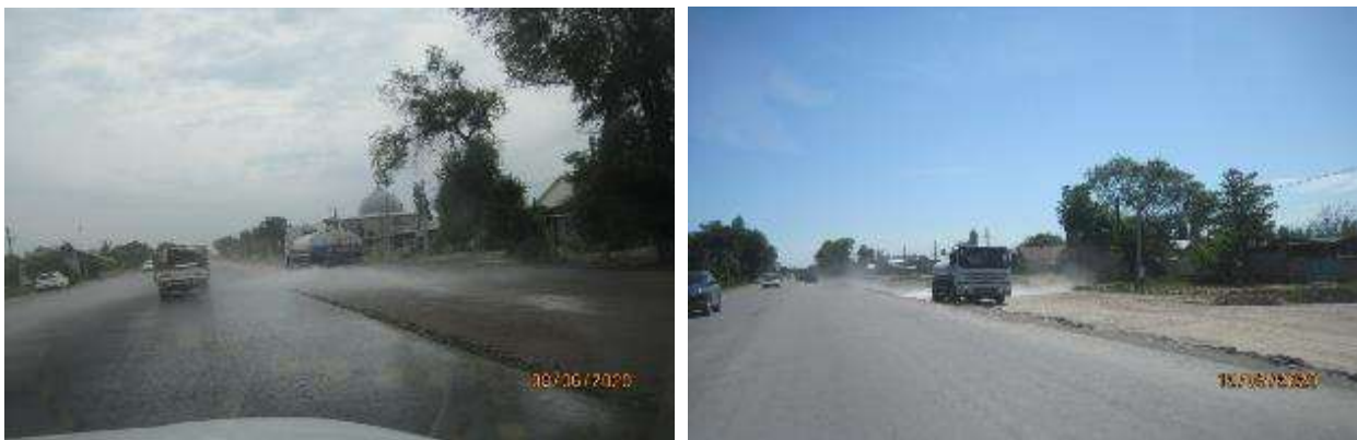
Figure 28 Water sprinkling at the road construction sites
