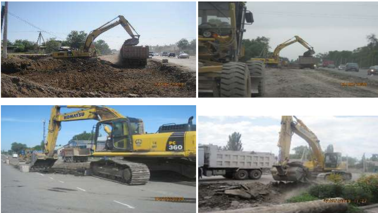
Figure 4 Removal of old asphalt and unsuitable soil
