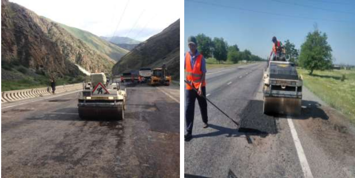
Figure-5. Current pavement repair
