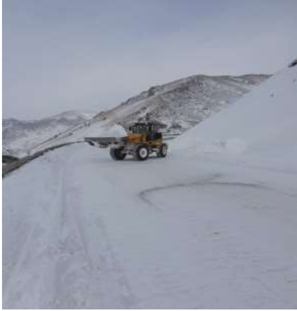
Figure-2. Winter road surface cleaning - Filling the road with sand (mechanical and manual) 61-129.5 km.
