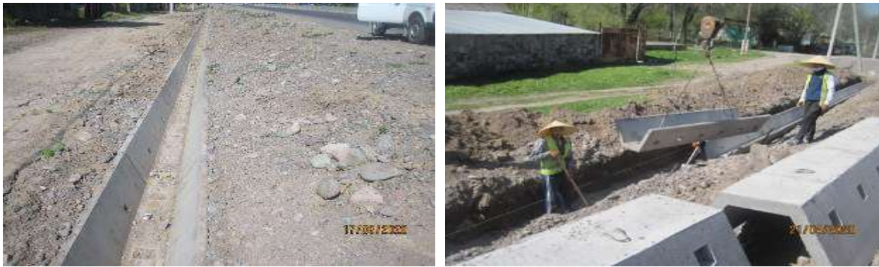
Figure 29 Construction of culvert chutes
