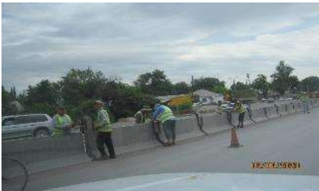
Figure 8 Installation of “New Jersey” type median parapets
