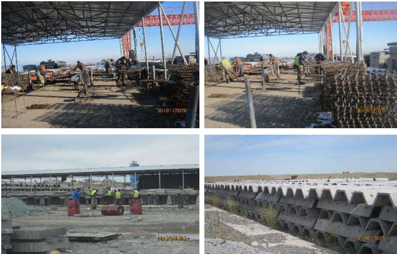
Figure 15 Site for production of reinforced concrete products
