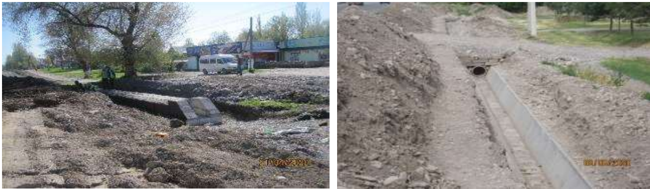
Figure 9 Construction of culvert chutes
