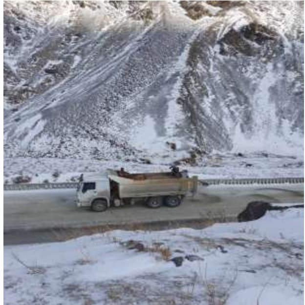
Figure-2. Winter road surface cleaning - Filling the road with sand (mechanical and manual) 61-129.5 km.
