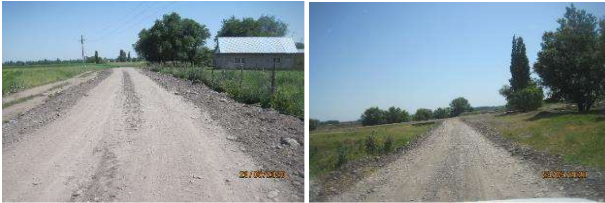
Figure 63 Kalinina street after levelling
