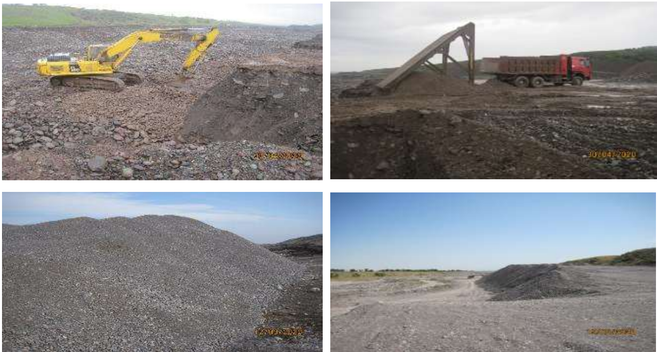
Figure 12 Works at Ak-Suu 2 borrow-pit
