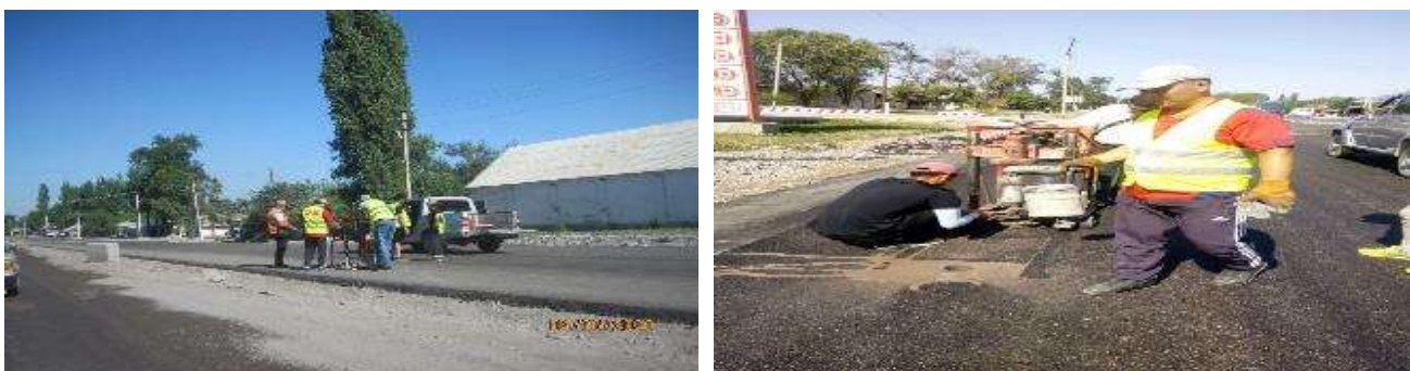
Figure 6 Sampling for asphalt quality control
