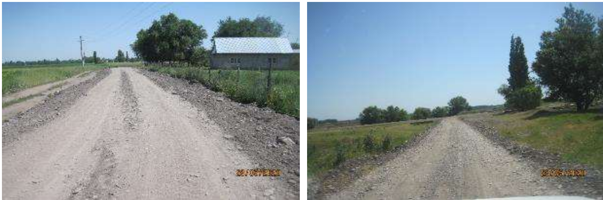
Figure 51 Kalinina street after levelling
