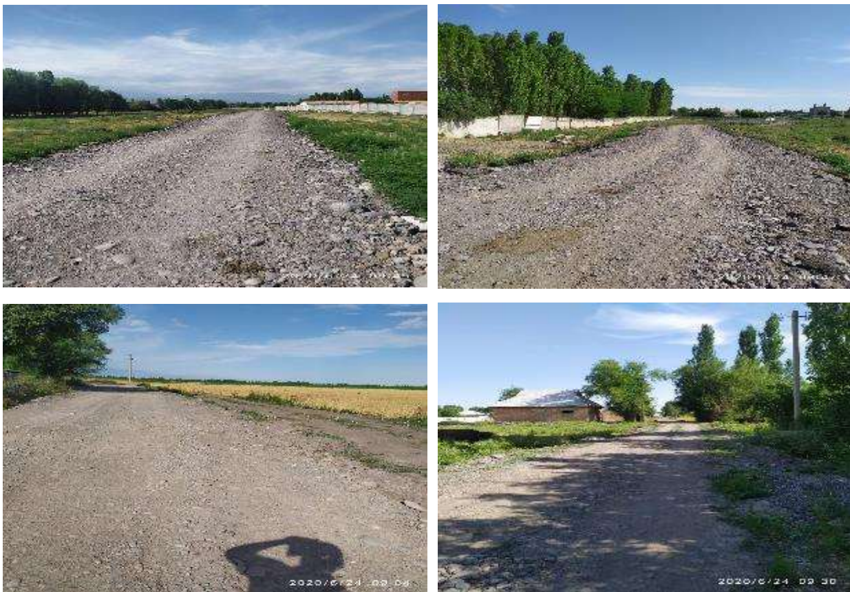
Figure 64 Removal of old asphalt to the territory of sections 5 and 6
