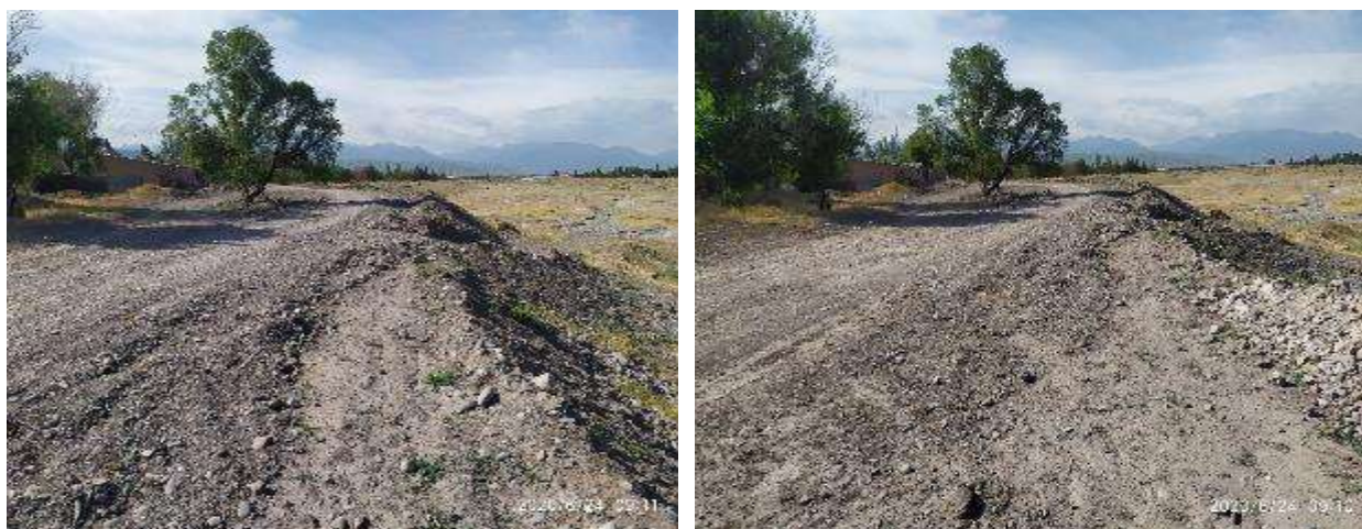
Figure 65 Taken out of unsuitable soil to the area of sections 5 and 6
