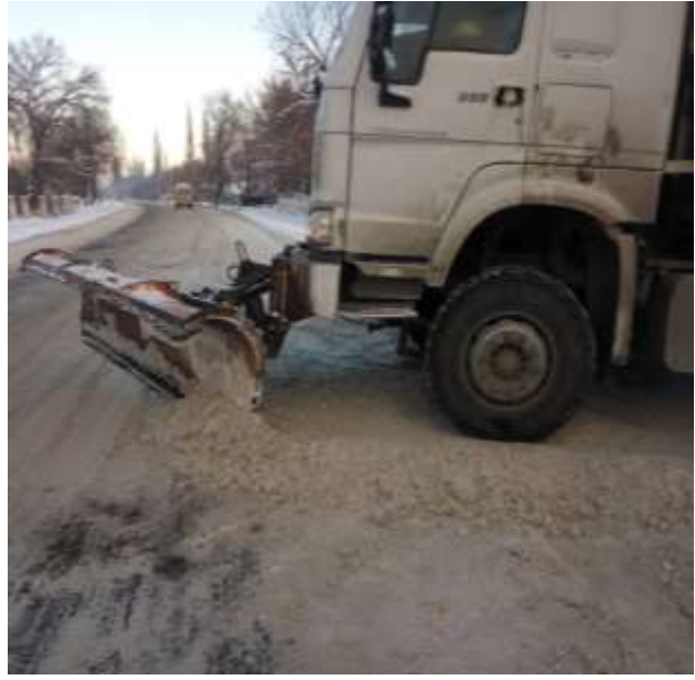
Figure-2. Winter road surface cleaning - Filling the road with sand (mechanical and manual) 61-129.5 km.
