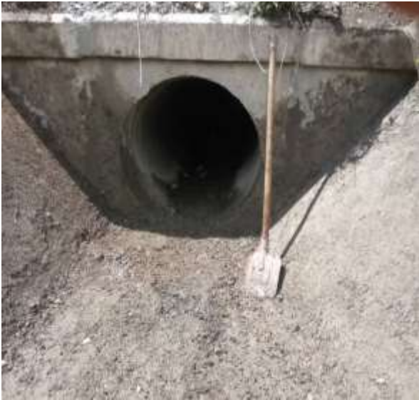
Figure-6. Culvert cleaning along parapets
