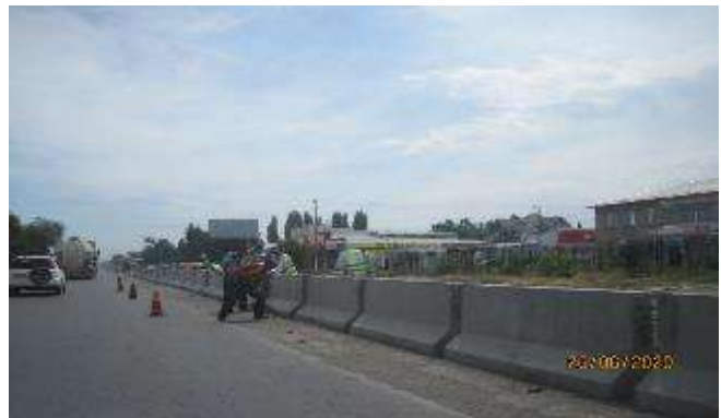
Figure 8 Installation of “New Jersey” type median parapets
