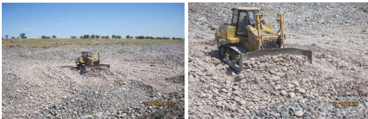
Figure 37 Reclamation works at the Ak-Suu 2 borrow-pit
