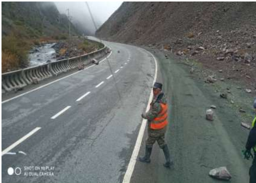
Figure-4. Cleaning roads from rubbish and rockfalls
