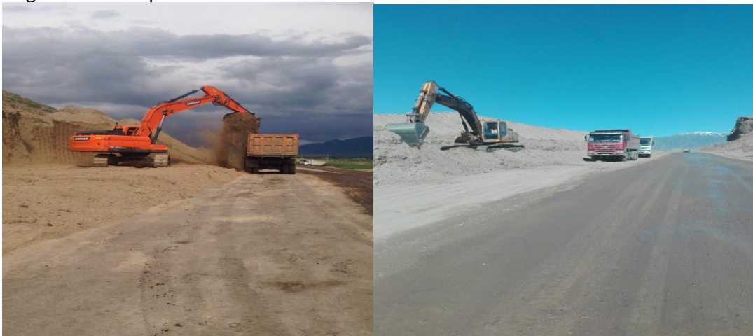
Figure 4. Excess soil removal
