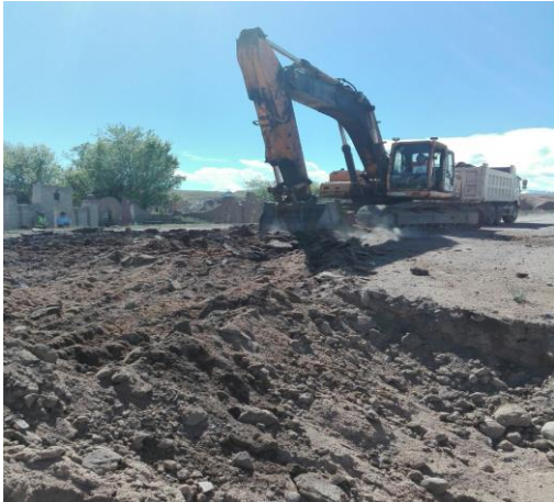
Figure 3 Old asphalt removal
