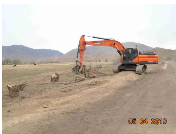
Figure 6 Grubbing the trees' root.
