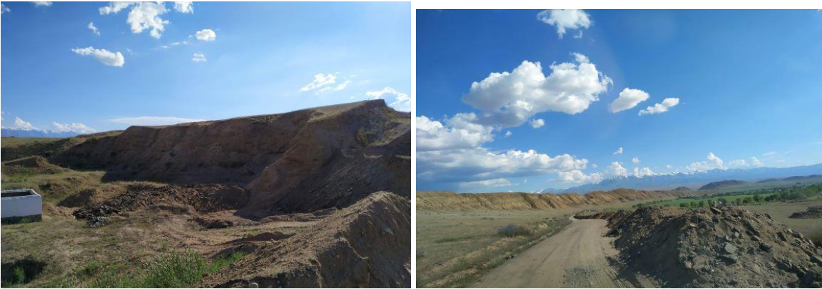
Figure 7. Taking out of old asphalt for backfilling of rural streets
