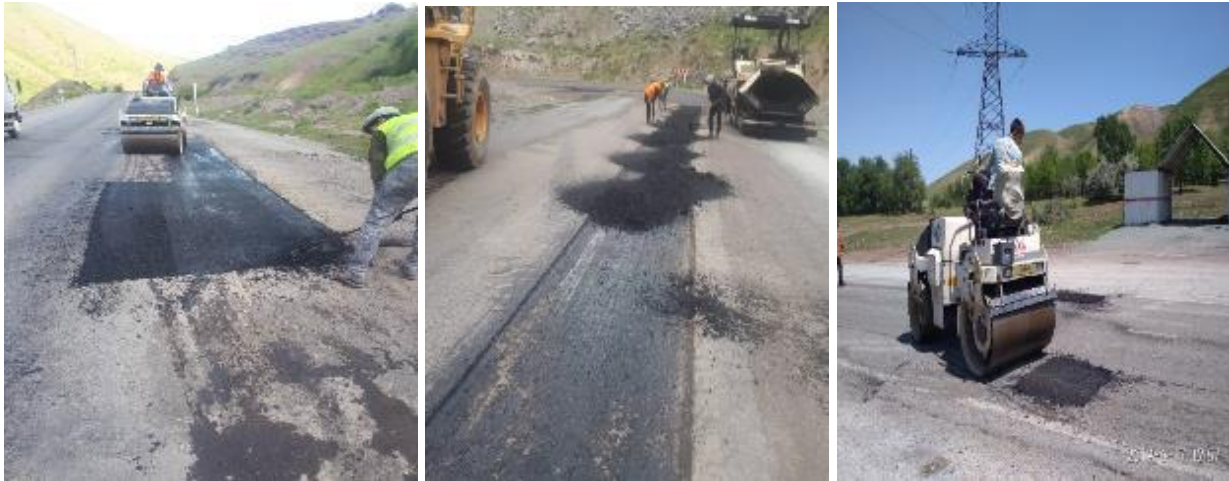
Figure - 5. Current repairs of the pavement
