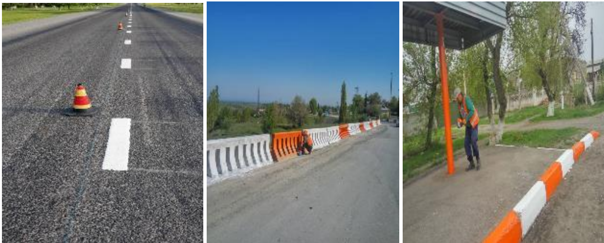
Figure - 8. Road marking
