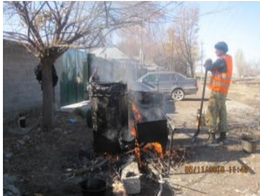
Figure 27. Burning bitumen to heat bitumen during the waterproofing of culverts
