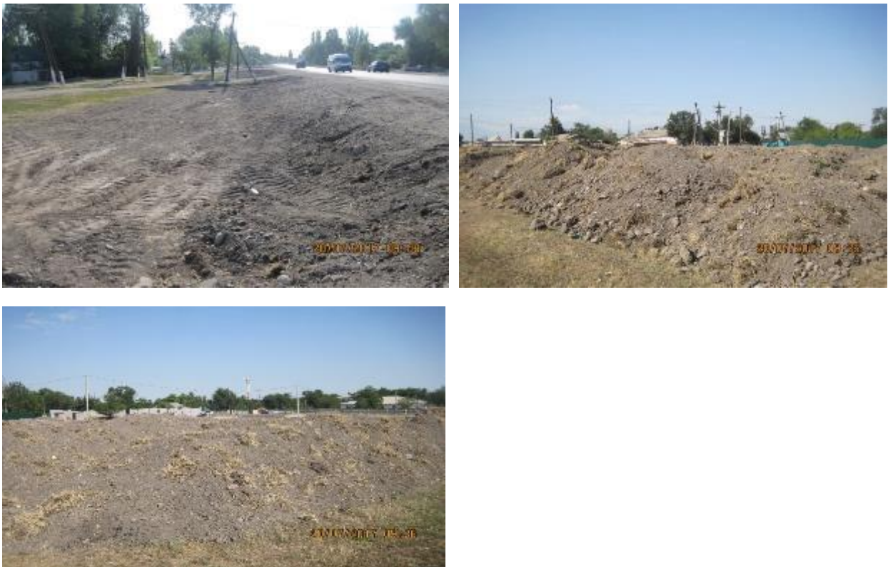
Figure 18. Topsoil Placement and Storage along the Alignment
