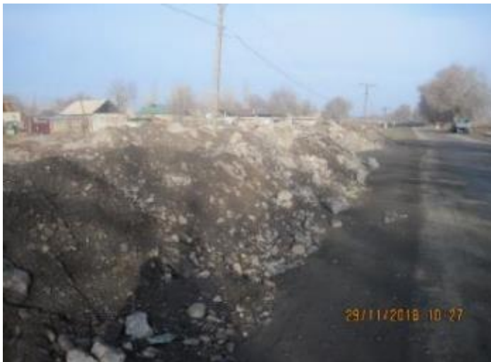
Figure 300 Construction waste at the northern side of the bridge under construction
