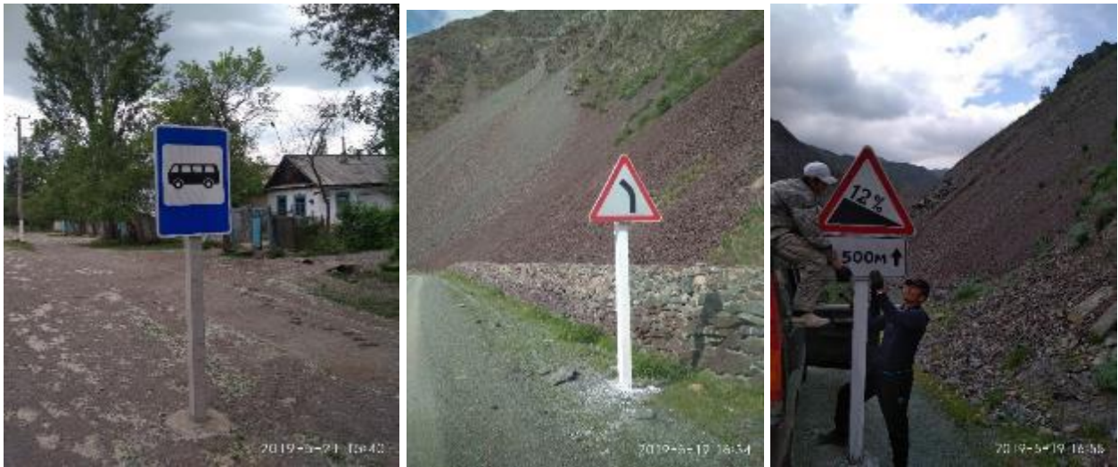
Figure 7 Installing road signs
