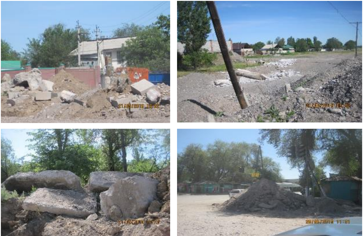
Figure 11. Examples of construction debris along roadside
