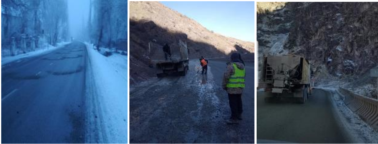
Figure-3. Filling road with sand
