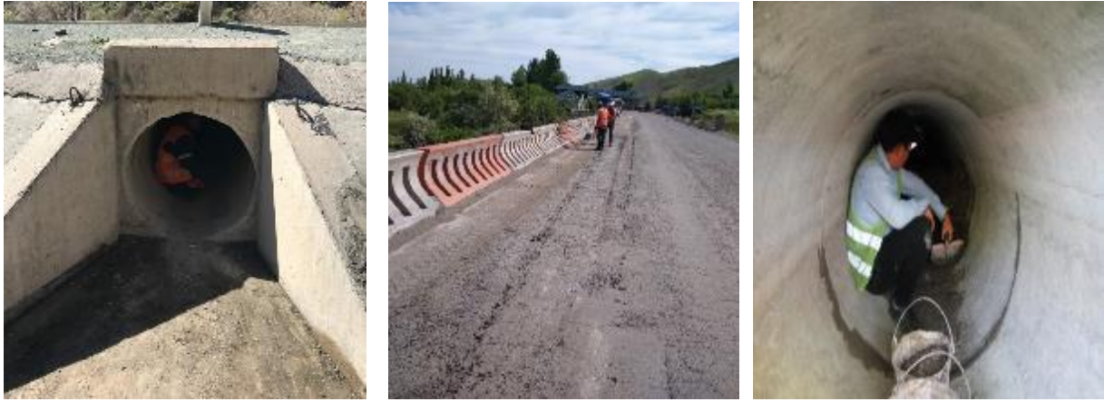
Figure - 9. Cleaning culvret pipes
