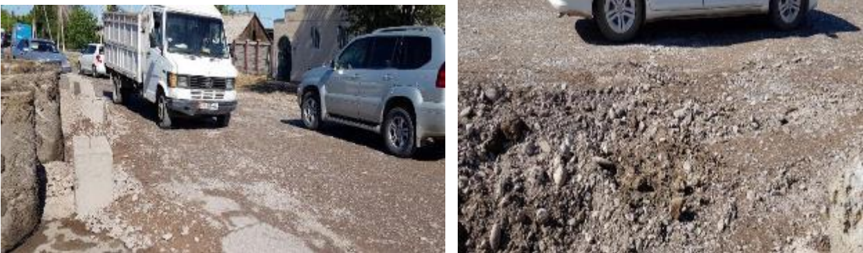
Figure 19. Alexandrovka construction waste blocking road
