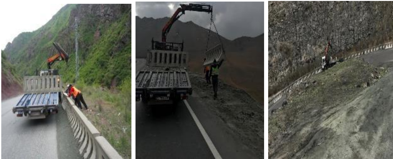
Figure 6 - Installing parapets BB-3. Unsuitables were replaced
