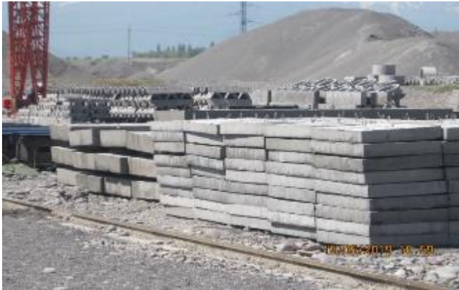
Figure 13. Concrete prefabrication yard.
