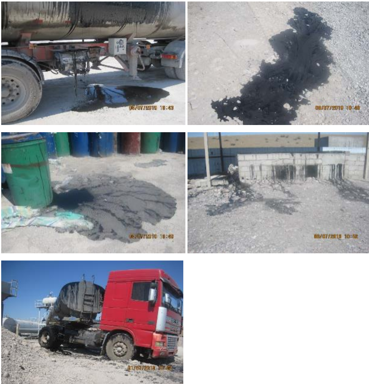
Figure 44 Bitumen leakages at the asphalt plant
