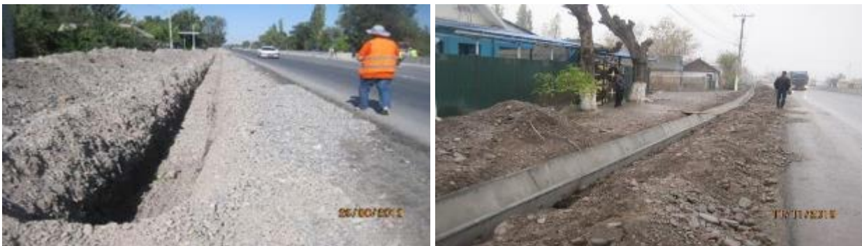
Figure 7 Installation of culvert chutes
