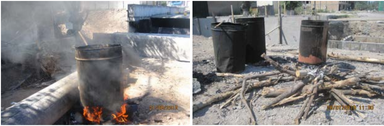
Figure 27 Melting of bitumen during waterproofing works
