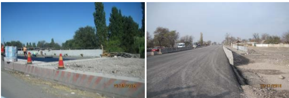
Figure 11 Construction of Sokuluk bridge
