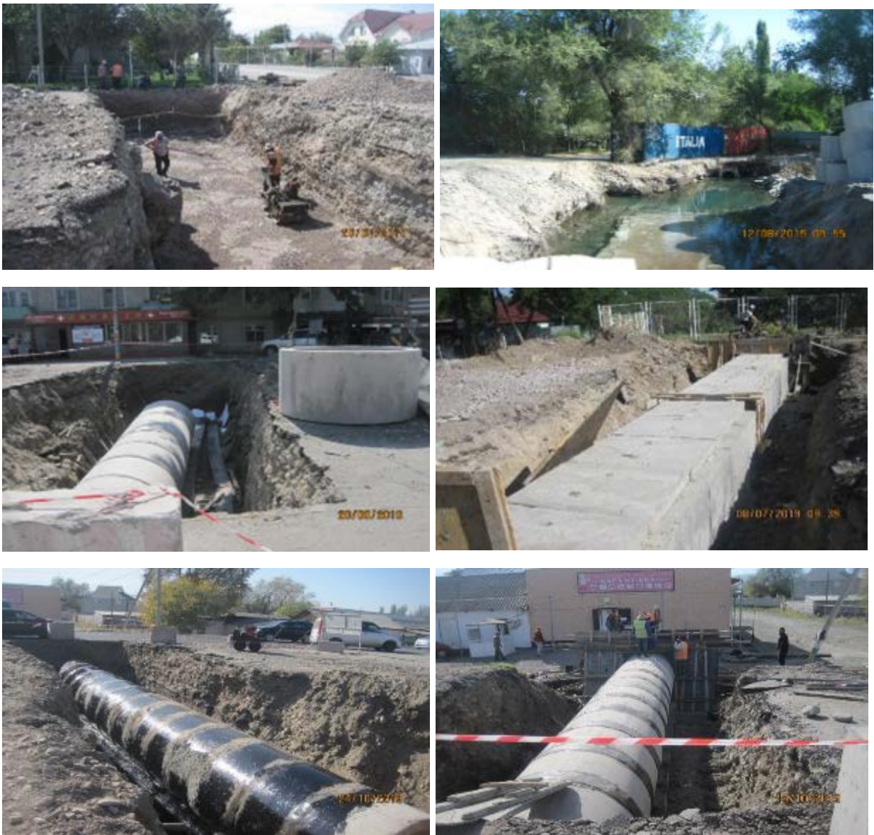
Figure 15 Construction of culvert pipes
