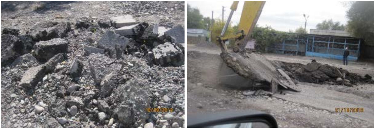
Figure 49 Old asphalt removal
