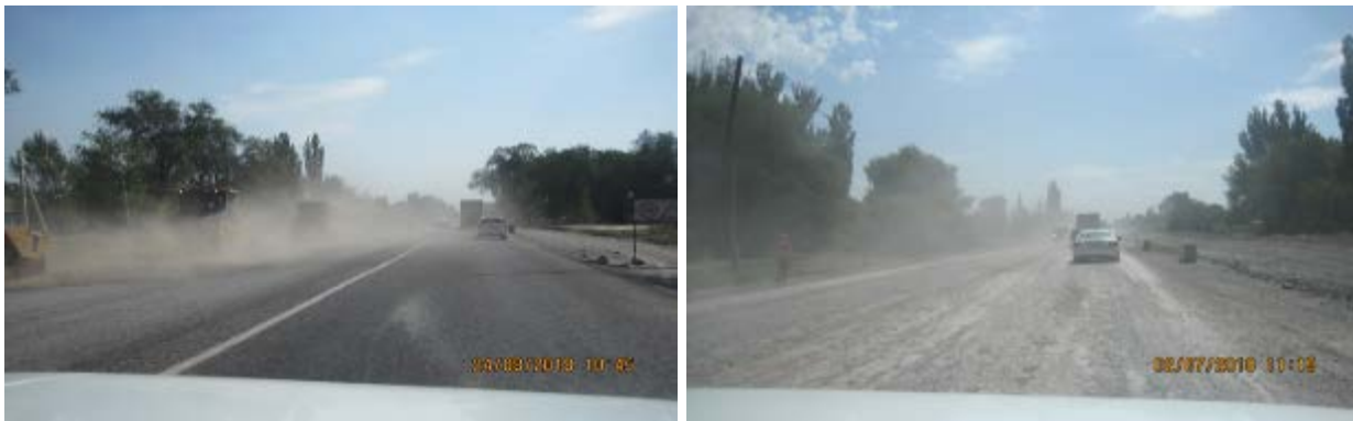
Figure 26 Increased dust generation at construction sites
