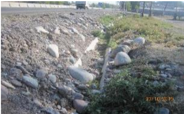
Figure 32 The state of constructed chutes
