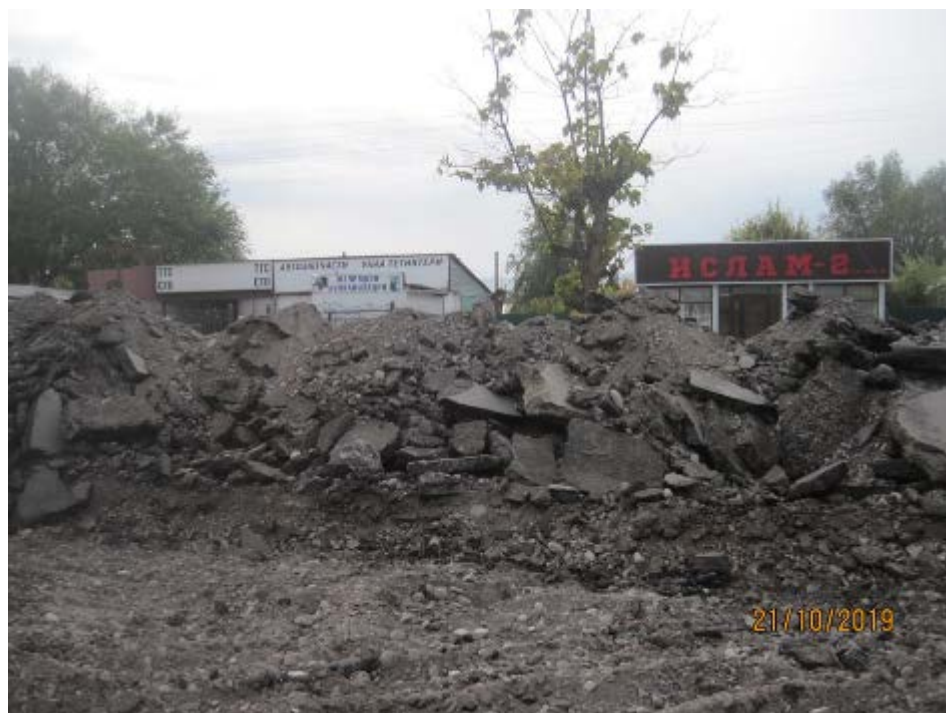
Figure 63 Old asphalt removed from the roadbed
