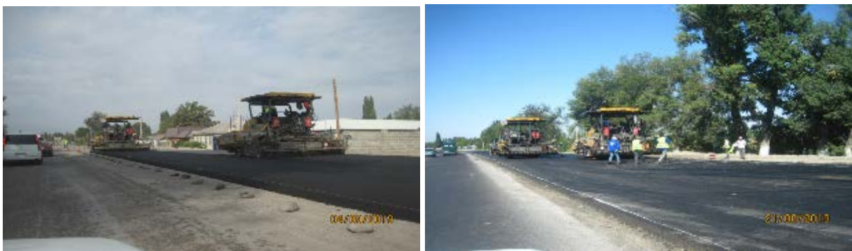
Figure 4 Lying of asphalt
