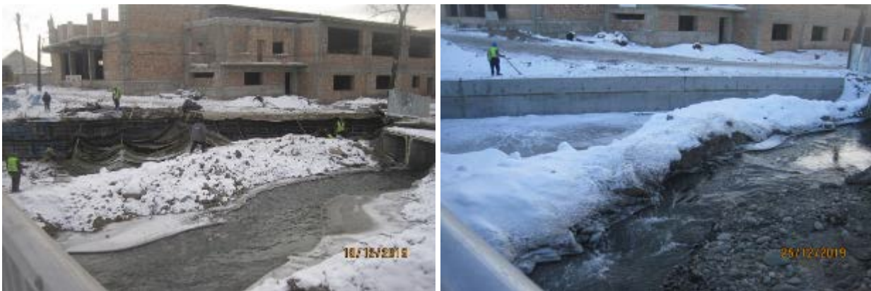
Figure 40 Bank protection works at the Sokuluk river (south side)
