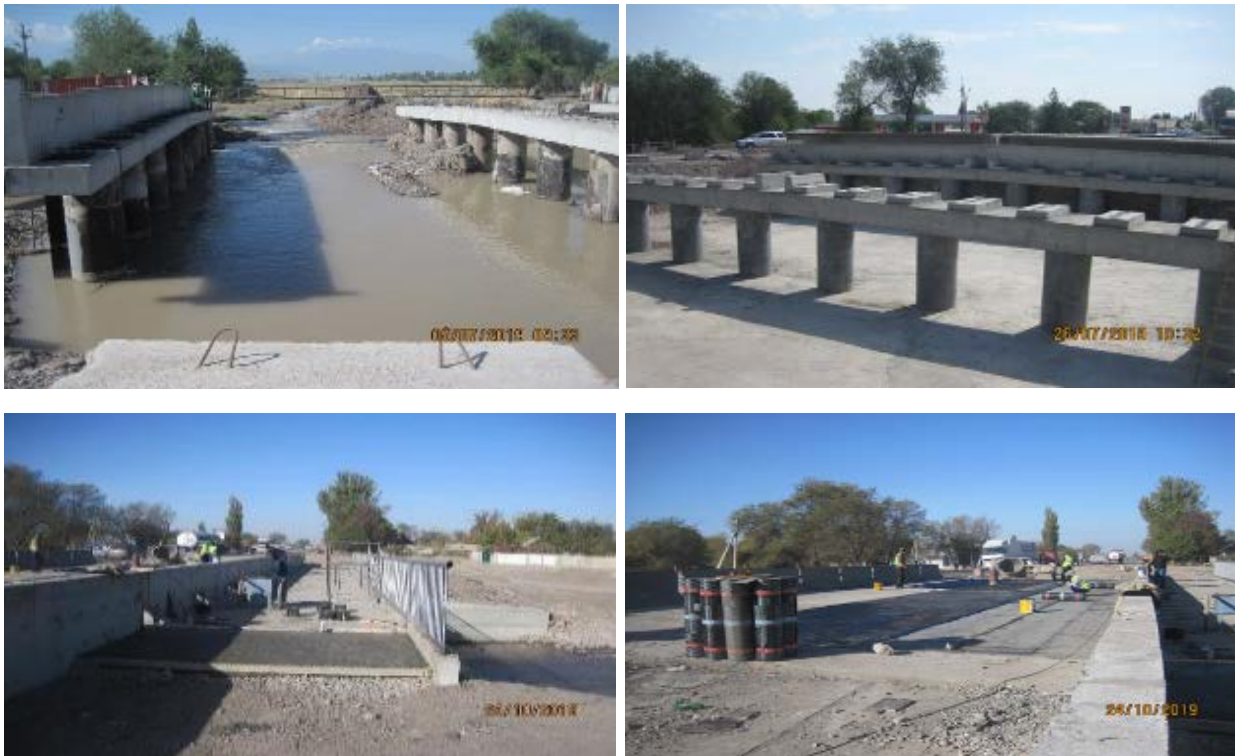
Figure 10 Construction of Ak-Suu bridge
