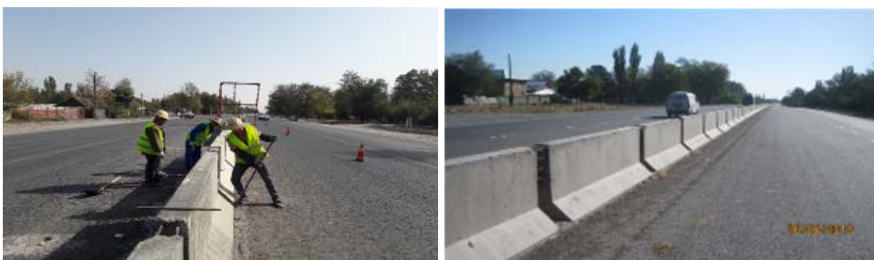
Figure 5 Construction of "New Jersey" type parapet fencing
