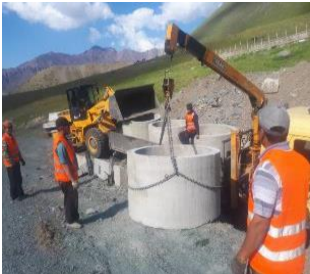
Figure – 6. Culvert replacement
