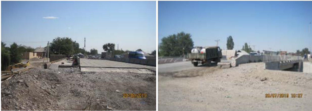
Figure 12 Bridge construction at the mudflow canal from the Ak-Suu River
