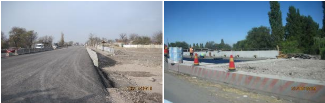
Figure 38 Construction of Sokuluk bridge
