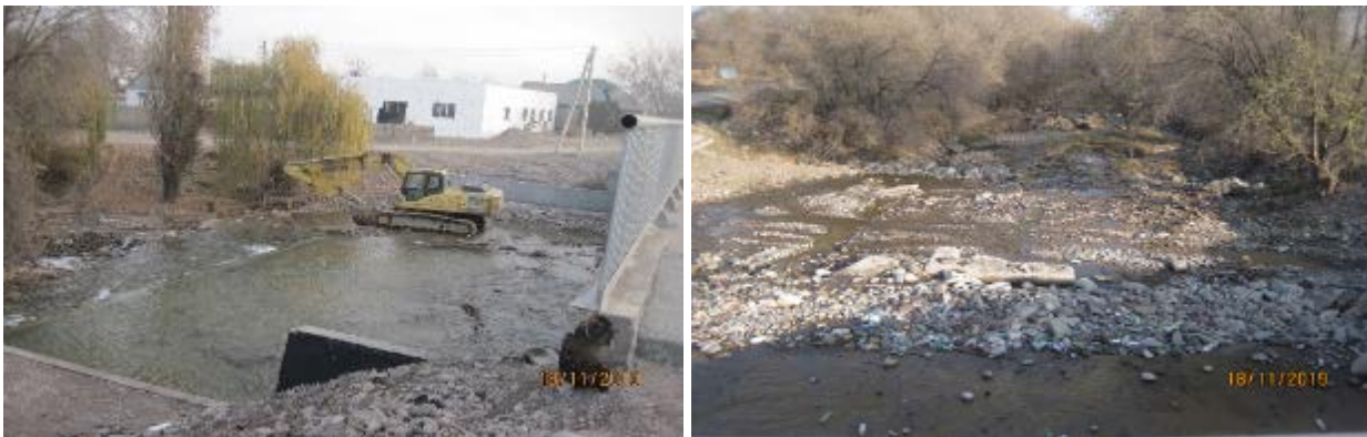
Figure 39 Cleaning the Sokuluk riverbed from construction waste (north side)
