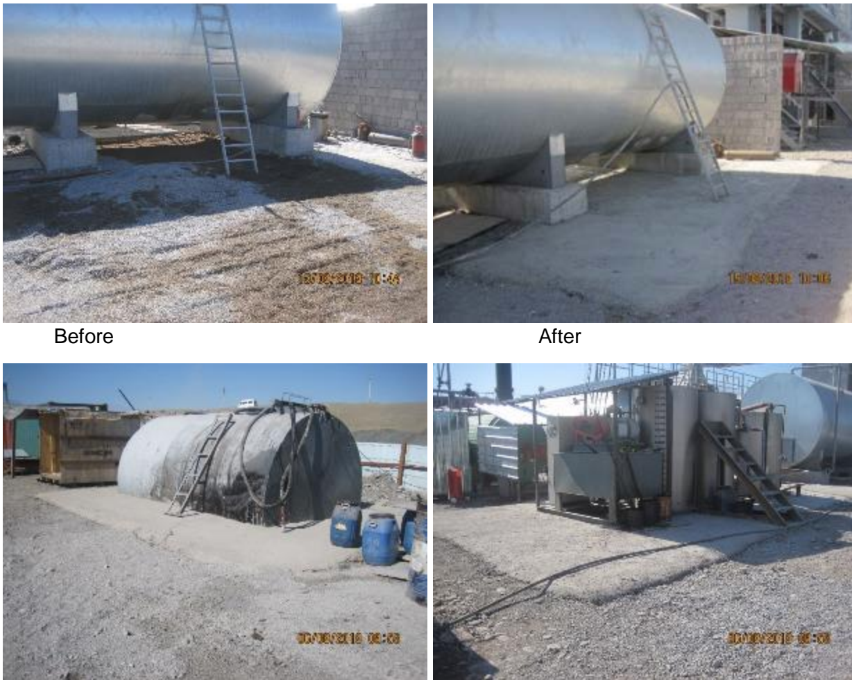
Figure 45 Impervious protective platform around the chemical storage containers
