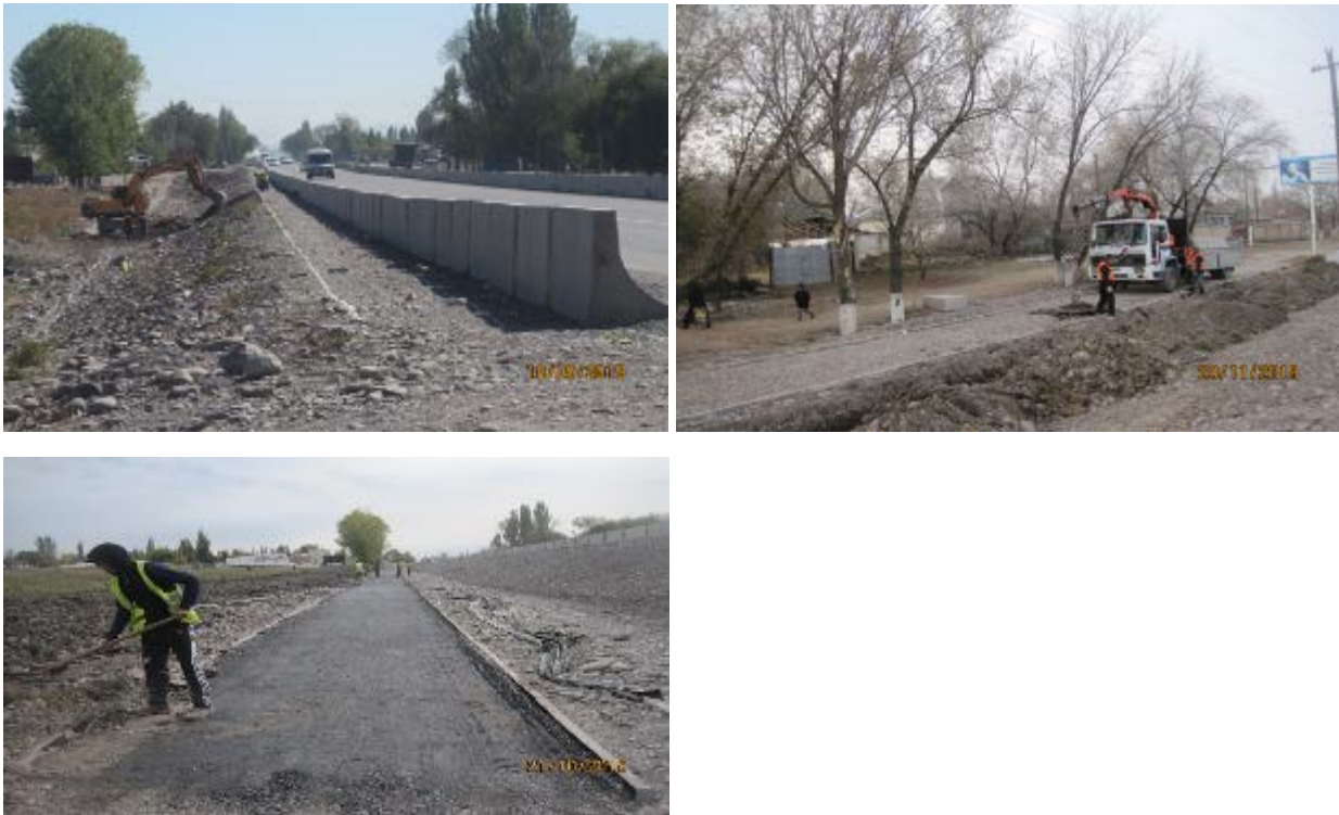
Figure 6 Construction of sidewalks
