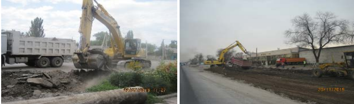
Figure 3 Removing of old asphalt and unsuitable soil
