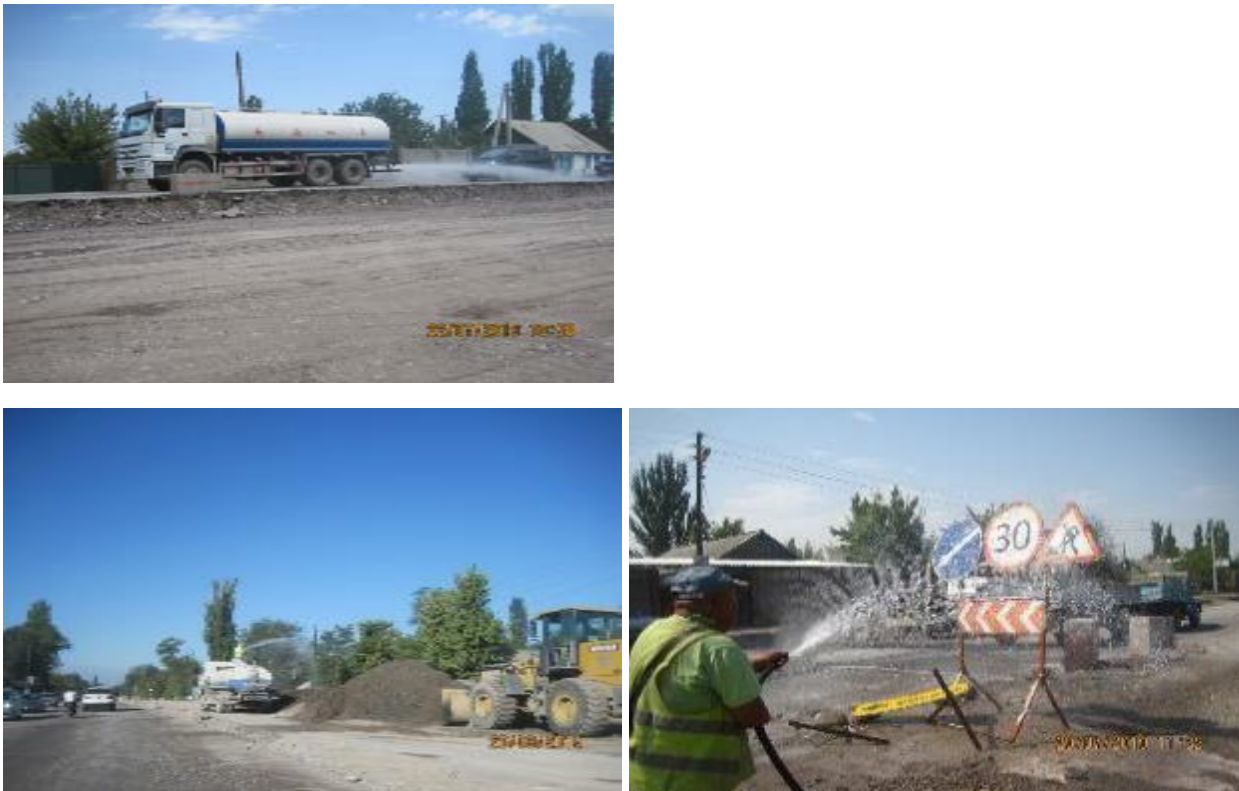
Figure 9 Road water sprinkling
