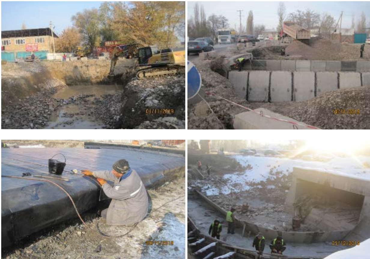
Figure 36 Construction of Jantai bridge
