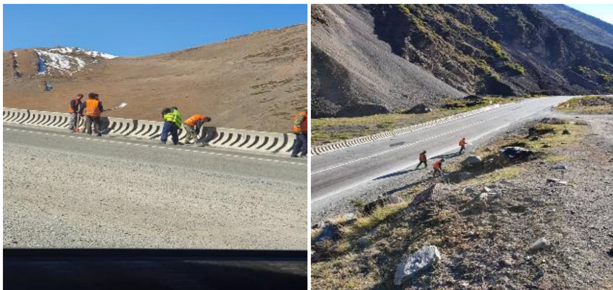
Figure-4. Cleaning roads from rubbish and rockfalls
