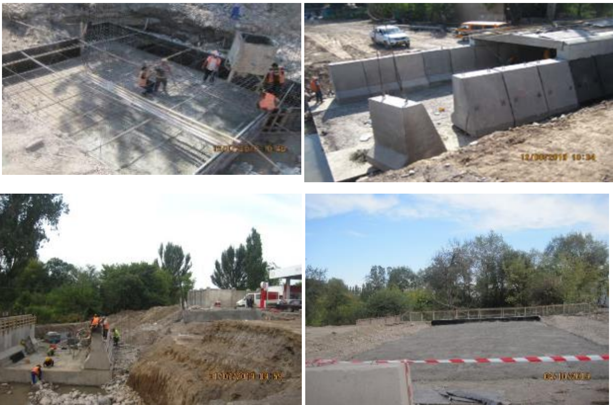
Figure 13 Bridge construction at Krepostnoy canal
