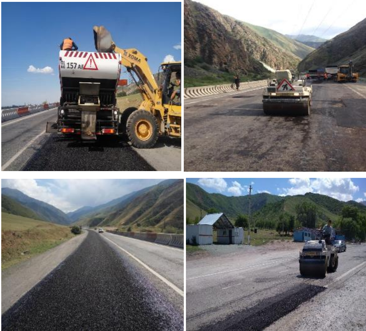
Figure-5. Current pavement repair
