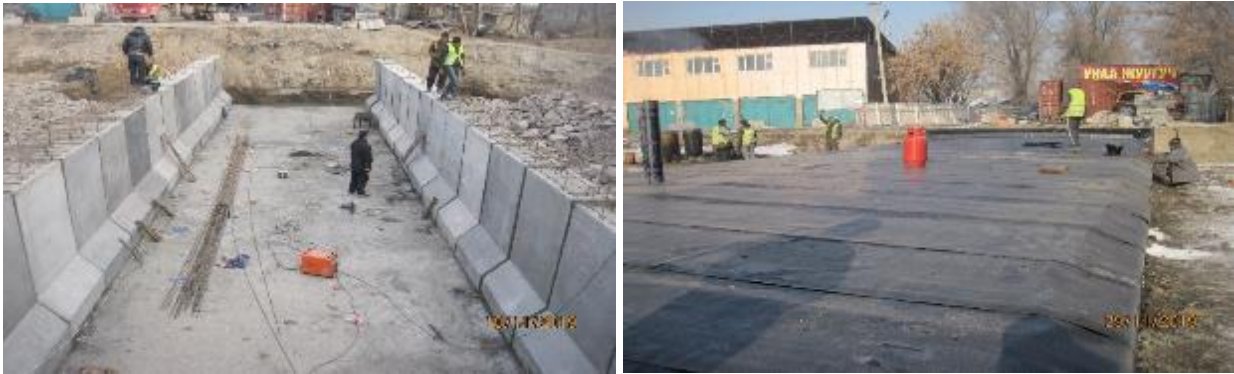
Figure 14 Brdige construction at Jantai canal
