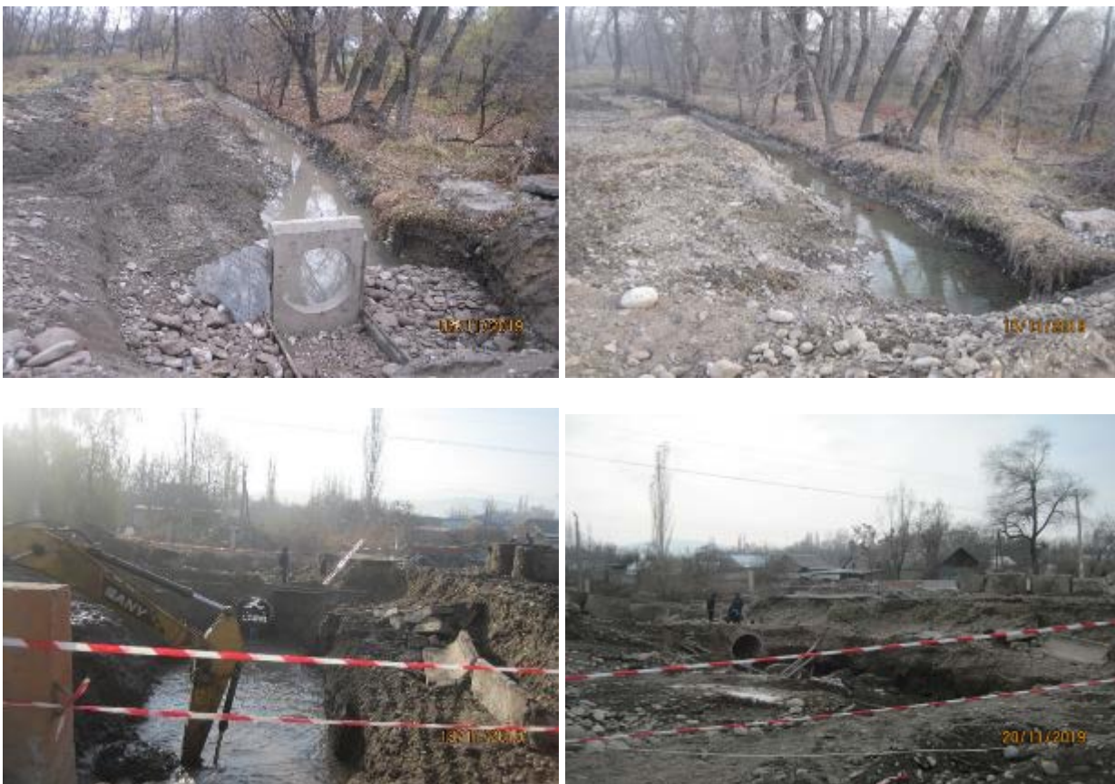
Figure 30 Ground water outcropping during the construction of culverts
