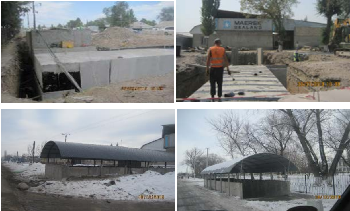
Figure 8 Construction and rehabilitation of underground crossings
