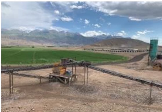
Photo 97 Lot 2. Poured technological earthen road to crusher plant Km 81 + 200.
