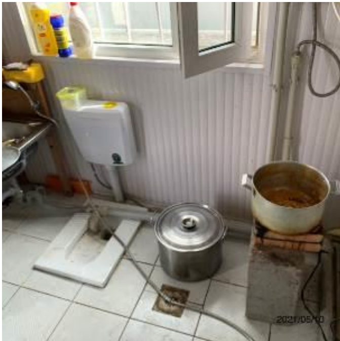
Photo 76. Lot 2. The bathroom transformed into kitchen.
