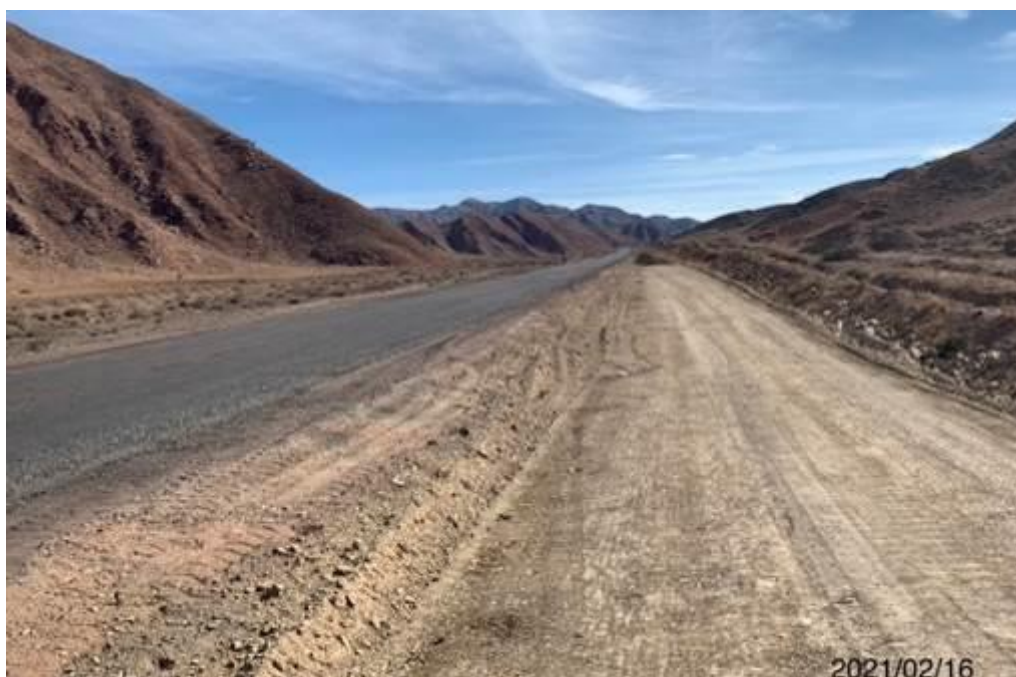
Photo 14. Road widening at km 14+050 – 16+500: after clearing and grubbing.
