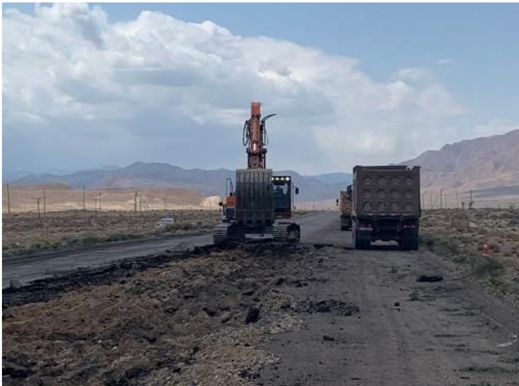
Photo 20. Lot 1. Removal and disposal of old asphalt concrete at km 4 + 800.
