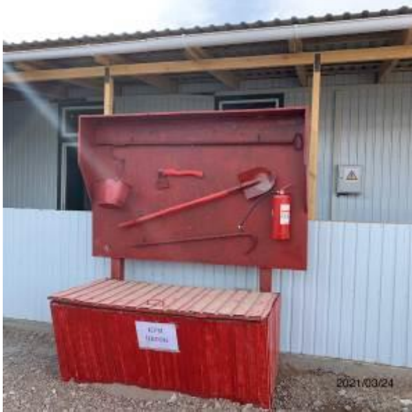
Photo 91. Lot 1 Shield with fire-fighting equipment.
