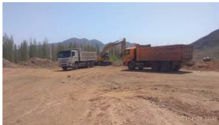
Photo 59. Lot 1. Work on the removal of waste from the old asphalt concrete from spoil bank at km. 12 + 000.
