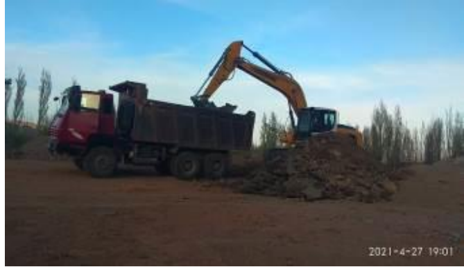
Photo 58. Lot 1. Removal of waste of old asphalt on a concrete.
