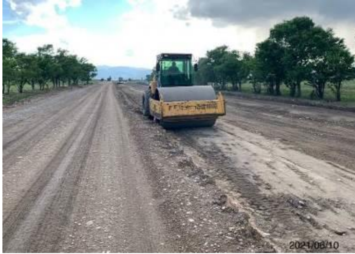
Photo 26. Subgrade soil compaction with moistening at km 79 + 300.
