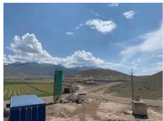
Photo 73. State of the production site of the crusher plant after watering.
