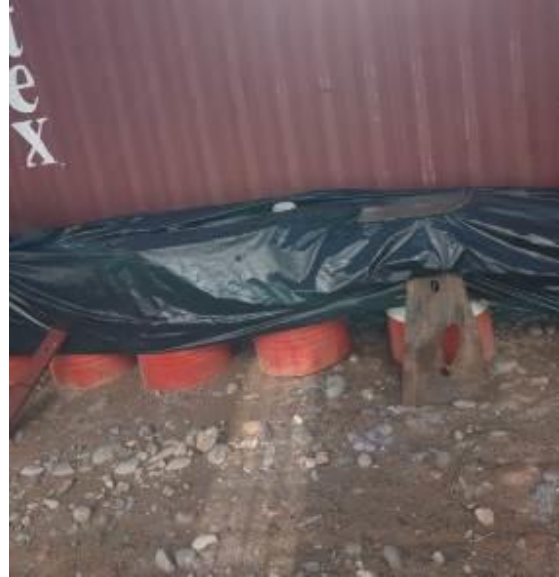
Photo 75. Lot 2. Cleaning of the territory and storage of containers with fuels under a protective film.
