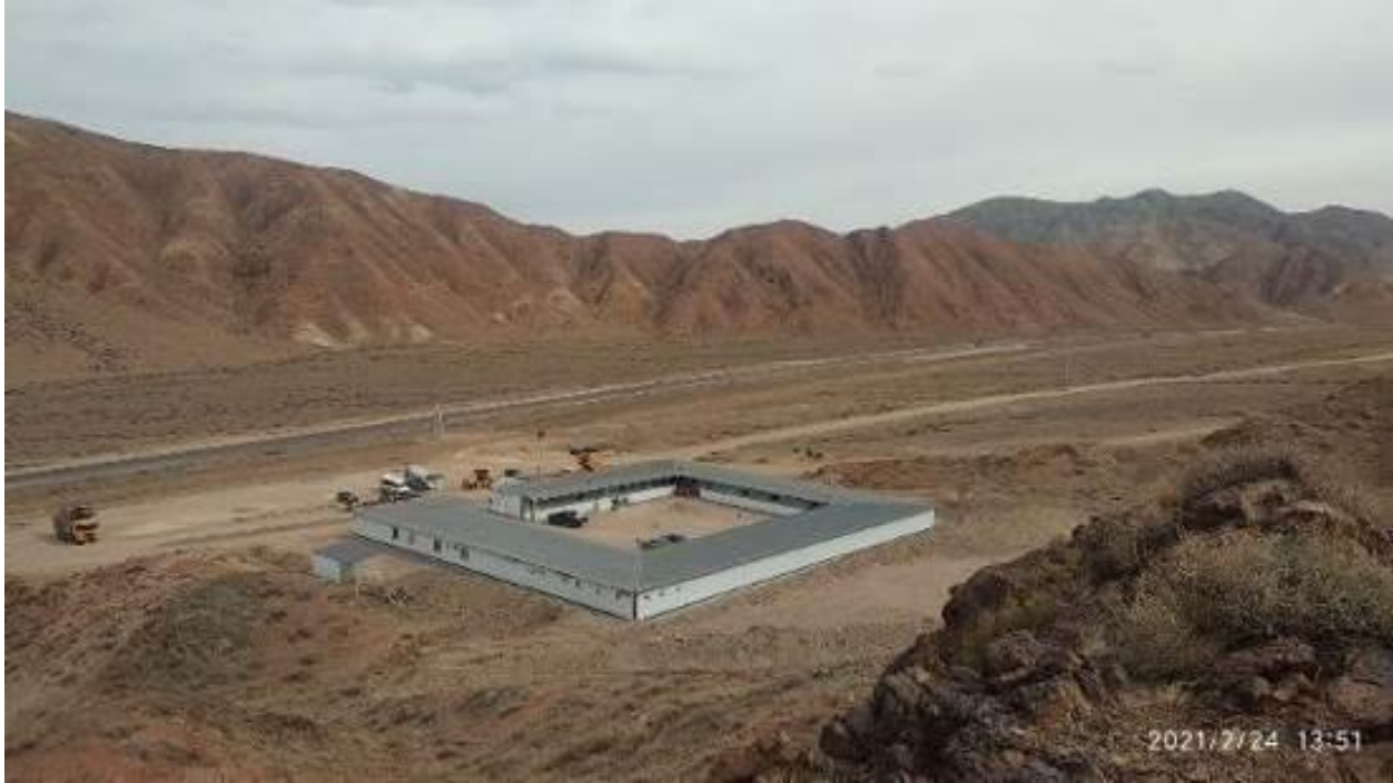
Photo 29. Location of camp road builders at km 16+100.
