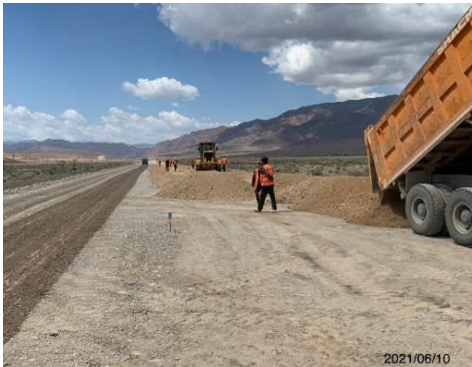
Photo 18. Lot 1. Earthworks on the embankment at km 4 + 200.
