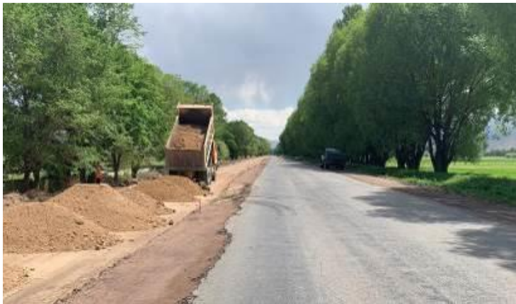
Photo 27. Embankment construction at km 64+300.
