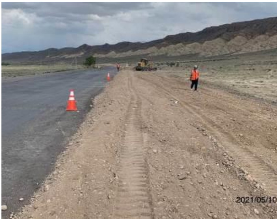
Photo 25. Km 74 + 100. Subgrade leveling.
