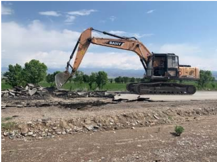
Photo 28. Scarifying of asphalt concrete pavement at km. 74 + 550.
