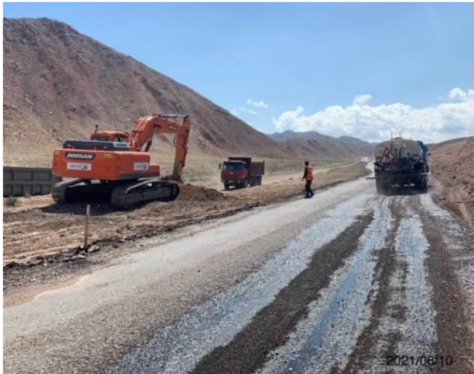
Photo 17. Removal of unusable material km.14 + 482.
