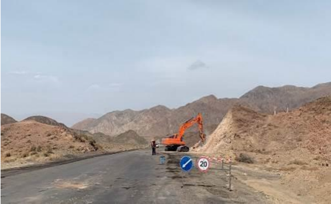
Photo 15. Lot 1. Excavation at km 21+000.
