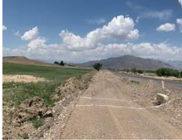
Photo 79. The area after cleaning km 75.
