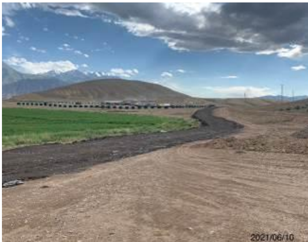
Photo 70, 71. Lot 2. Backfilled technological earthen road to the crusher plant.
