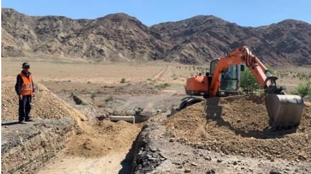
Photo 23. Culvert backfilling at km 18+585.
