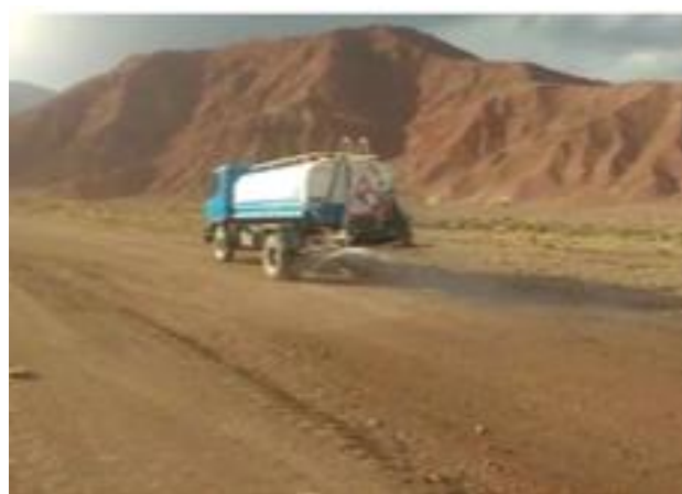
Photo 67. Pressure irrigation system.
