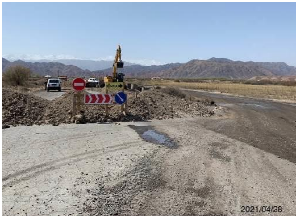
Photo 22. Lot 1. Culvert construction work at km 8 + 159.
