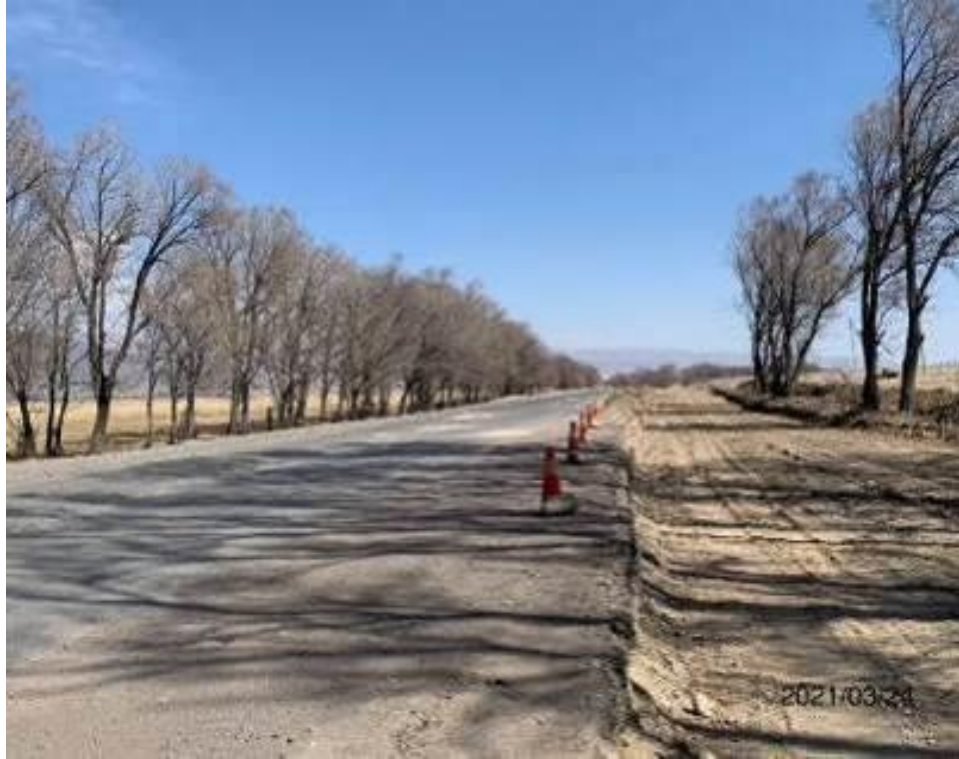
Photo 24. Road widening at km. 14 + 050 - 16 + 500: after clearing and grubbing.
