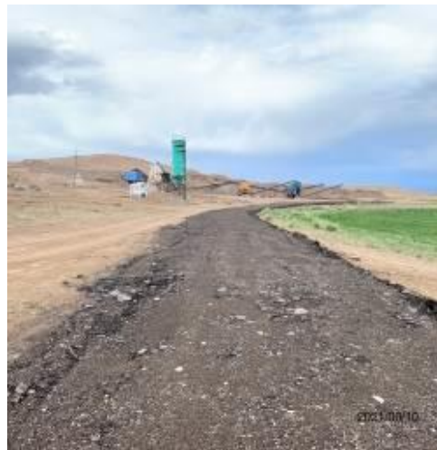
Photo 70, 71. Lot 2. Backfilled technological earthen road to the crusher plant.
