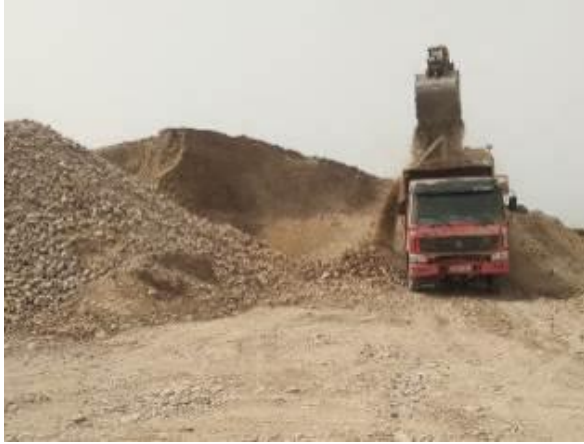
Photo 99. Lot 2. Loading of material at the quarry km. 75 + 400.
