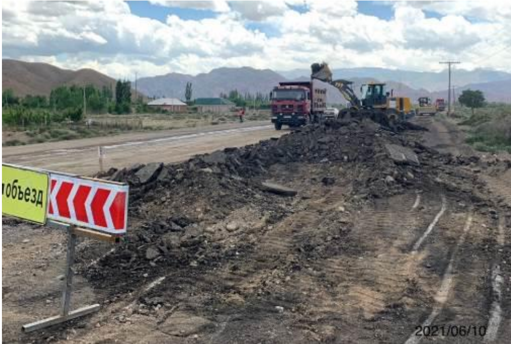
Photo 19. Lot 1. Scarifying and removal of old asphalt concrete at km 7 + 560.
