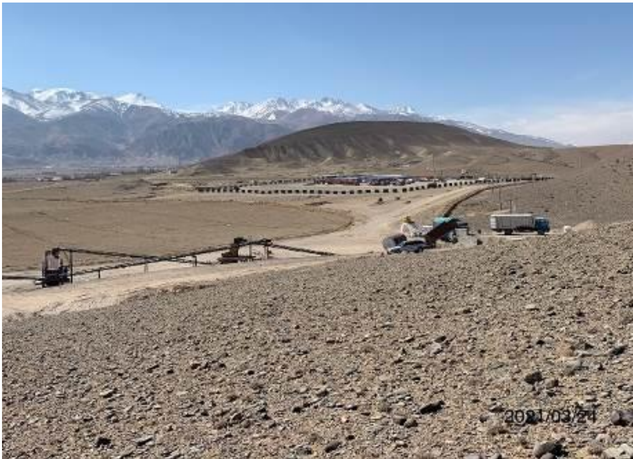
Photo 45. Contractor's camp location Lot 1.
