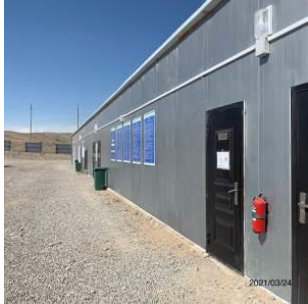
Photo 92. Lot 2. Fire extinguishers.
