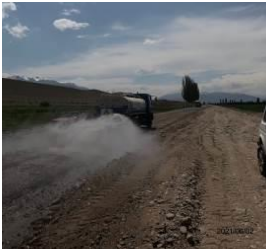
Photo 101. Lot 2. Hydraulic irrigation of the roadbed.
