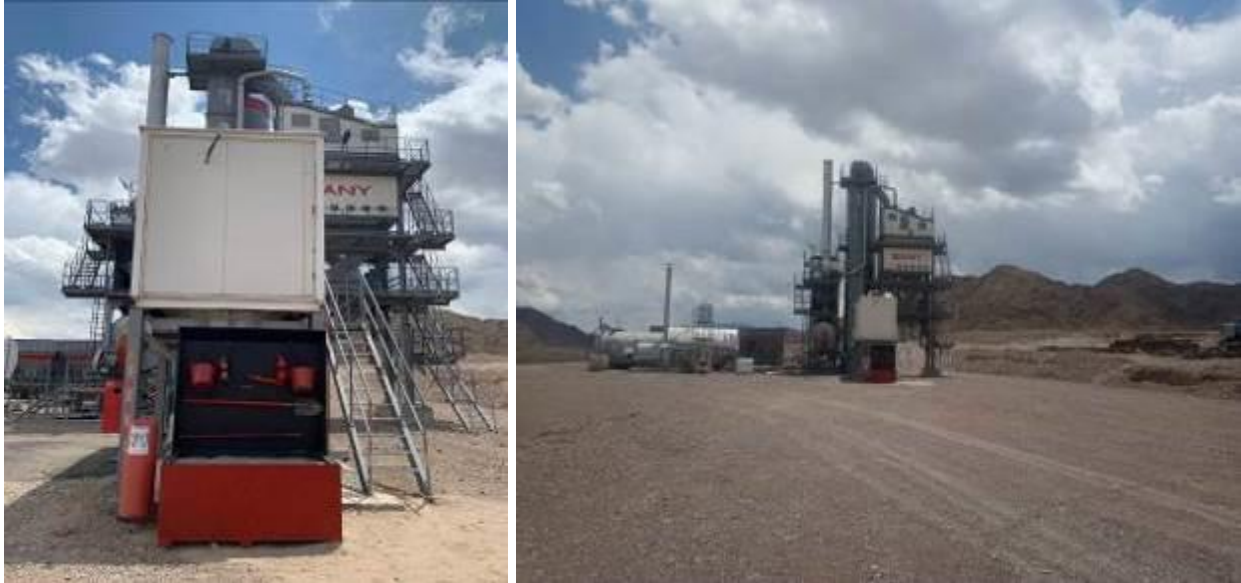
Photo 103-104. The state of the territory after the completion of the arrangement of the concrete plant.
