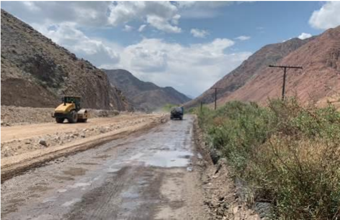
Photo 16. Soil compaction at section km 13 + 280.
