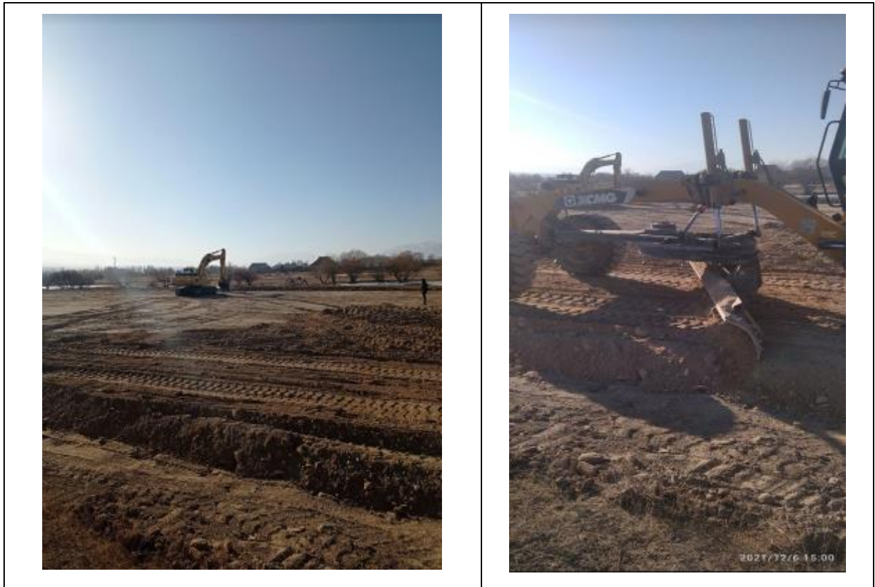
Figure 4. Work on the new production site territory.
