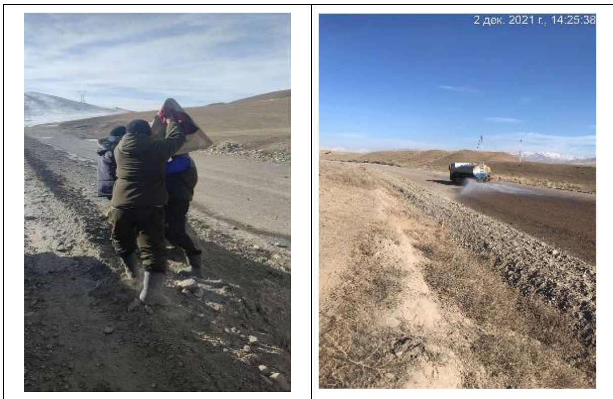
Figure 3. Work on the project area.
