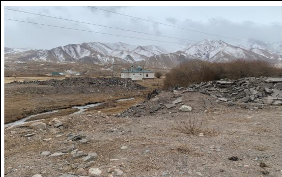
Photo 3. Old asphalt piled up on both sides of the river
