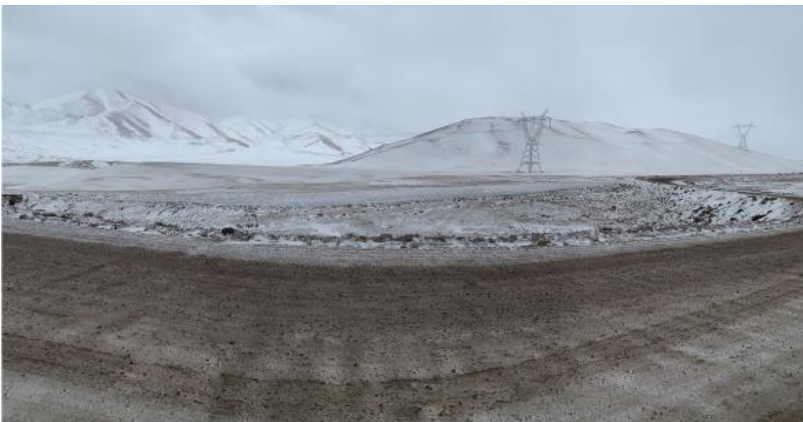
Photo 12. Spoiled area (leveled)
