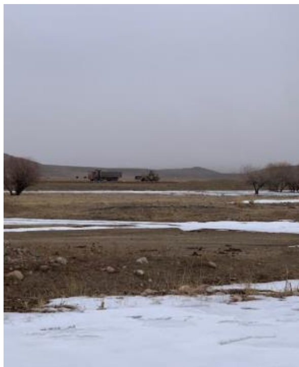
Photo 16. Leveling the area for production base site
