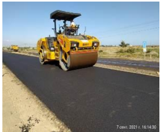
Photo 13: Compaction of the asphalt base at km 3+140-km 3+700.
