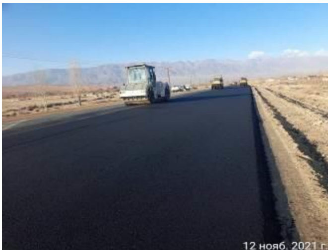
Photo 12. Bottom layer of asphalt concrete km 8+845-9+269 LHS.
