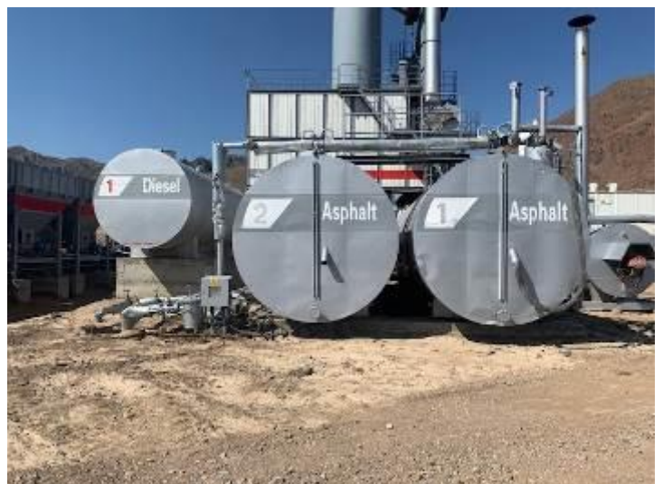
Photo 55. Storage area for tanks with bitumen and diesel fuel.
