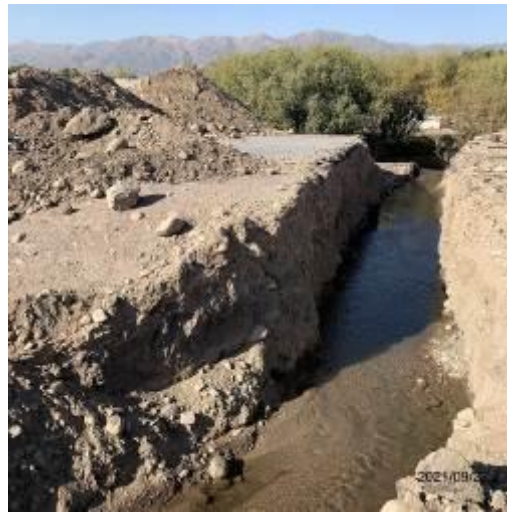
Photo 94. Lot 2. Drainage from sections of new culverts km 86+220.
