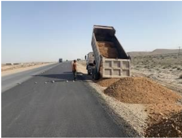
Photo 8. Earthworks for the embankment of road shoulder at km. 7+350.
