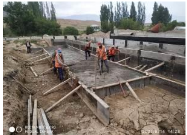
Photo 17: Fastening with a steel beam of bank bridge abutment km 12+063.
