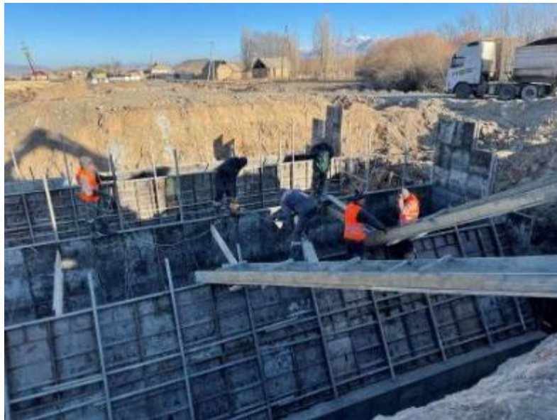
Photo 32. Pouring of the bridge abutment at km 88+795.
