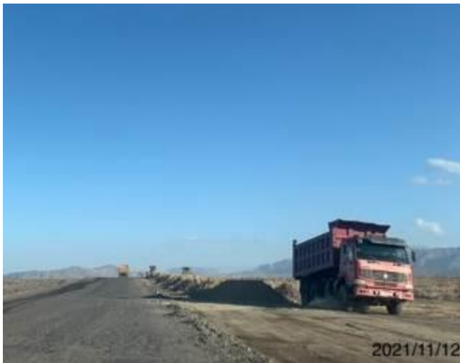
Photo 10. Arrangement of sub-base at km 24+260-24+700.
