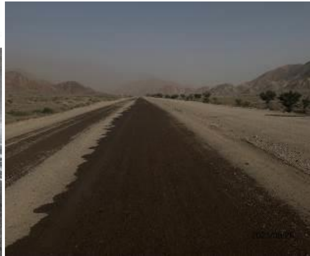
Photo 87. Water sprinkling of access roads to quarry and Photo 88 to production base of the CSU on Lot 2
