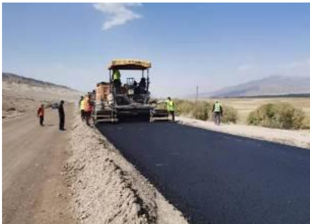
Photo 28. Laying of asphalt base at km71+880-72+640 (RHS).
