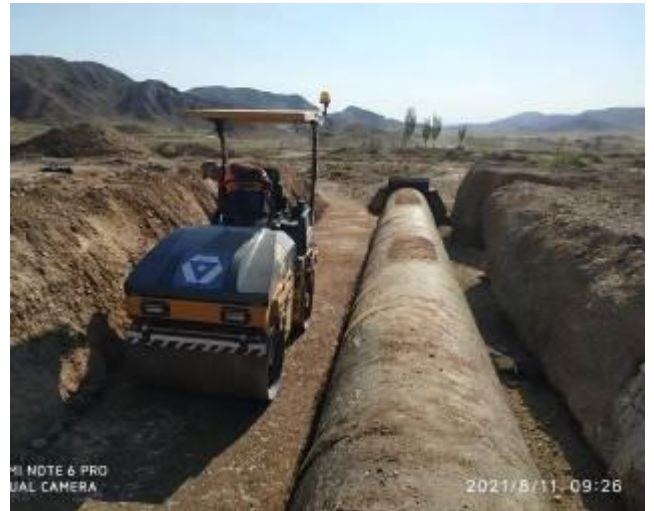
Photo 15. Backfill compaction of culvert at km 20+670.
