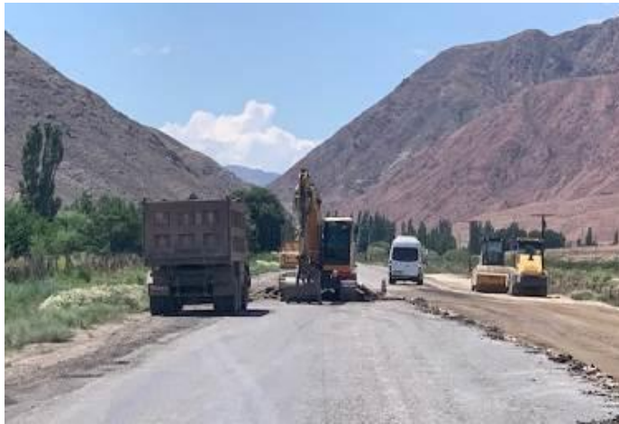
Photo 3. Scraping and removal of old asphalt concrete at km.10+900.
