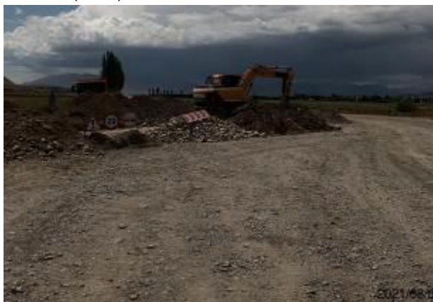
Photo 30. Backfilling of the in/out pipe km 80+100.
