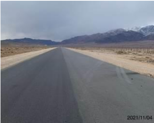
Photo 14: Bottom layer of 9 cm pavement at km 3+140- km7+000.
