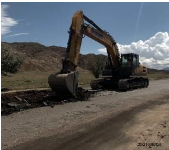
Photo 4. Scraping old asphalt at km 17+500.
