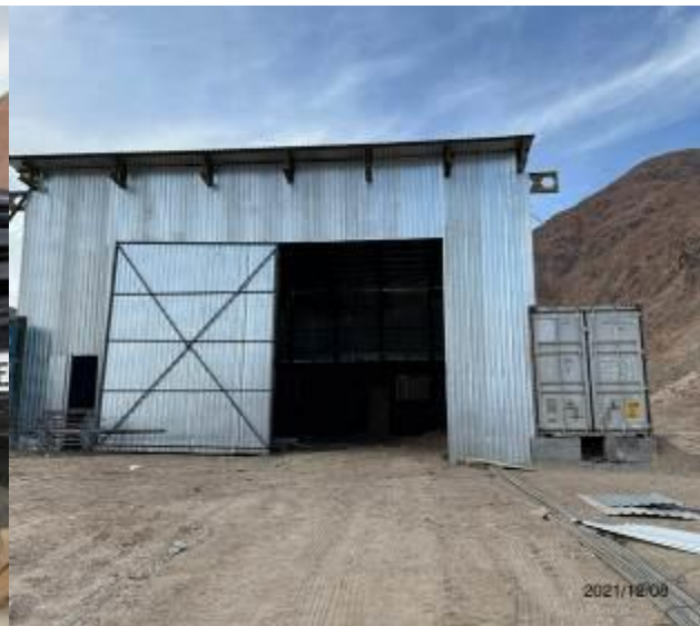
Photo 53. Machine repair box and nearby container for storing used oil.
