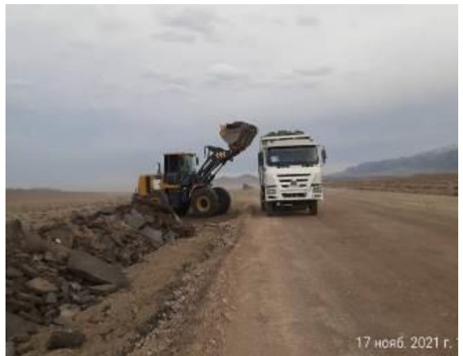
Photo 5. Scraping and removal of old asphalt at km.28+200-28+700 RHS.
