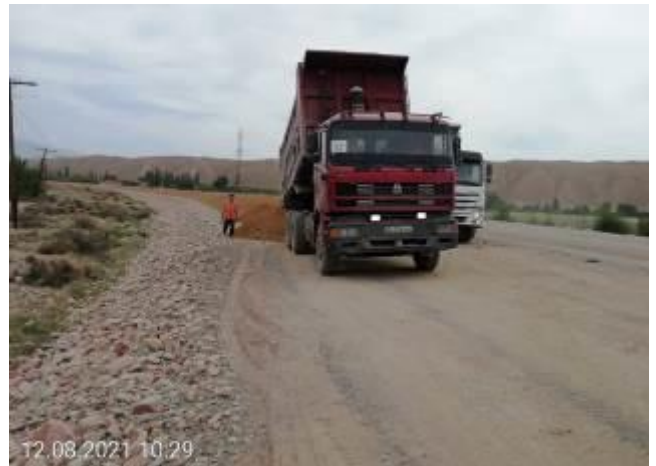
Photo 9. Laying subbase course km 10+100-10+600.
