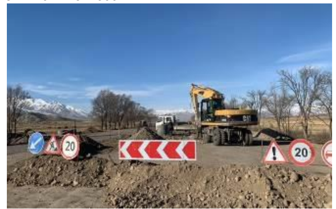
Photo 31: Installing the headers at km 78+772.
