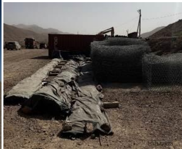
Photo 92. Storage of materials on Lot1.
