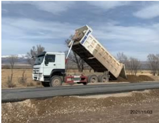
Photo 22: Road shoulder embankment at km.
