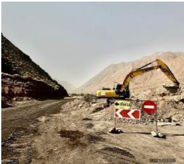
Photo 16: Backfill of pipe at km 16+150.
