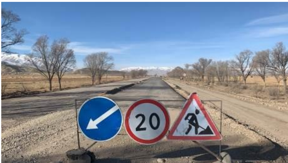
Photo 19: Section after widening and shaping of roadway at km 78+840.
