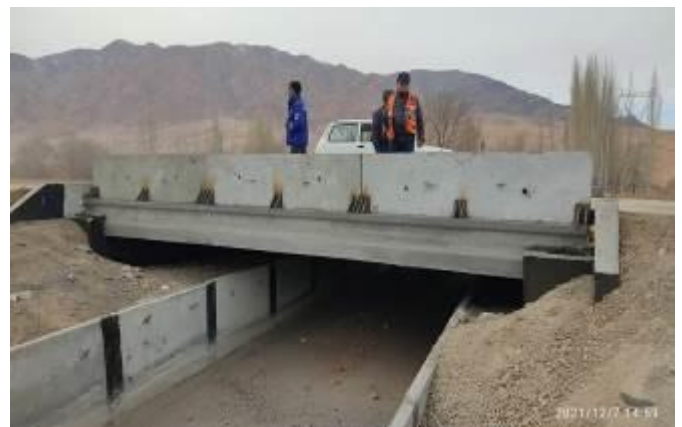
Photo 18. Bridge construction completed.
