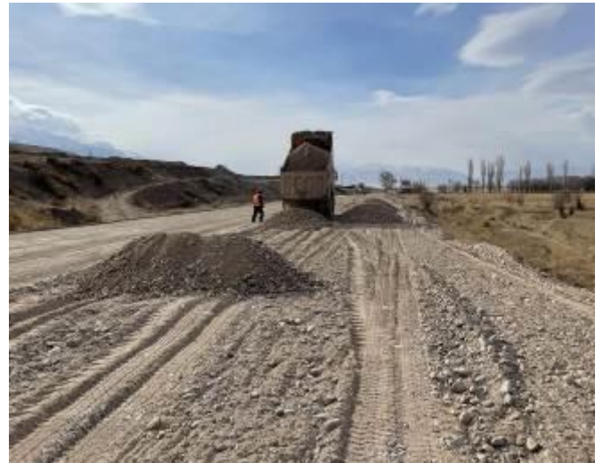
Photo 27. Works on laying base course km 80+660 - 81+260.
