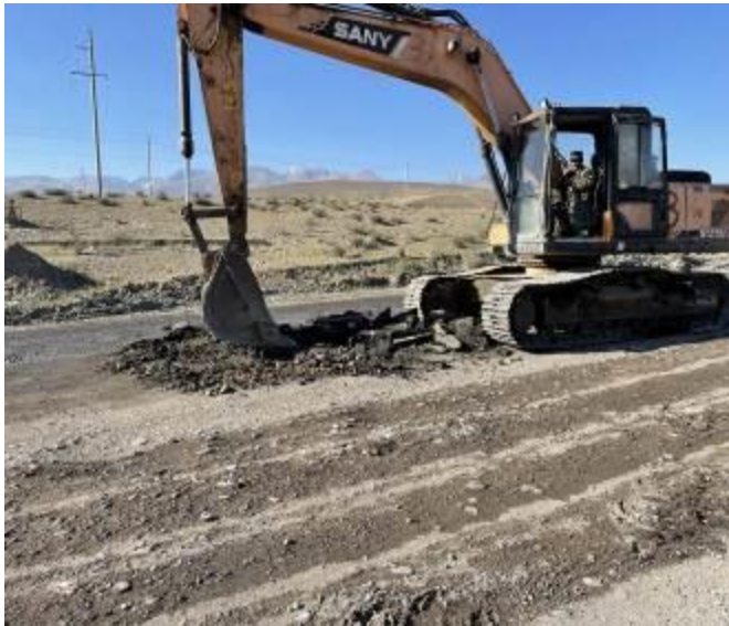
Photo 20. Removing existing asphalt pavement at km. 81+460-81+500.
