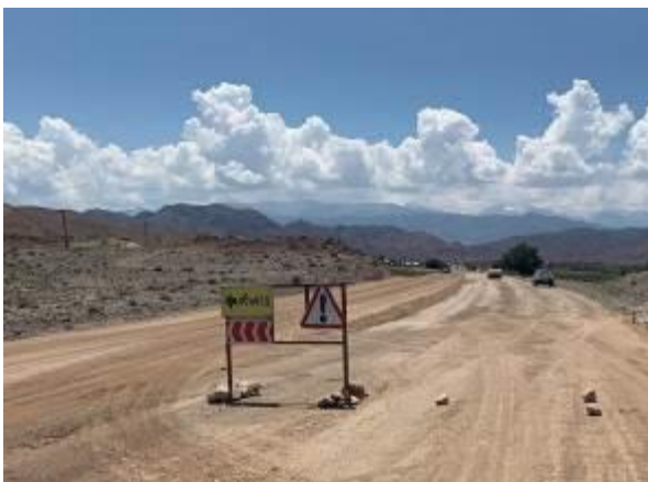
Photo 6. Compaction of roadbed soil at km. 7+800.
