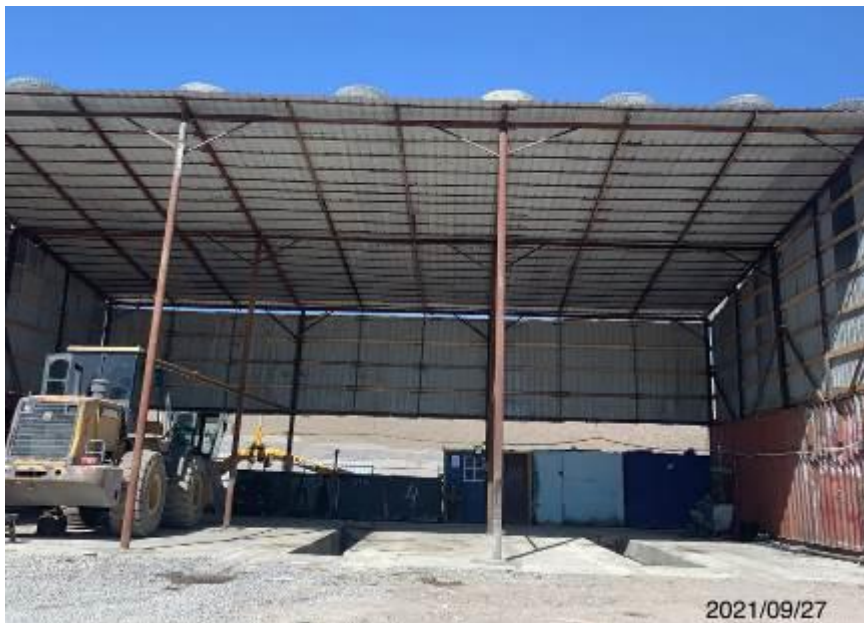
Photo 67. Specialized area for the inspection and repair of transport and construction equipment.
