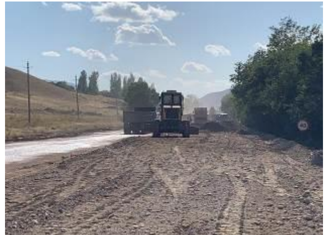
Photo 23: Earthworks at km. 85+430
