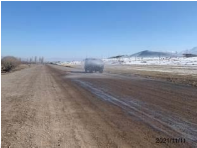
Epkin Photos 84, 85. Water sprinkling of unpaved road sections on Lot 2.
