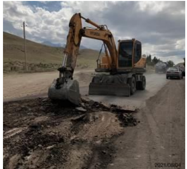
Photo 21. Removing existing asphalt pavement at km. 74+550.
