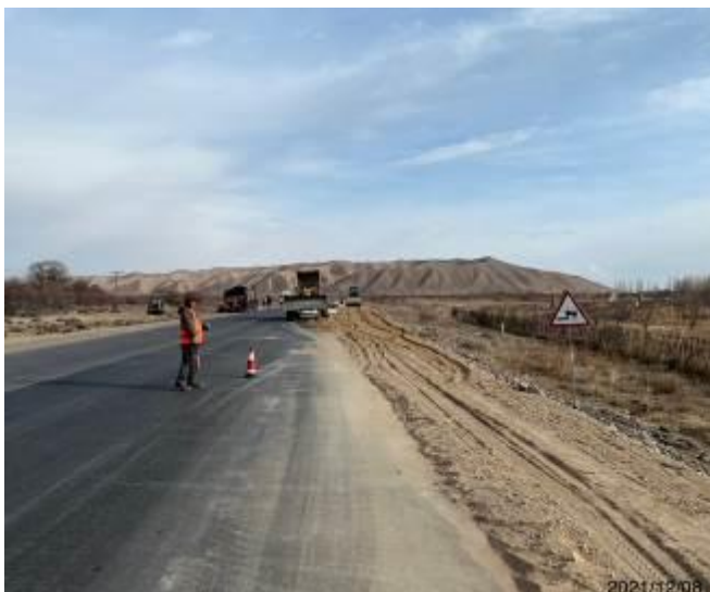
Photo 24. Arrangement of embankment of road shoulder.
