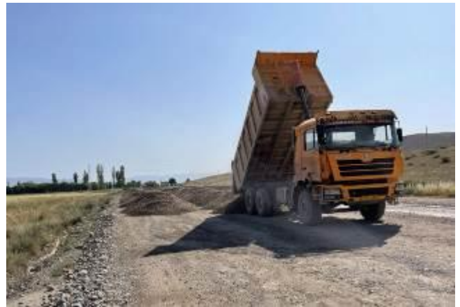
Photo 29. Preparation of bedding material at km 81+720-km 82+300.
