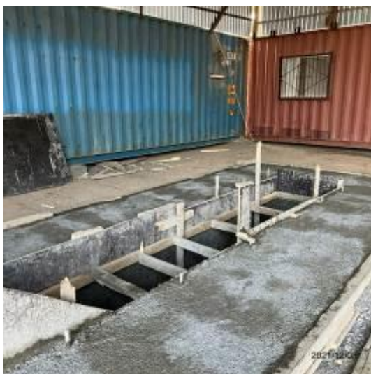
Photo 54. Concreted inspection pit inside the box.
