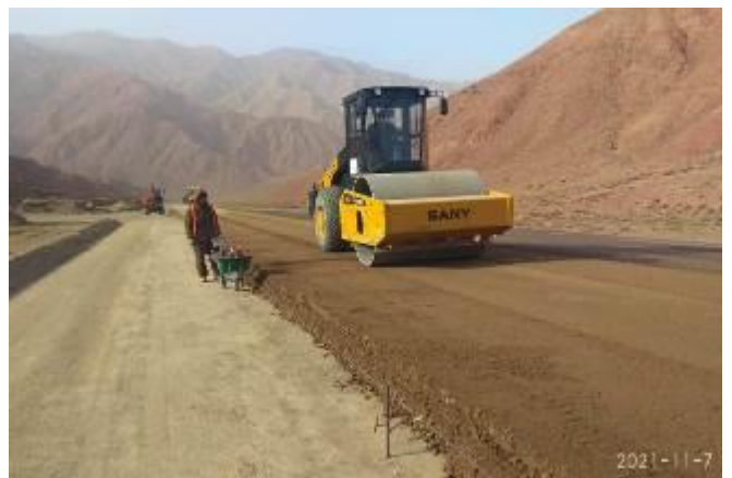
Photo 7. Compaction at km 12+300 - km 15+750.
