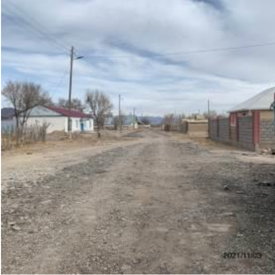
Photo 83. Improvement of internal roads in village of
