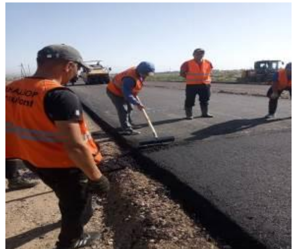
Photo 11. Laying of asphalt concrete on section km 3+140 - km 5+000.
