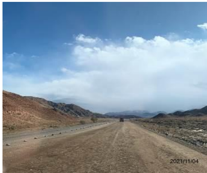
Photo 2. Road widening on the section km. 17+500-18+500: after clearing and uprooting.
