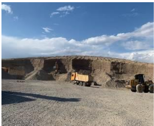
Photo 60. Lot 2. Quarry km 71+500.
