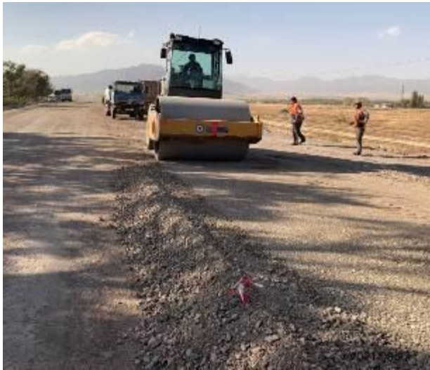
Photo 26. Earthworks of km. 76+540.
