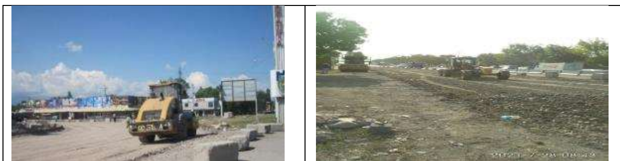
Figure 3 Removal of asphalt in the Sokuluk village.
