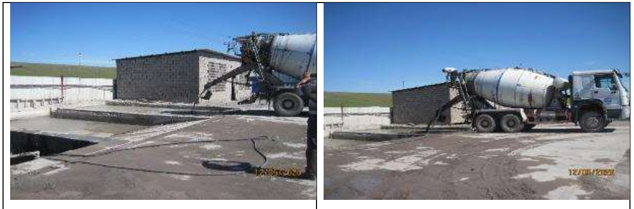
Figure 59 Washing of concrete mixer trucks.
