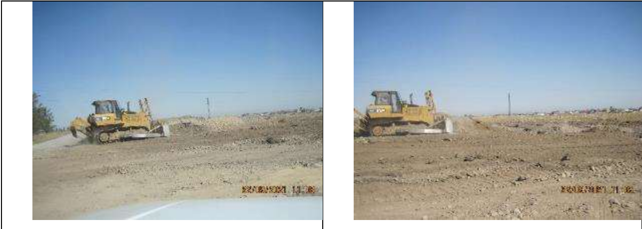
Figure 93 Transportation of unsuitable soil to a prepared area.
