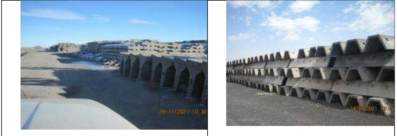
Figure 61 Polygon for the production of reinforced concrete products.
