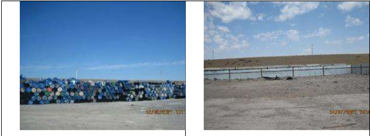
Figure 38 Barrels of bitumen on a special prepared site. Empty barrels after use and a storage area after the removal of used barrels
