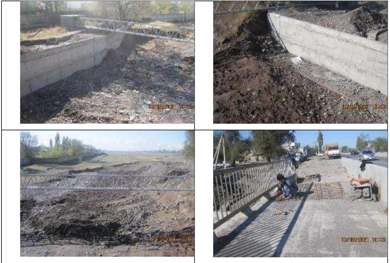
Figure 47 Ak-Suu River after completion of construction.
