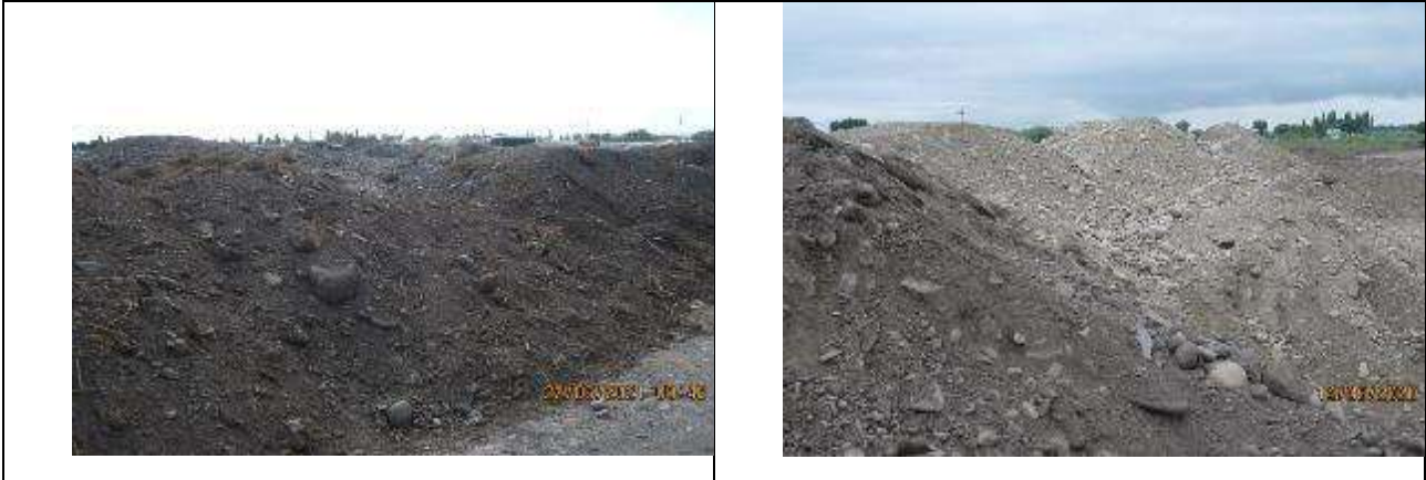
Figure 95 Storage of unsuitable soil for further use.
