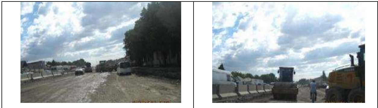
Figure 21 Rolling and compaction of the soil at 7.4 km section.
