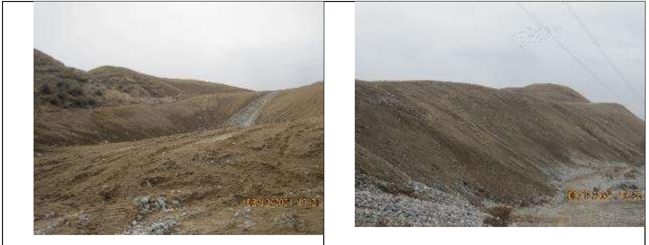
Figure 51 Jelamysh borrow pit after reclamation.
