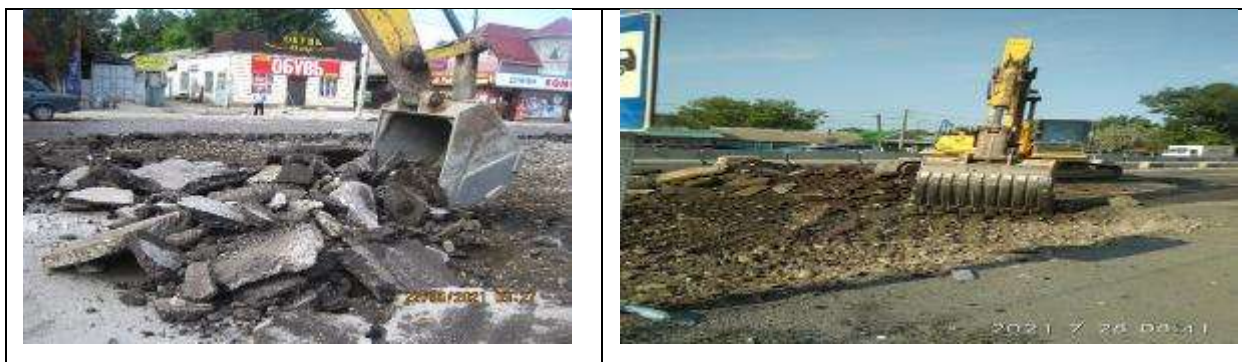
Figure 3 Removal of asphalt in the Sokuluk village.
