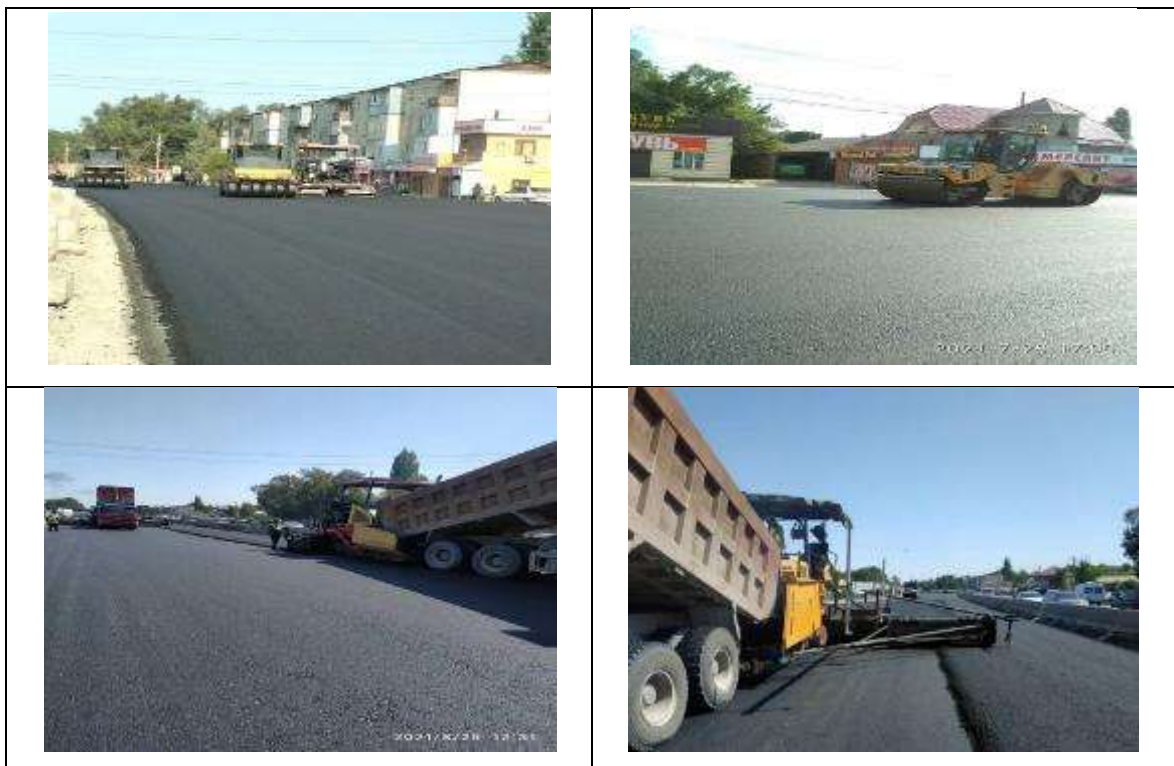
Figure 5 Laying asphalt from km 15.9 to km 61.
