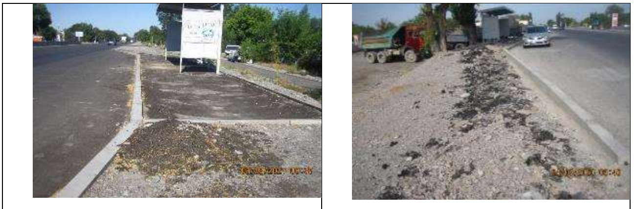
Figure 44 Remnants of asphalt scraps at bus stops.
