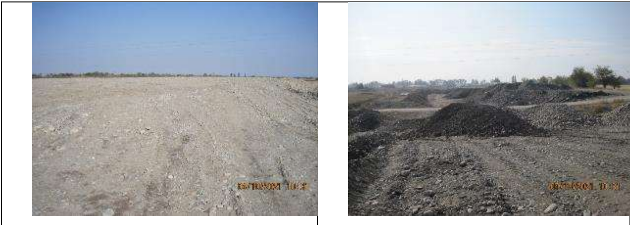
Figure 94 An area for storing unsuitable soil after transportation and levelling the unsuitable soil.
