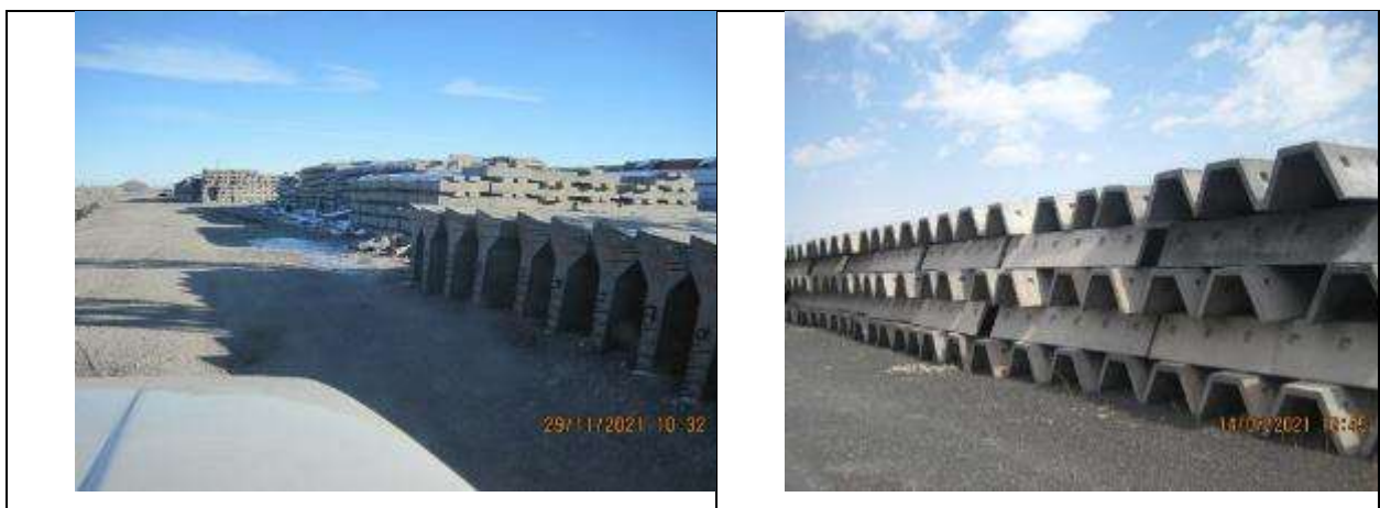
Figure 33 Production of reinforced concrete structures.
