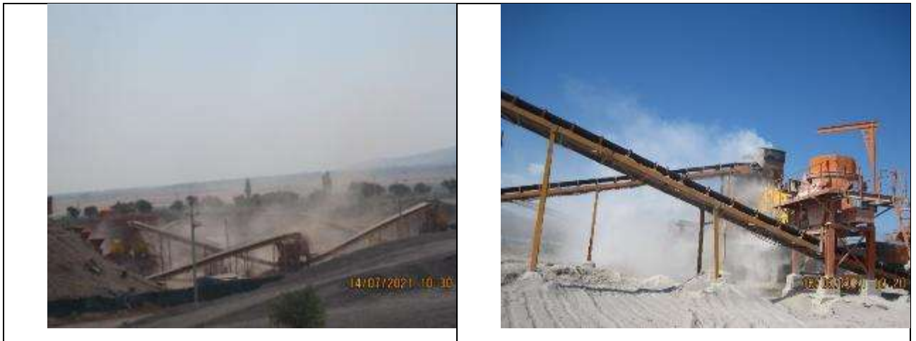
Figure 54 Operation of the stone crushing plant without watering the raw materials.
