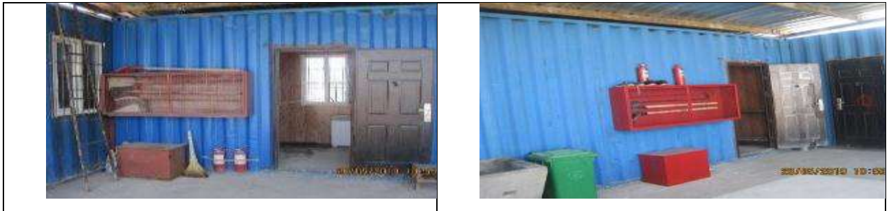
Figure 64 Fire shields on the territory of the camp
