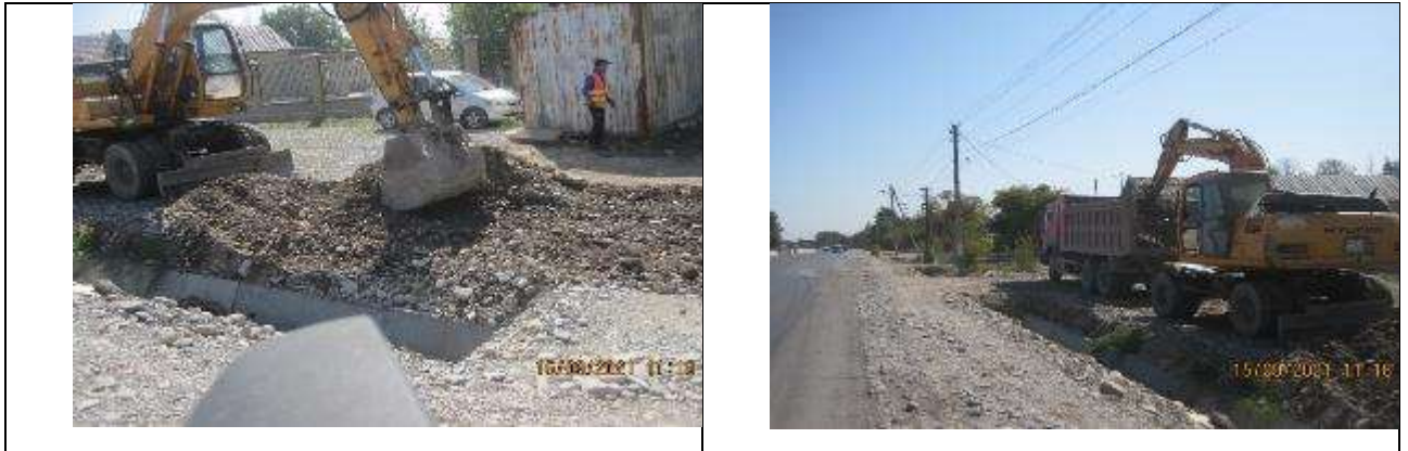
Figure 45 Removal of excess soil formed during the construction of culvert ditches.
