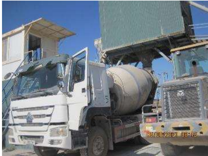
Figure 58 Refueling of concrete mixer trucks
