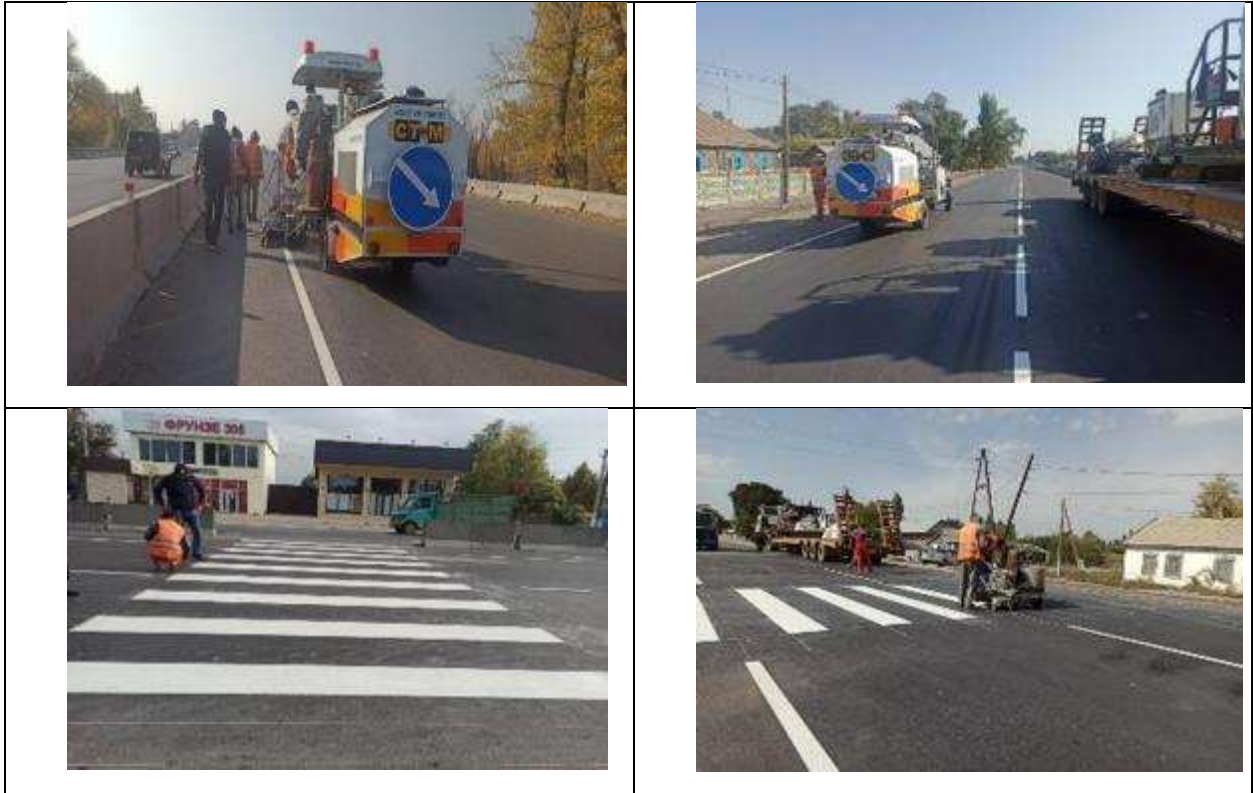
Figure 17. Application of horizontal markings.
