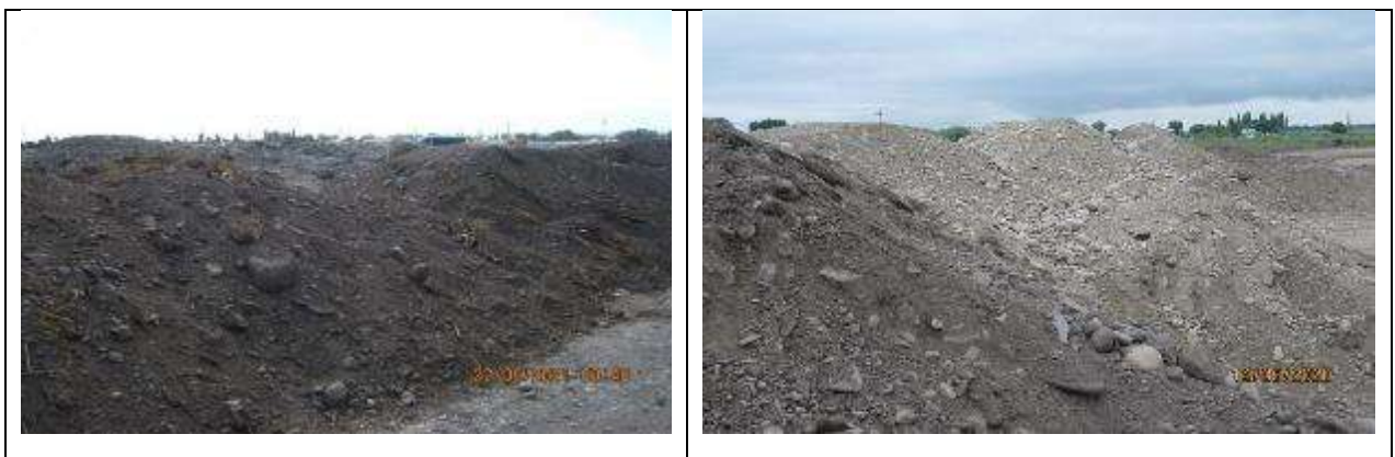
Figure 89 Storage of unsuitable soil for further use in the village of Romanovka.
