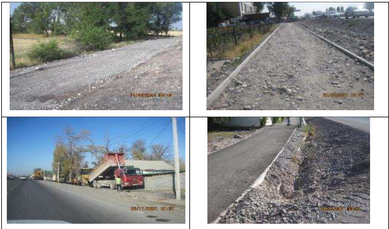
Figure 9 Construction of sidewalks.
