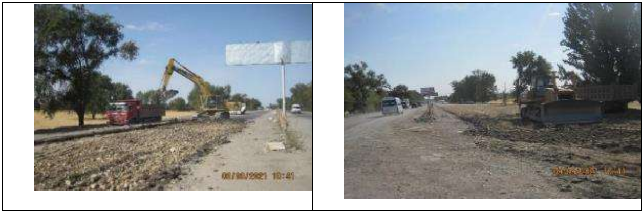
Figure 20 Leveling of the roadbed and removal of unsuitable soil.
