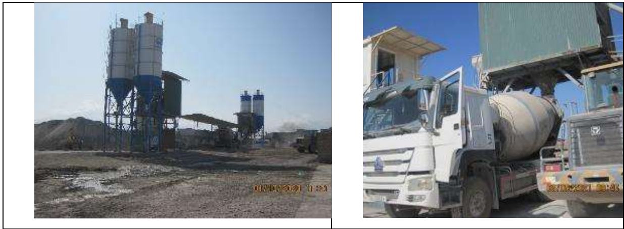
Figure 36 Filling the concrete mixing machine with concrete
