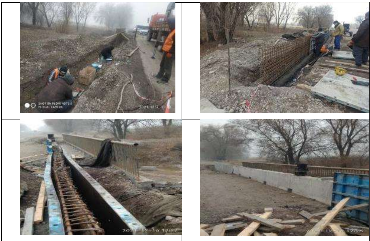
Figure 19 Construction wheel-safety parapet barrier on the Jelamysh river
