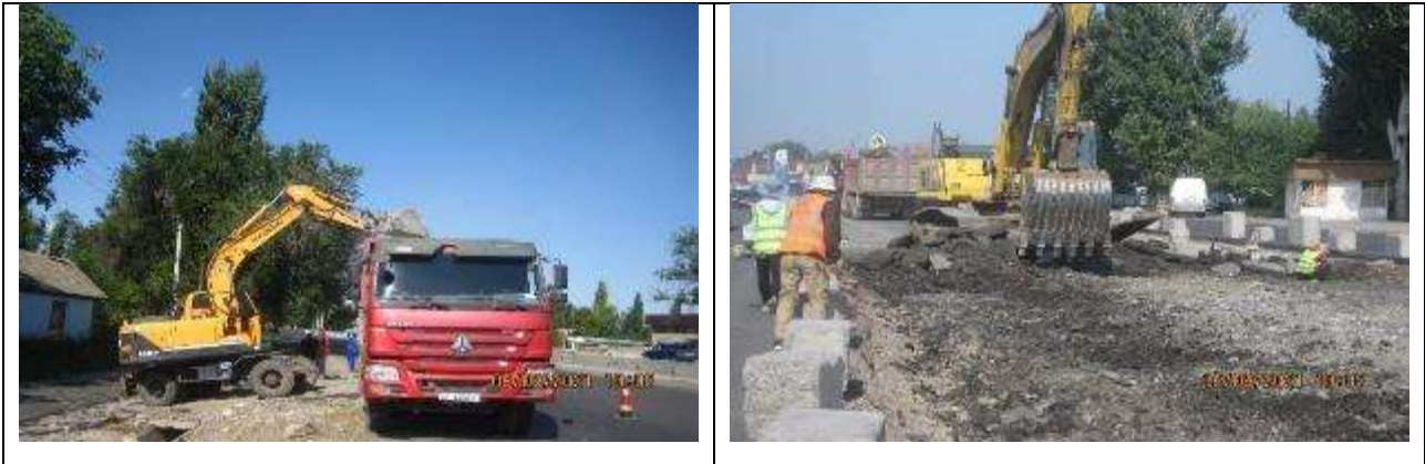
Figure 87 Transportation of removed asphalt to Sadovoye and Novopavlovka villages.
