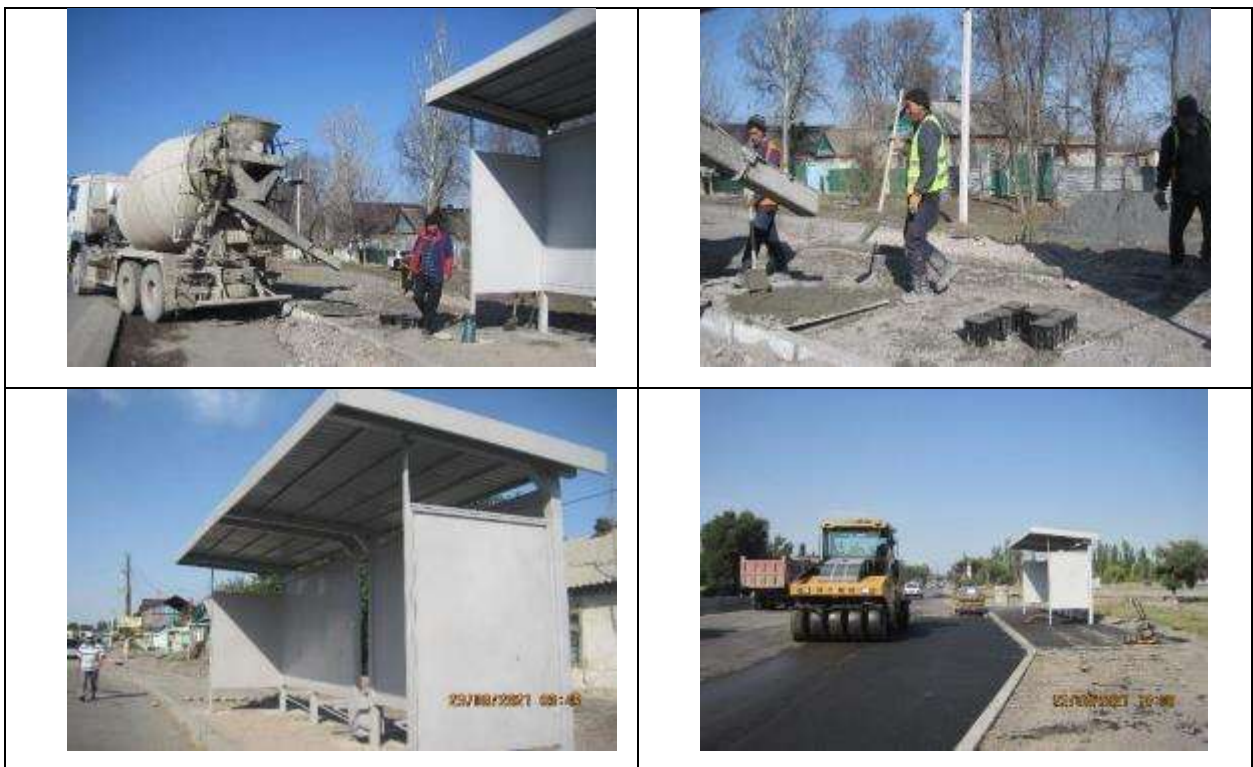
Figure 12 Construction of bus stops.
