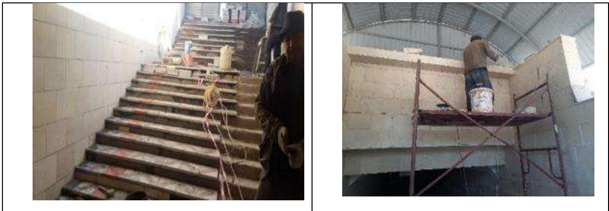
Figure 14 : Completion works on underpasses.
