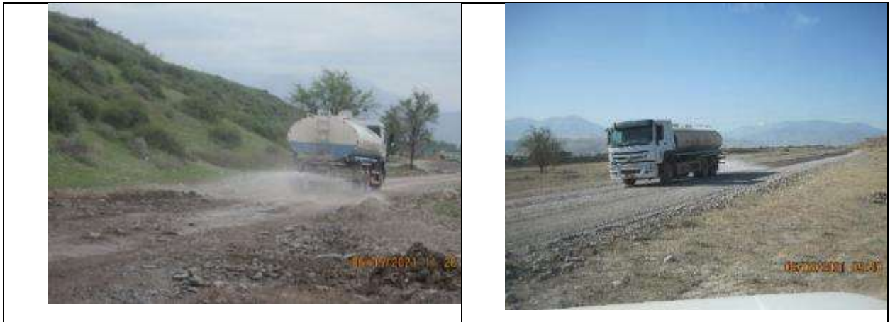
Figure 26 Water sprinkling on the road to Ak-Suu 2 borrowpit to avoid dusting.
