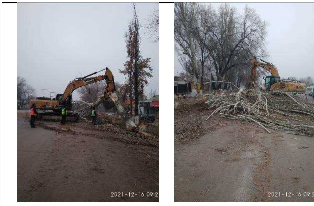
Figure 70 Tree cutting on the road section km 8.5 - 15.9.
