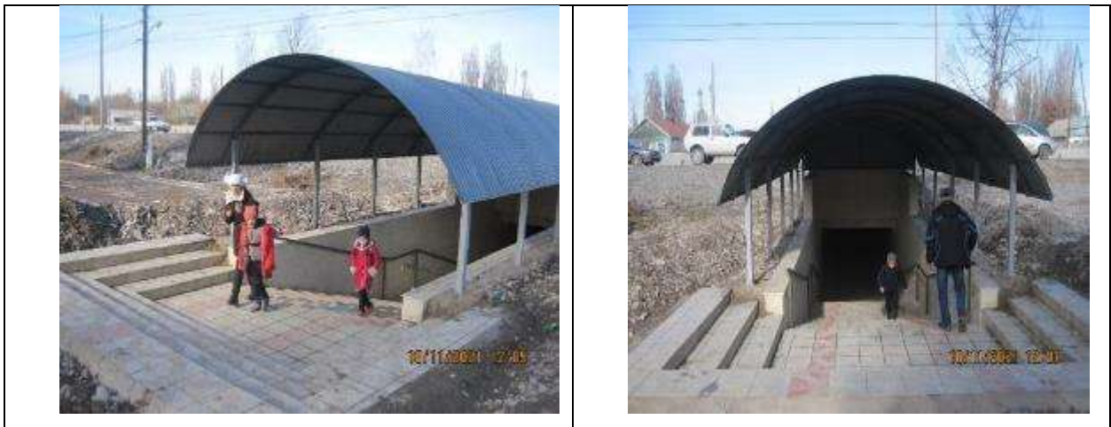
Figure 15 Underpass in the Novonikolayevka village.
