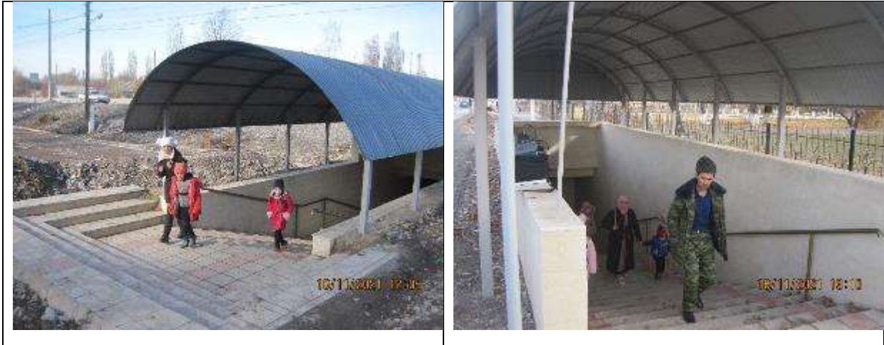
Figure 103 Local people using underpasses.
