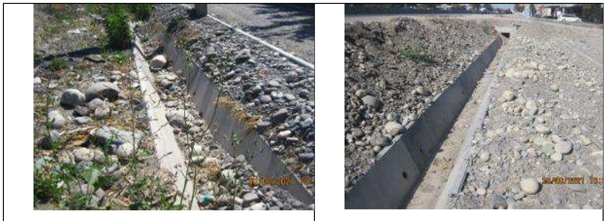
Figure 48 Condition of previously installed ditches before and after cleaning.
