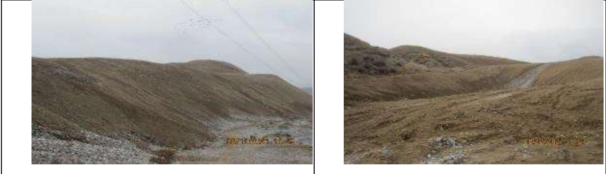
Figure 31 . Jelamysh borrow pit after the completion of reclamation works.
