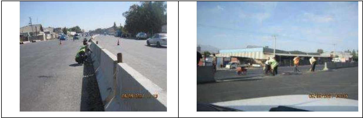
Figure 13 Works on concreting of ditches on the carriageway between the parapets.
