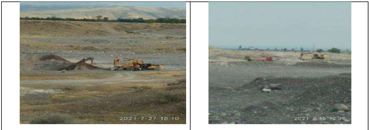
Figure 25 Leveling of used areas at the Ak-Suu 2 borrow pit
