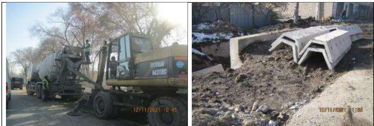
Figure 22 : Installation of roadside culvert ditches at 7.4 km section.
