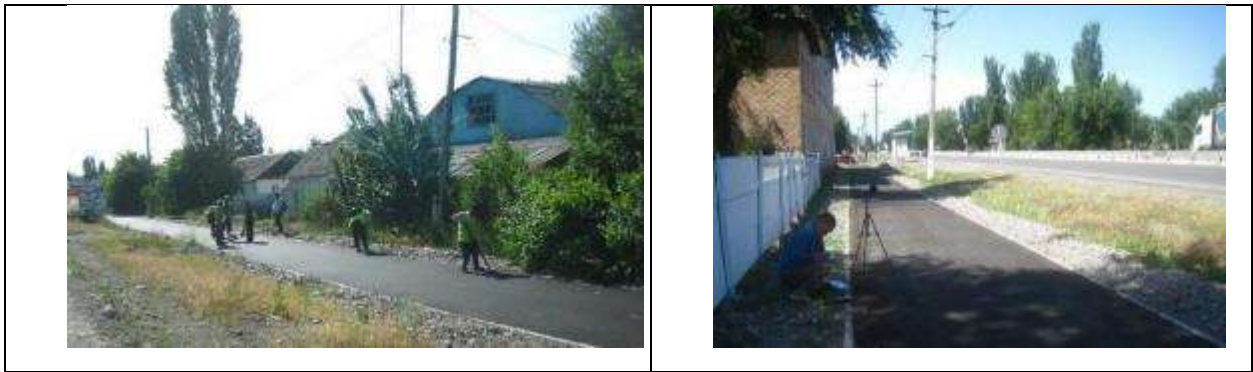
Figure 11 Construction of sidewalks in the Petrovka village.
