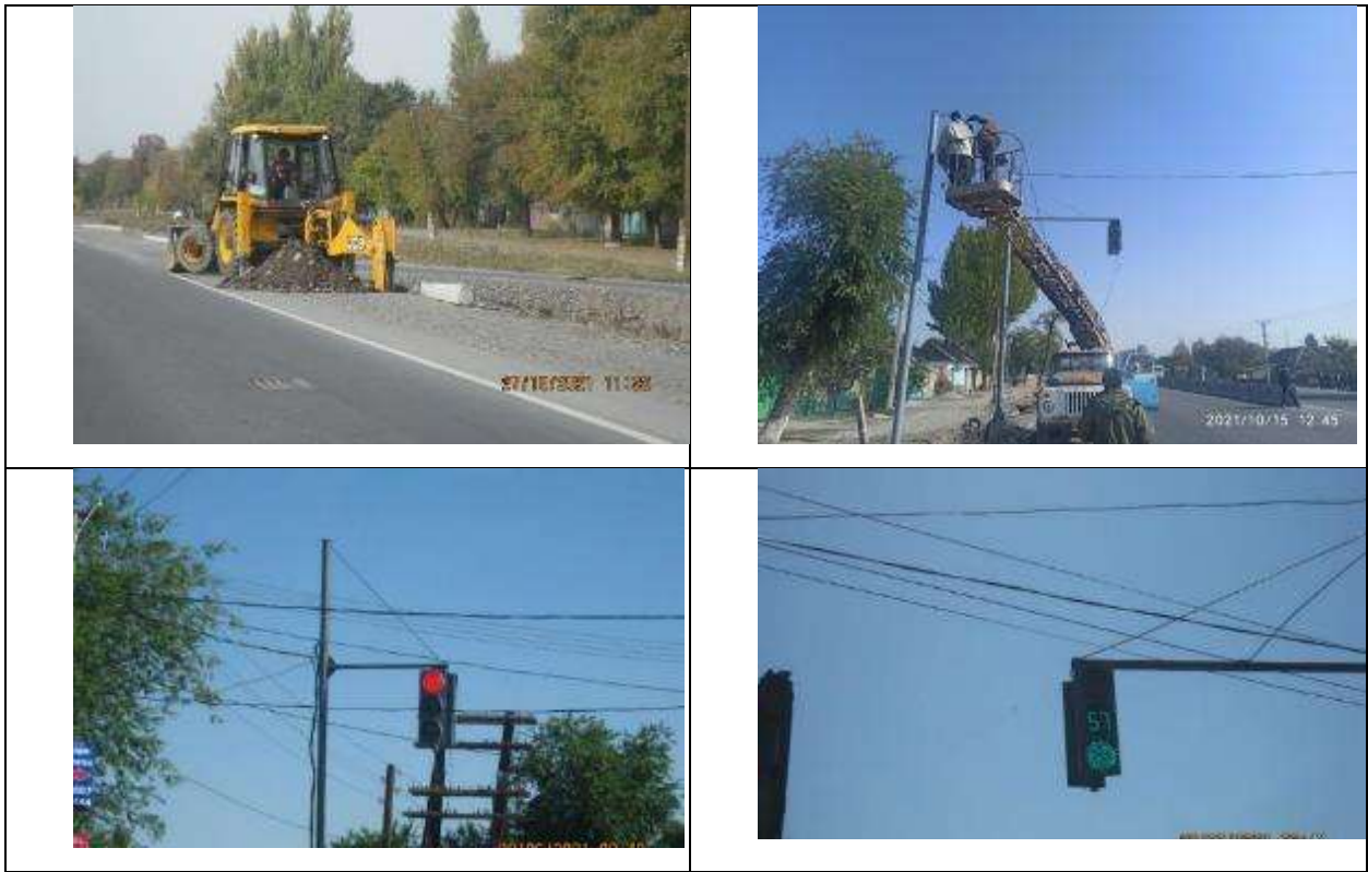
Figure 16: Installation of new traffic lights on the project road.
