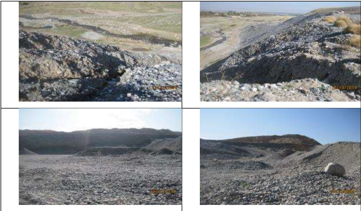
Figure 30 Jelamysh borrow pit after development.
