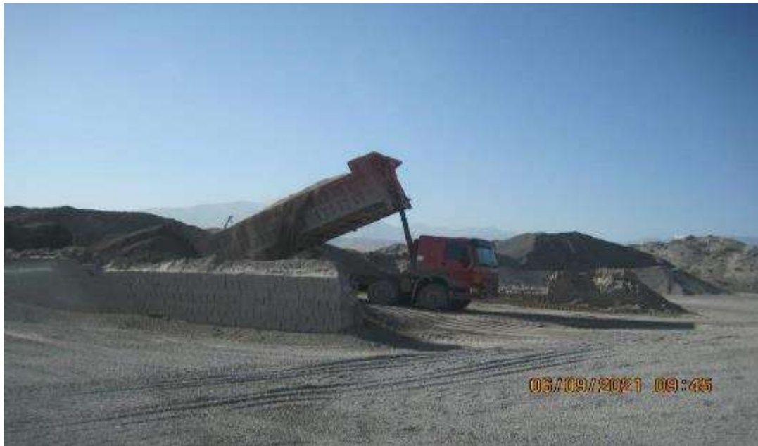
Figure 35 Preparation of gravel material for the production of concrete and asphalt
