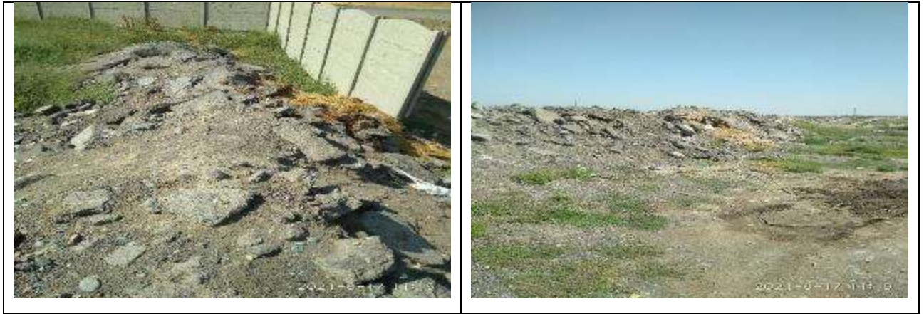
Figure 88 Dumping of old asphalt on designated areas in the Sokuluk village
