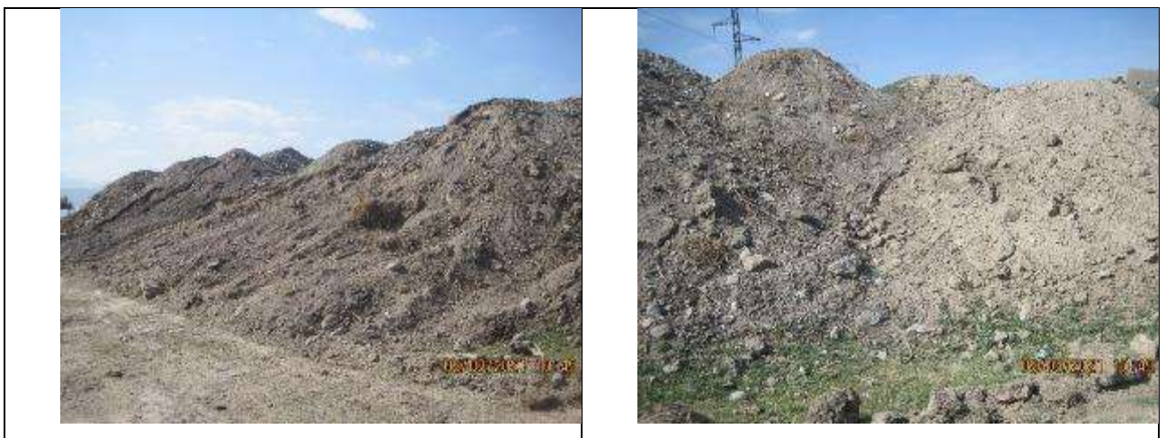
Figure 91 Dumping of soil unsuitable for road construction in the Voенно-Antonovka village.
