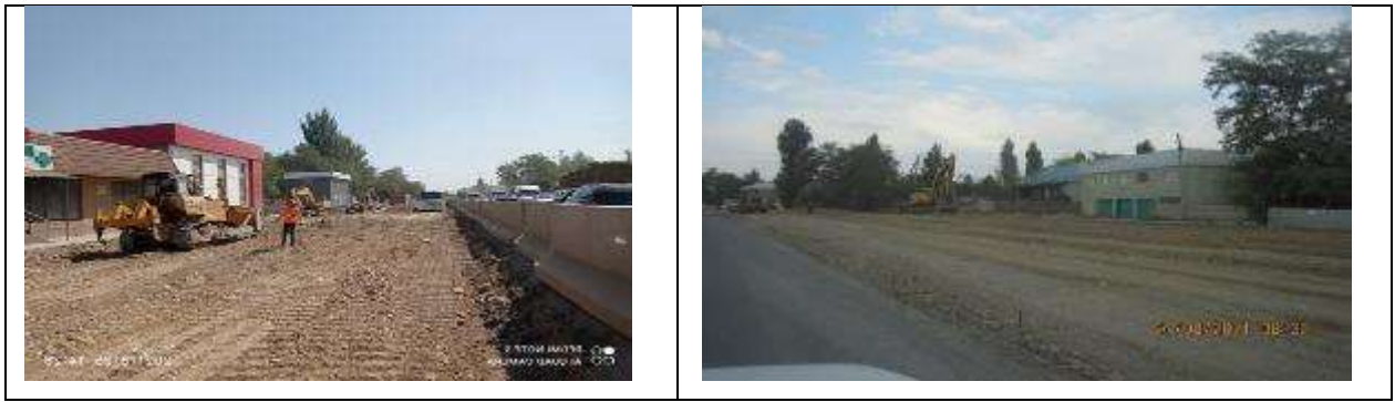
Figure 4 Leveling and compacting of roadbed in the Sokuluk village.
