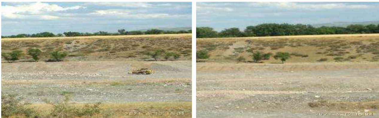
Figure 42 Reclamation works at the Ak-Suu 2 borrow pit
