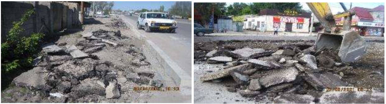
Figure 3 Removal of asphalt
