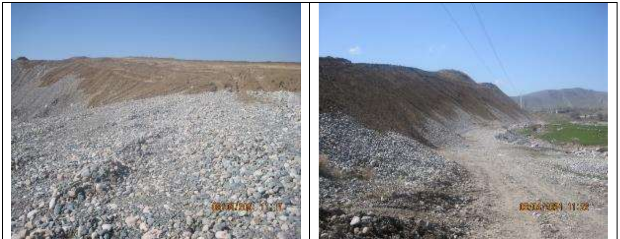
Figure 20 Jelamysh borrow pit after reclamation
