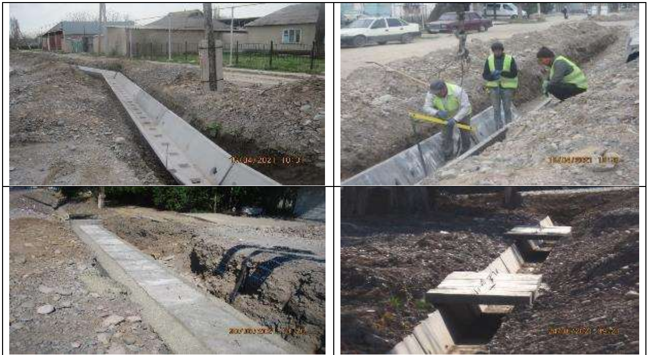
Figure 6 Installation of roadside culvert chutes and junctions adjustment to the road
