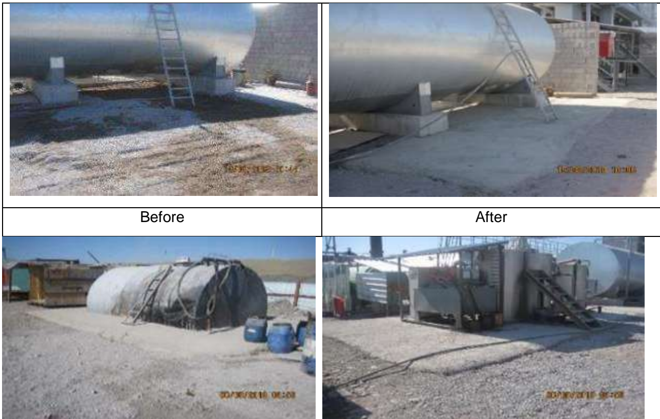
Figure 43 Impermeable protective coating around chemical containers
