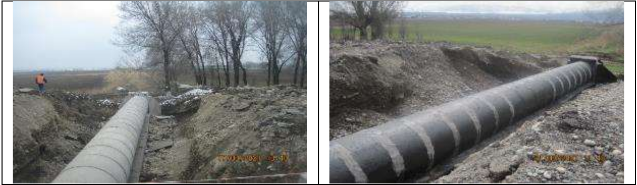
Figure 32 Laying of pipes at 7.4 km section
