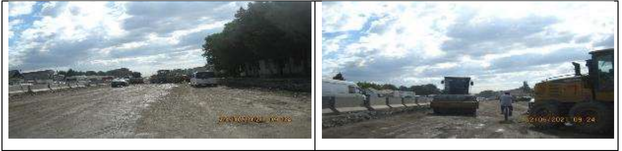
Figure 13 Rolling and compaction of soil at section KM 8+511 – KM 8+800
