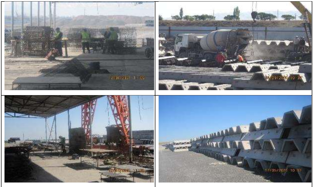
Figure 21 Production of reinforced concrete structures
