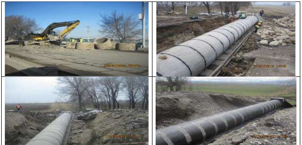
Figure 12 Construction of culvert pipes
