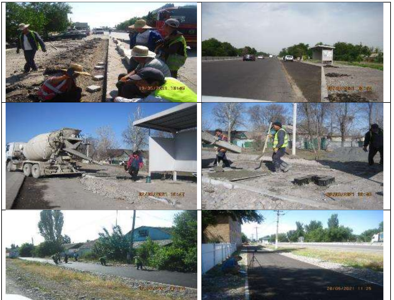
Figure 7 Construction of bus stops and sidewalk
