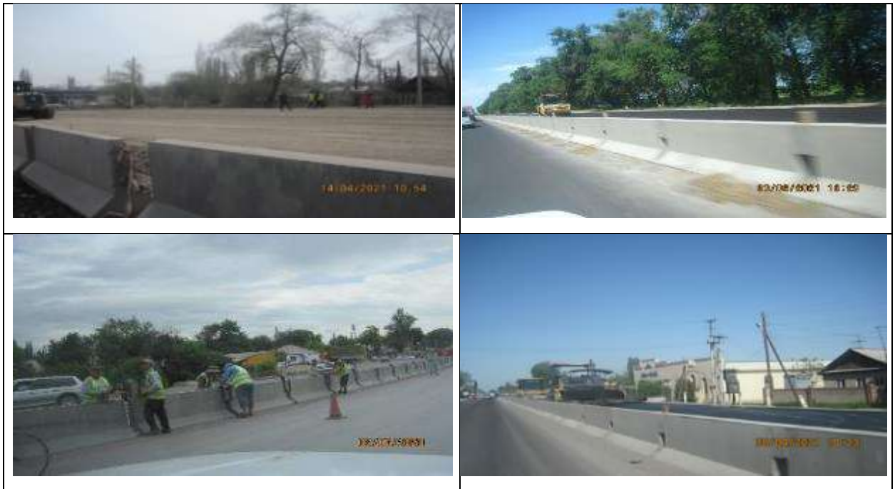
Figure 8 Installation and strengthening of New Jersey type parapets
