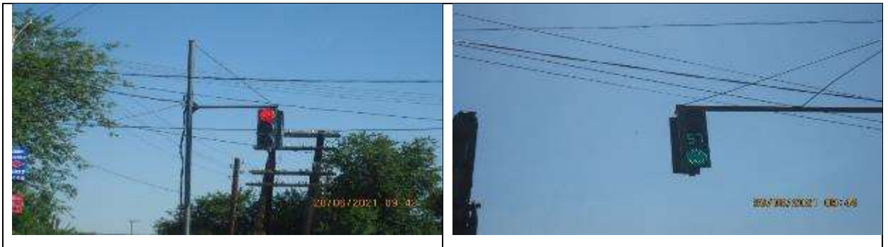
Figure 11 Installation of traffic lights
