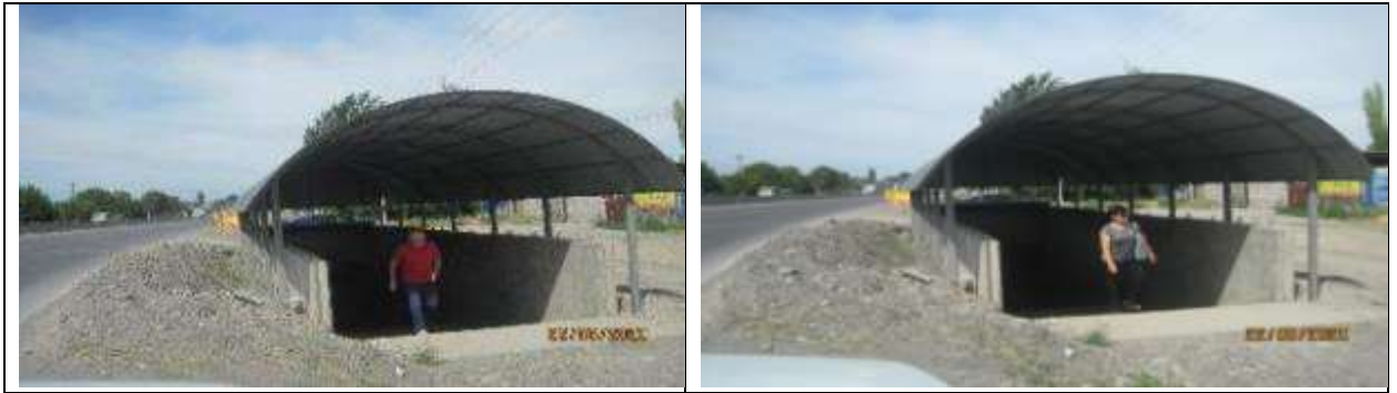
Figure 10 Construction and rehabilitation of underground passages
