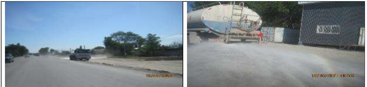
Figure 14 Dust control works (water sprinkling)
