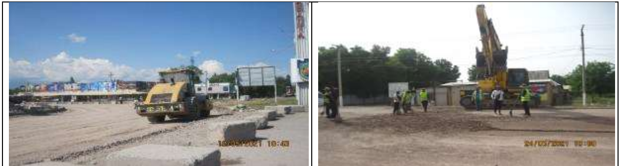
Figure 4 Leveling and compacting of roadbed
