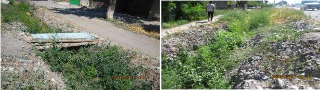
Figure 35 Previously excavated and abandoned trench for culvert chutes
