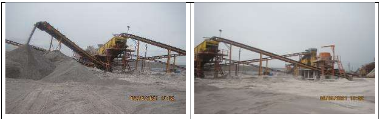
Figure 22 Stone crushing plant
