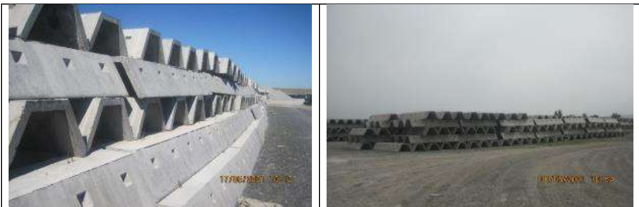
Figure 49 Polygon for the production of reinforced concrete products
