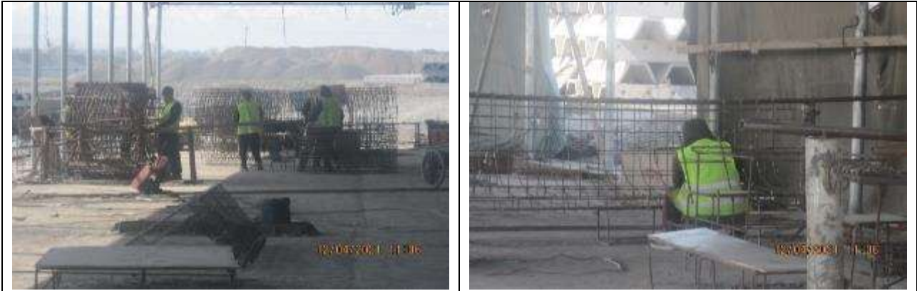
Figure 45 Work of the reinforcement-welding section
