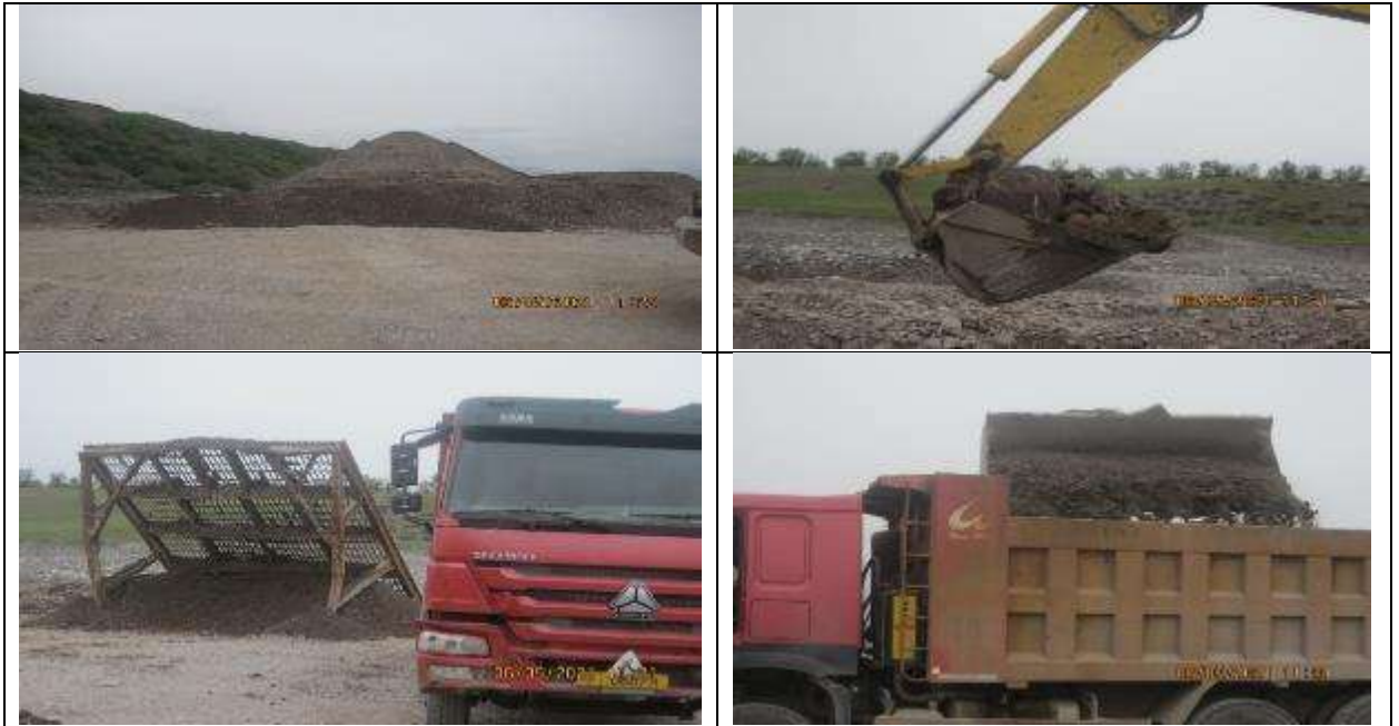
Figure 15 Development of Ak-Suu 2 borrow pit
