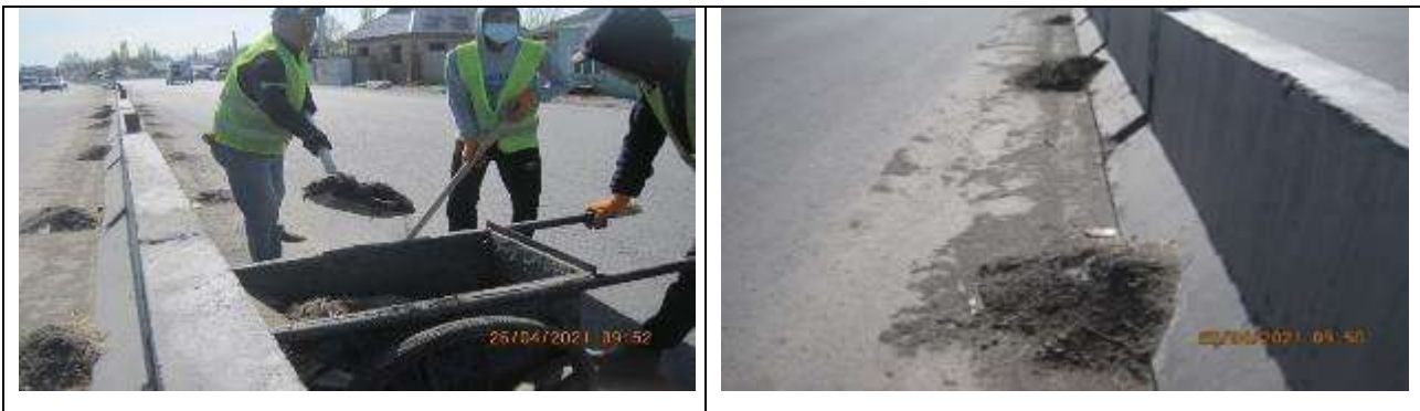
Figure 36 Cleaning parapets from accumulated soil
