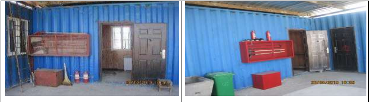
Figure 52 Fire shields on the territory of the camp
