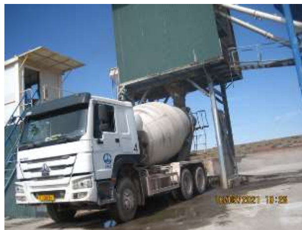
Figure 46 Refueling of concrete mixer trucks
