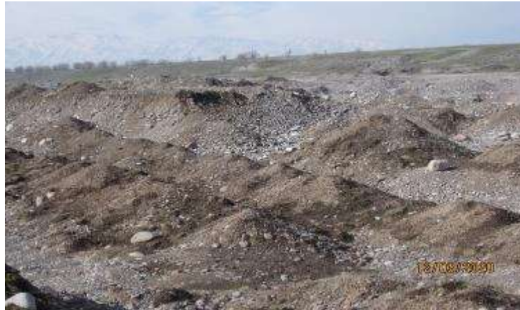
Figure 41 Areas disturbed in the process of subsoil use in Ak-Suu 2 borrow pit
