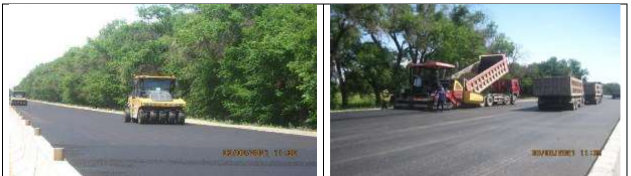
Figure 5 Asphalt laying
