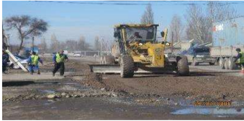
Figure 31 Work in winter 2021
