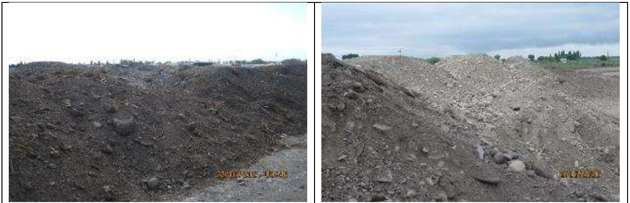
Figure 72 Storage of unsuitable soil for further use
