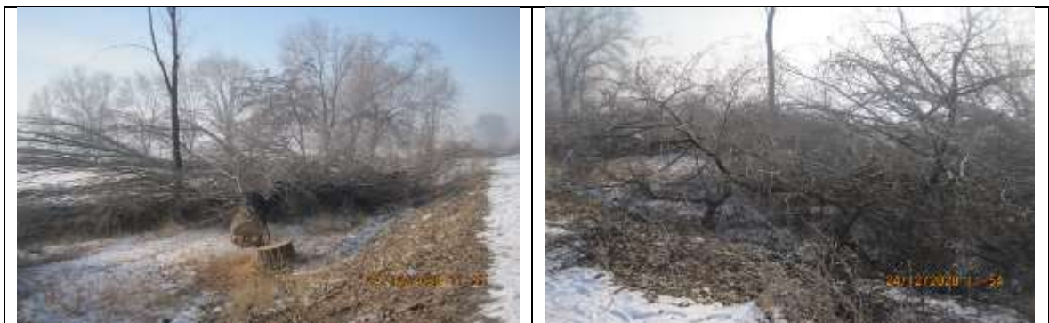
Figure 30 Tree cutting on the road section km 8.5 - 15.9
