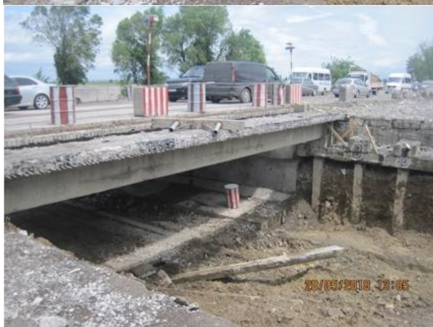
Jelamysh Bridge construction
