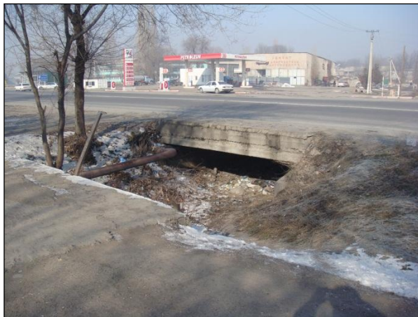
Flood canal in Novo-Pavlovka Village
