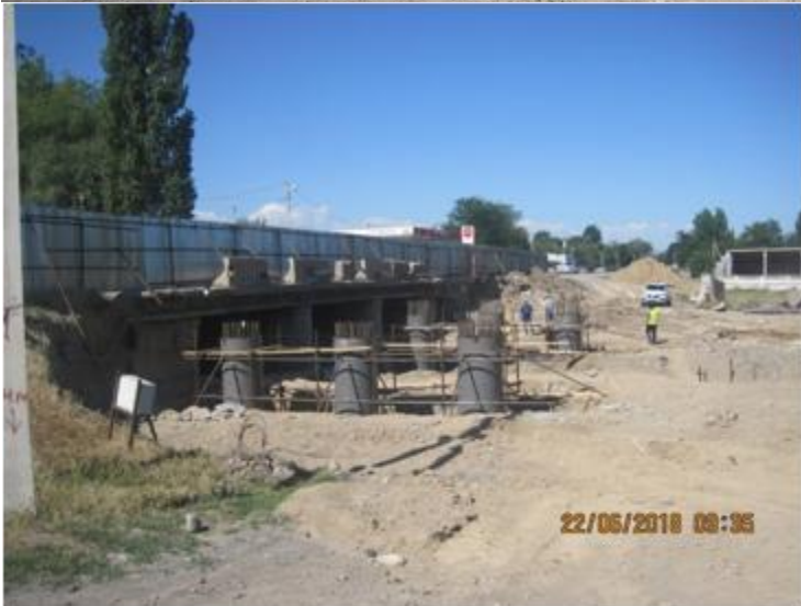
Sokuluk River bridge Construction site, June 2018
