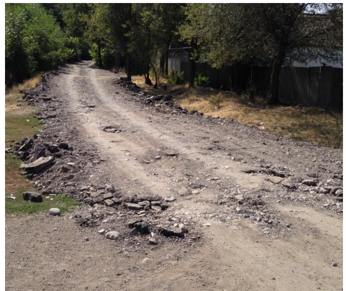
Figure 22. Six examples of waste asphalt and subgrade gravel placed on rural roads by the contractor. Transport placement and grading usually took 6-14 days.
