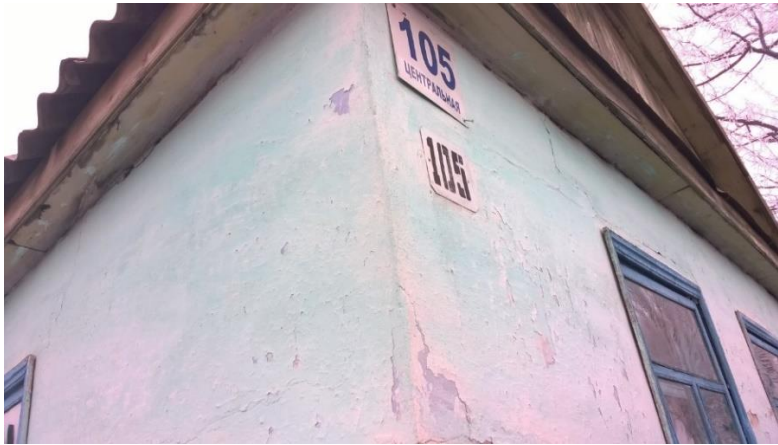
Figure 6. No. 105a Centralnaya Street, Petrovka
