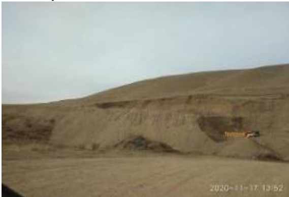
Borrow pit at Km 133+000.
