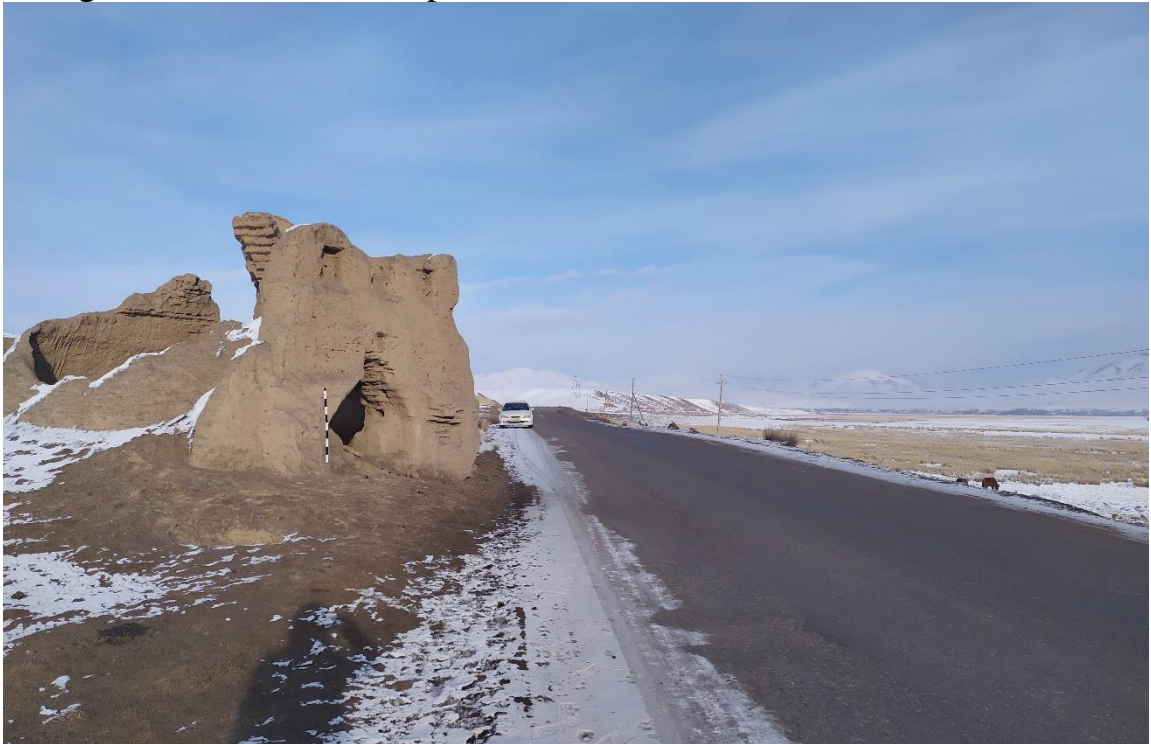
Fig.14. Altyn-Aryk 1. Kumbez next to the shoulder. It is recommended to construct the pavement from the kumbez side without shoulder with barriers along the road and to install a "Stopping Prohibited" sign.
