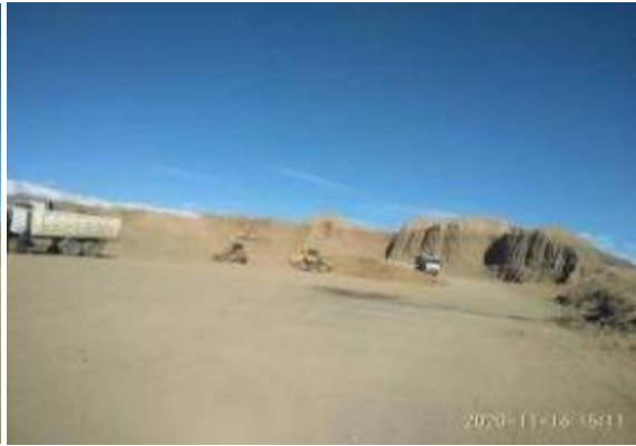
Borrow pit at Km 135+280.
