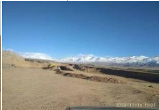
Borrow pit at Km 140+990.
