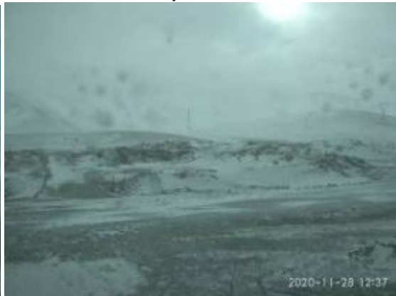
Borrow pit at Km 106+350.
