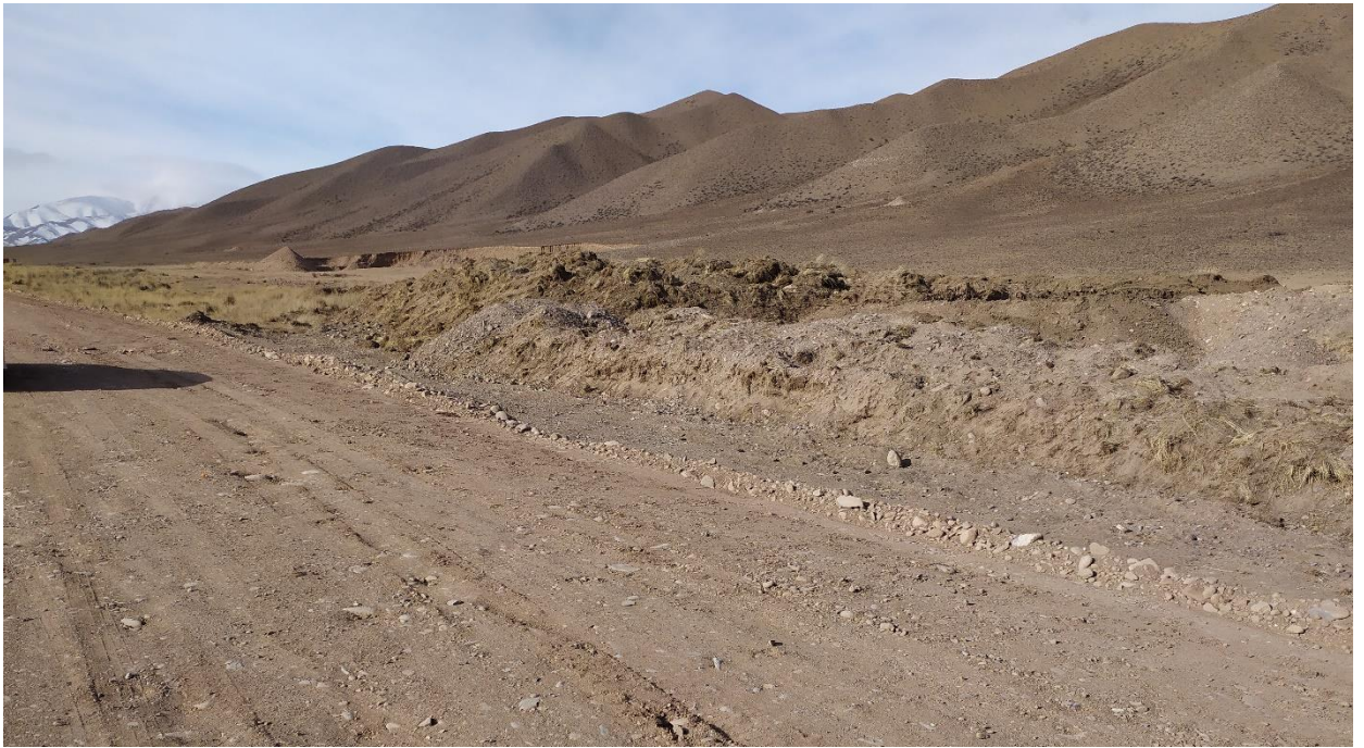
Fig.1. Ak-Chiy 1 Section. Leveled road section.
