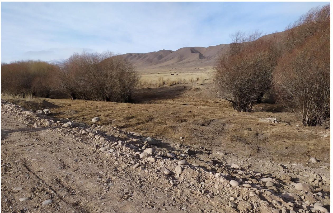
Fig.4. Ak-Chiy 2 and 3 Section. Right-of-way Leveling.
