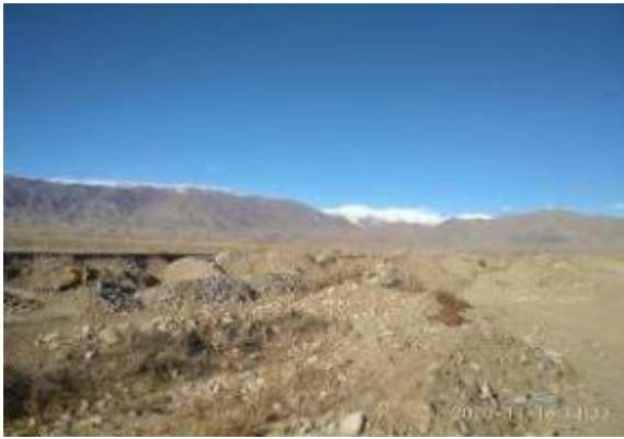
Borrow pit at Km 148+630.
