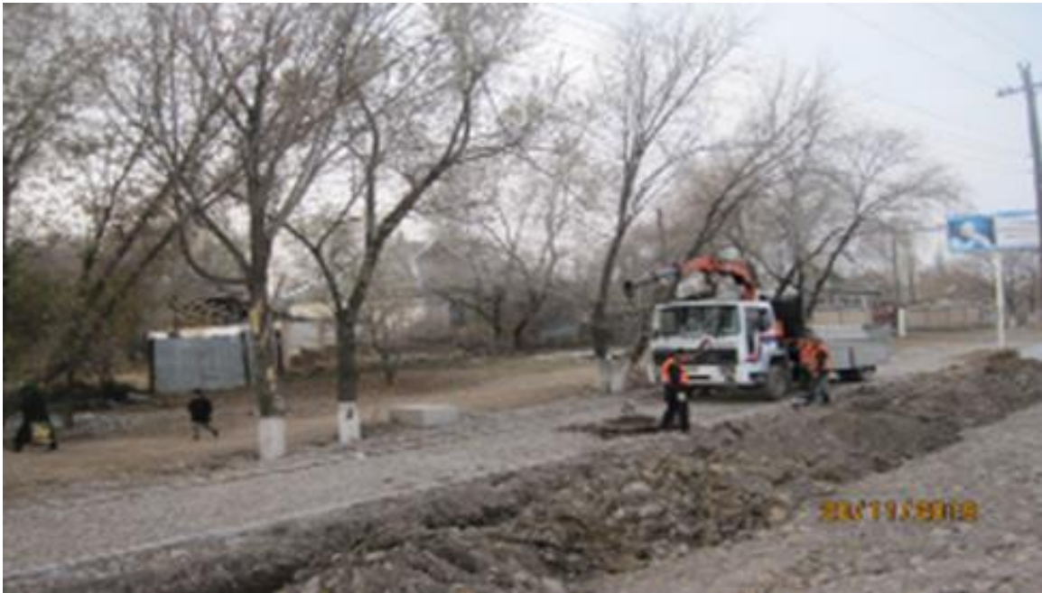
Relocation underground lines and culvert installation
