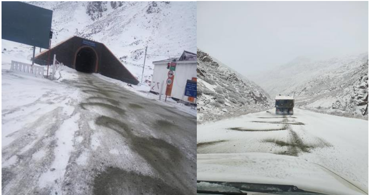
Sand bedding of the road
