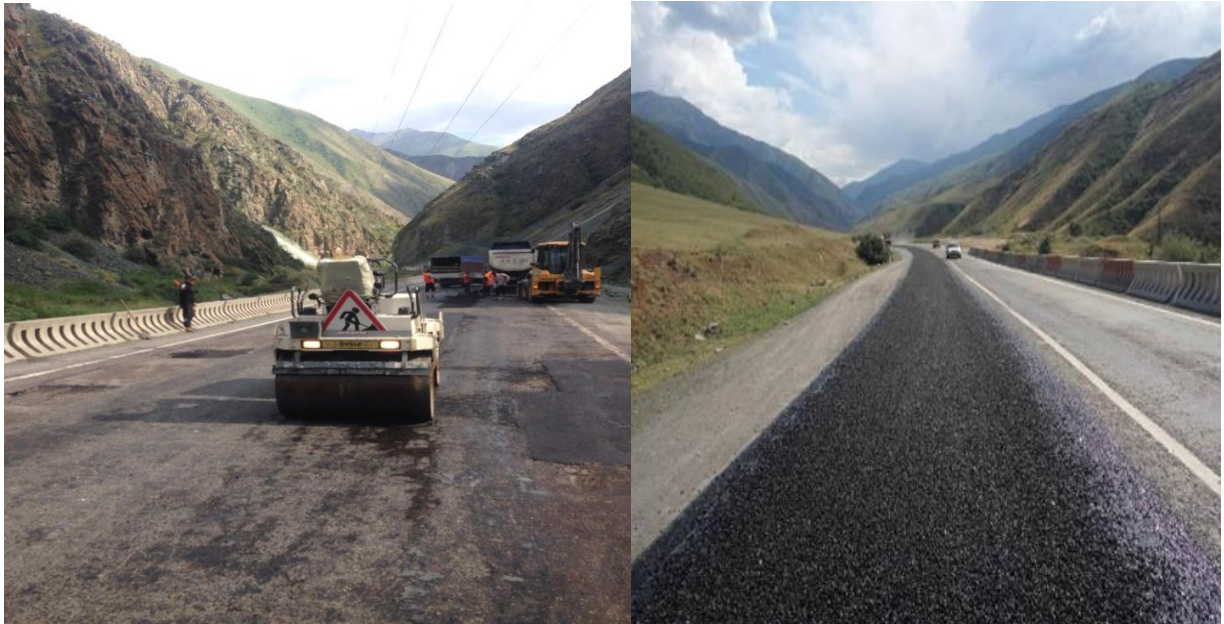
Current repairs of the pavement
