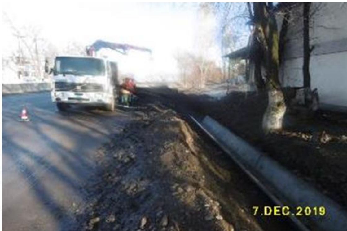
Installation of irrigation ditches
