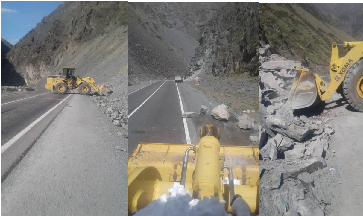
Clearing roads from debris and rock falls
