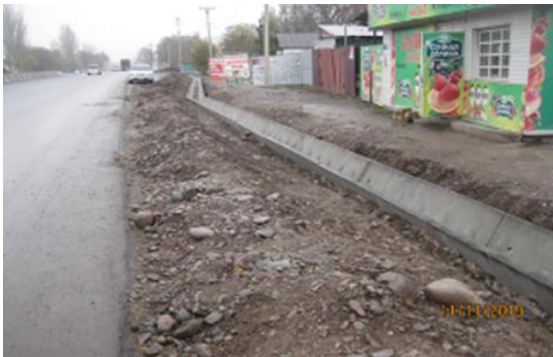
Installation of irrigation ditches
