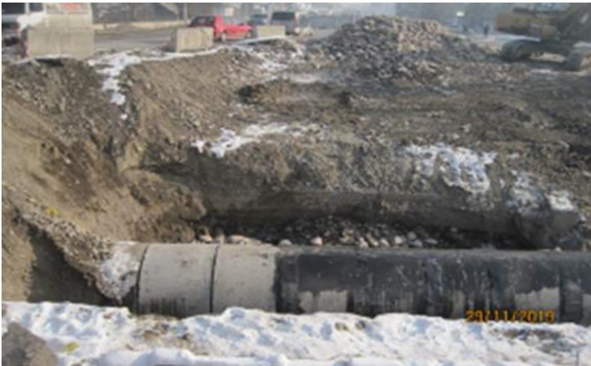
Relocation underground lines and culvert installation
