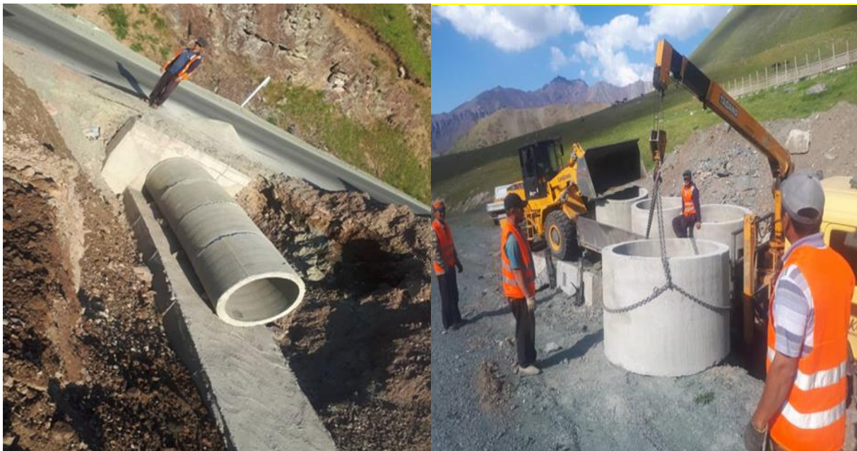
Culvert replacement
