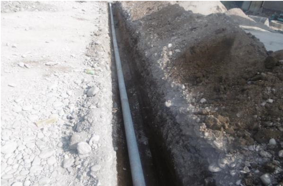
Figure 2-4: Placing the Concrete Tubes for the Underground Communication Cables
